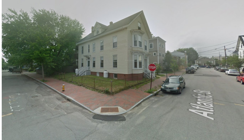
Figure 3: The existing conditions at the project site, from Google Street View.
