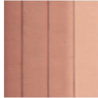
Painted Siding Primary Cladding
