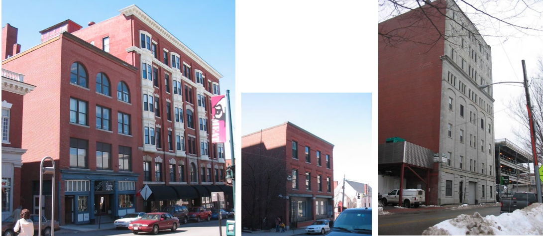
Figure 3: 2006 views of (from left to right) The Potter Building (24 Preble), The Wadsworth (28 Preble), 38 Preble, and The Allen Storage Building (338 Cumberland).
