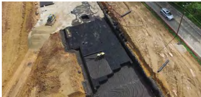
R-TANK SD INSTALLATION
