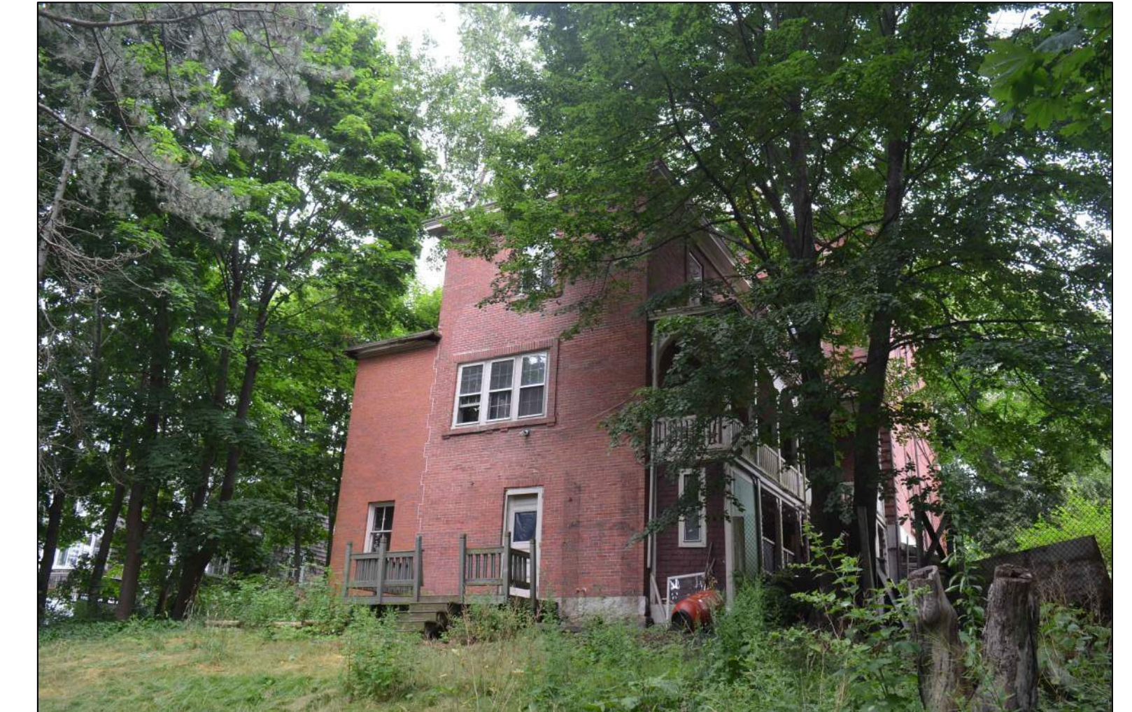
EAST VIEW FROM REAR YARD
