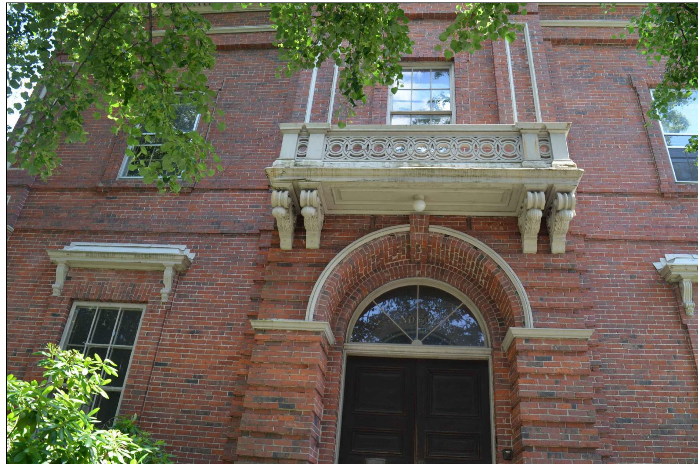
NORTHWEST ELEVATION FROM SIDEWALK
