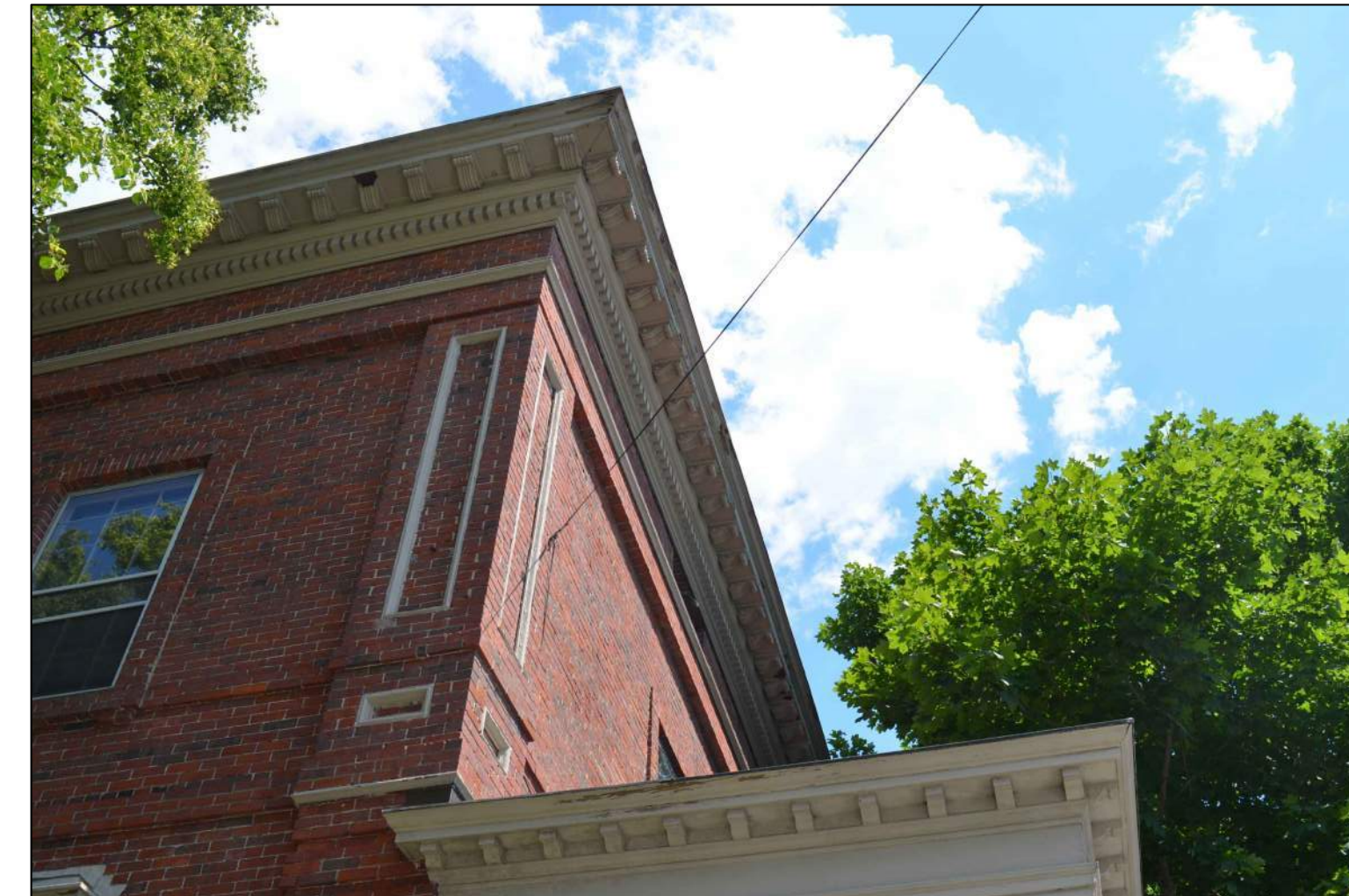
FRIEZE AND SOFFIT DETAIL FROM FRONT YARD
