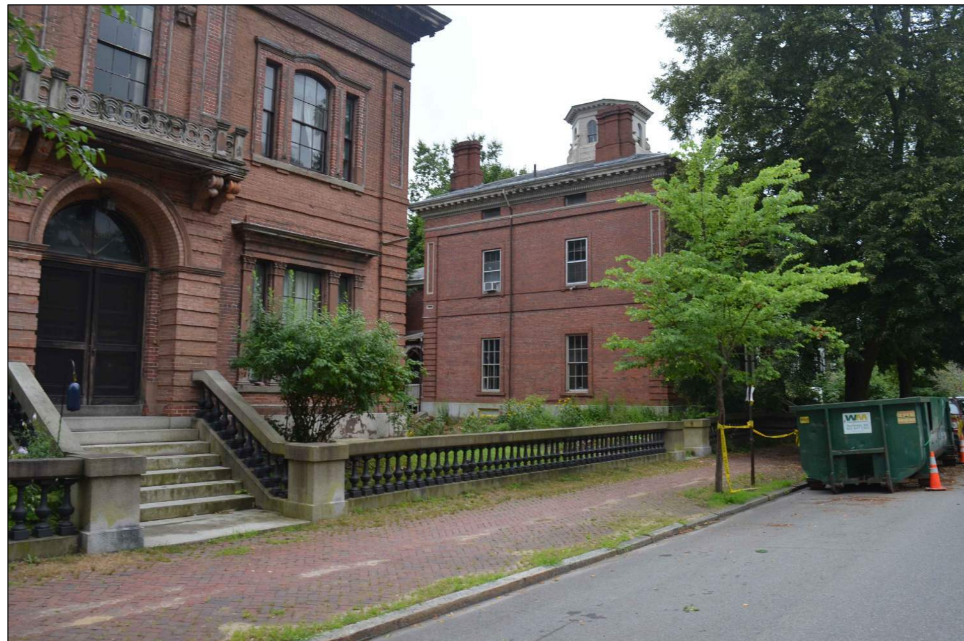
NORTH VIEW FROM DANFORTH ST
