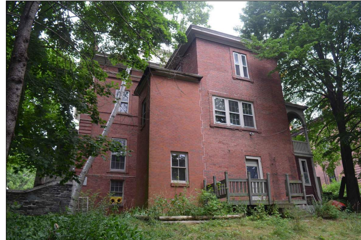
SOUTHEAST VIEW FROM REAR YARD
