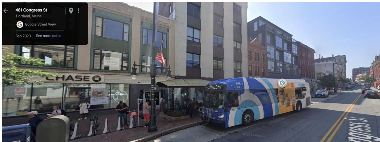
Congress Street Bus Shelter and Bike Share at front of building
