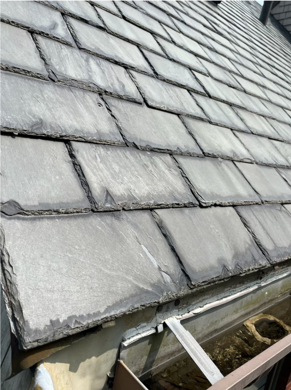
Close up of the roof.
