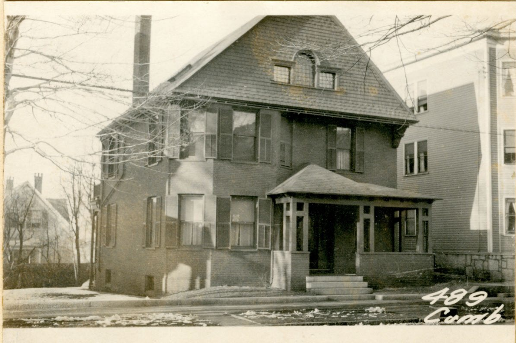
Figure # 3: 1924 Tax Photo of 489 Cumberland Avenue
