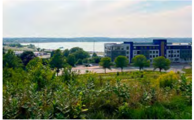
Four-story, 55 H (with rooHop appurtenances) at 218 Washington Avenue
