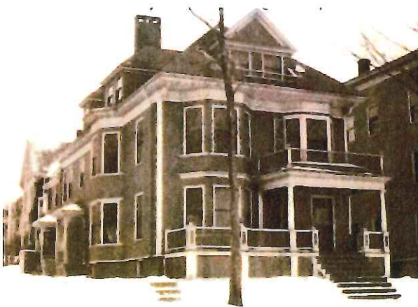
Colonial Revival apartment house at 164 Eastern Promenade.
