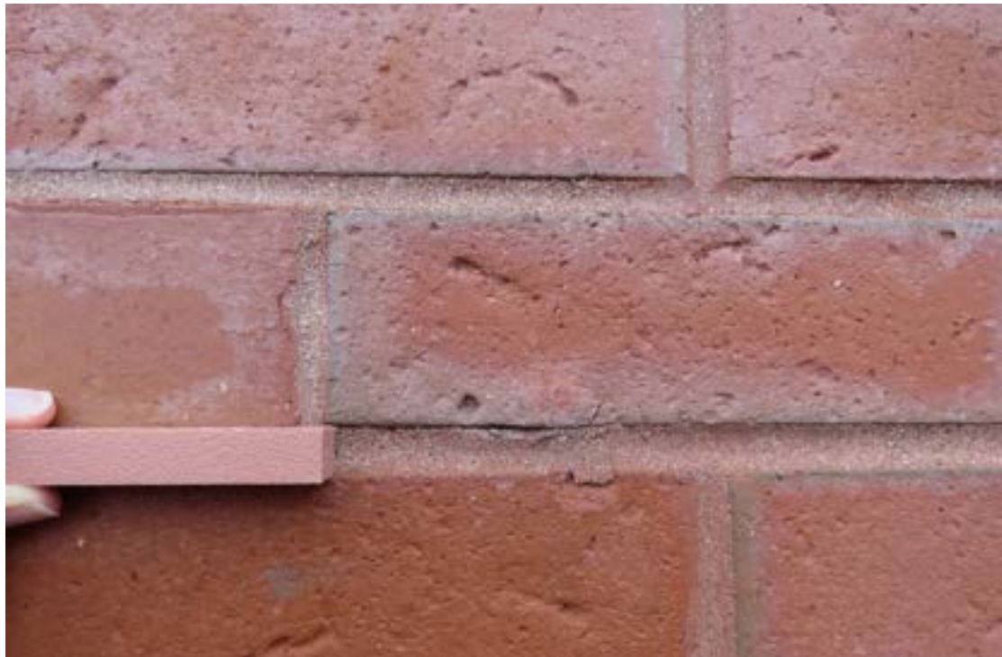
Masonry: Morin Brick Old Port Full Range Blend Red Mortar
