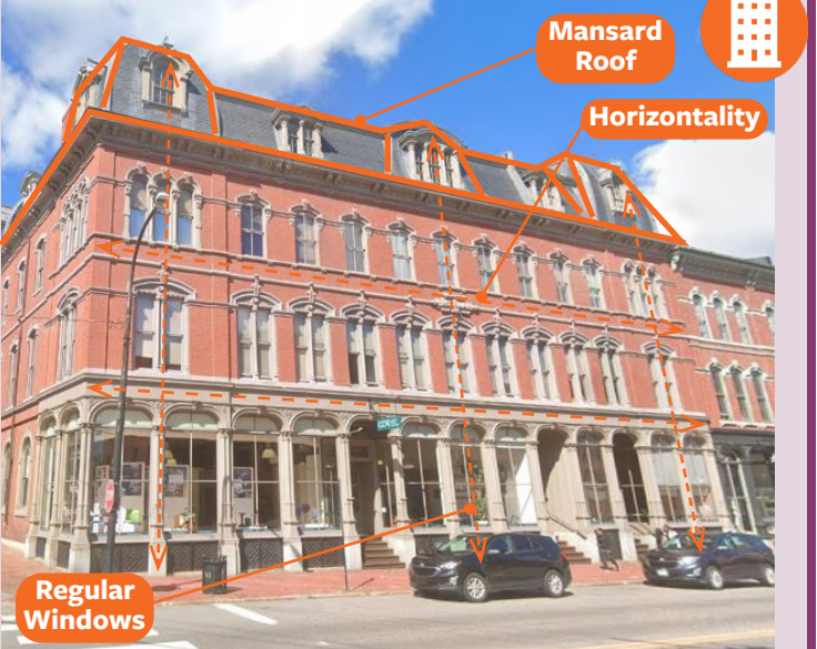
141 Middle St, Woodman Bldg (1867) REDO.jpg
