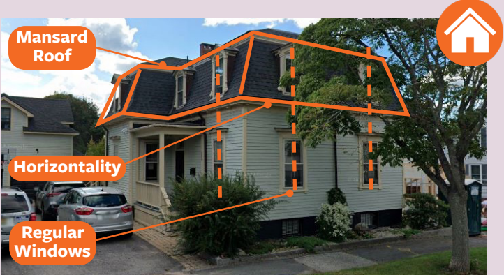
122 North St (1890) REDO.jpg
