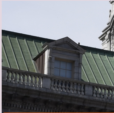
Standing seam copper
