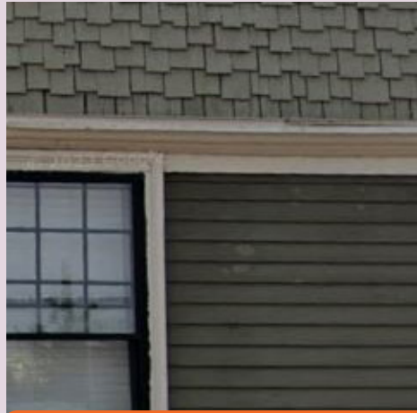
Clapboards and staggered shingles
