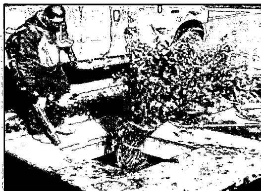
5. Clean area around Filterra
