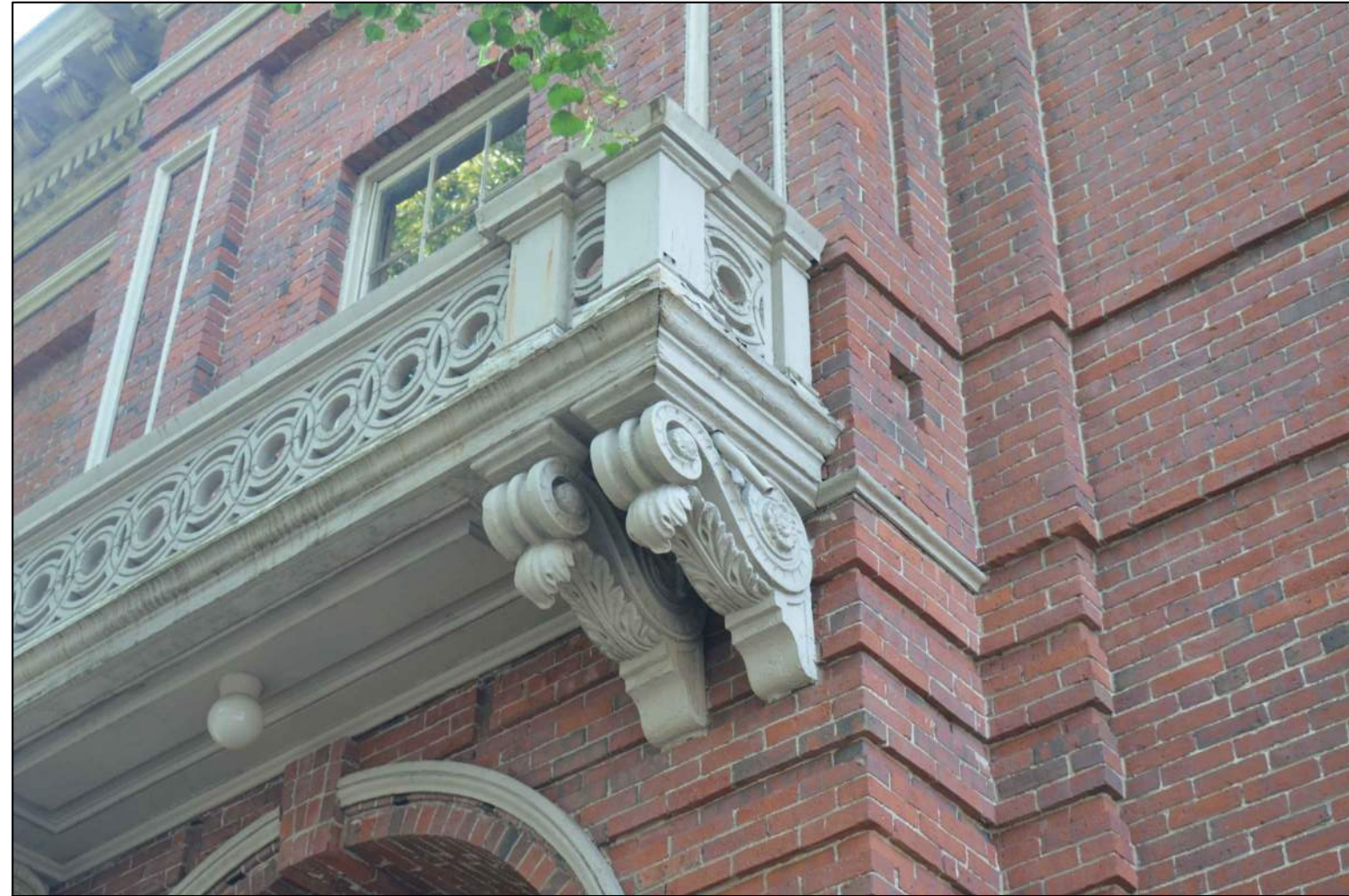
ORNATE DETAIL FROM FRONT YARD
