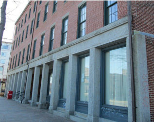
Expressed structural elements, Arcade, Fenestration recessed from building face, Change of materials, Lintels, Cornice
