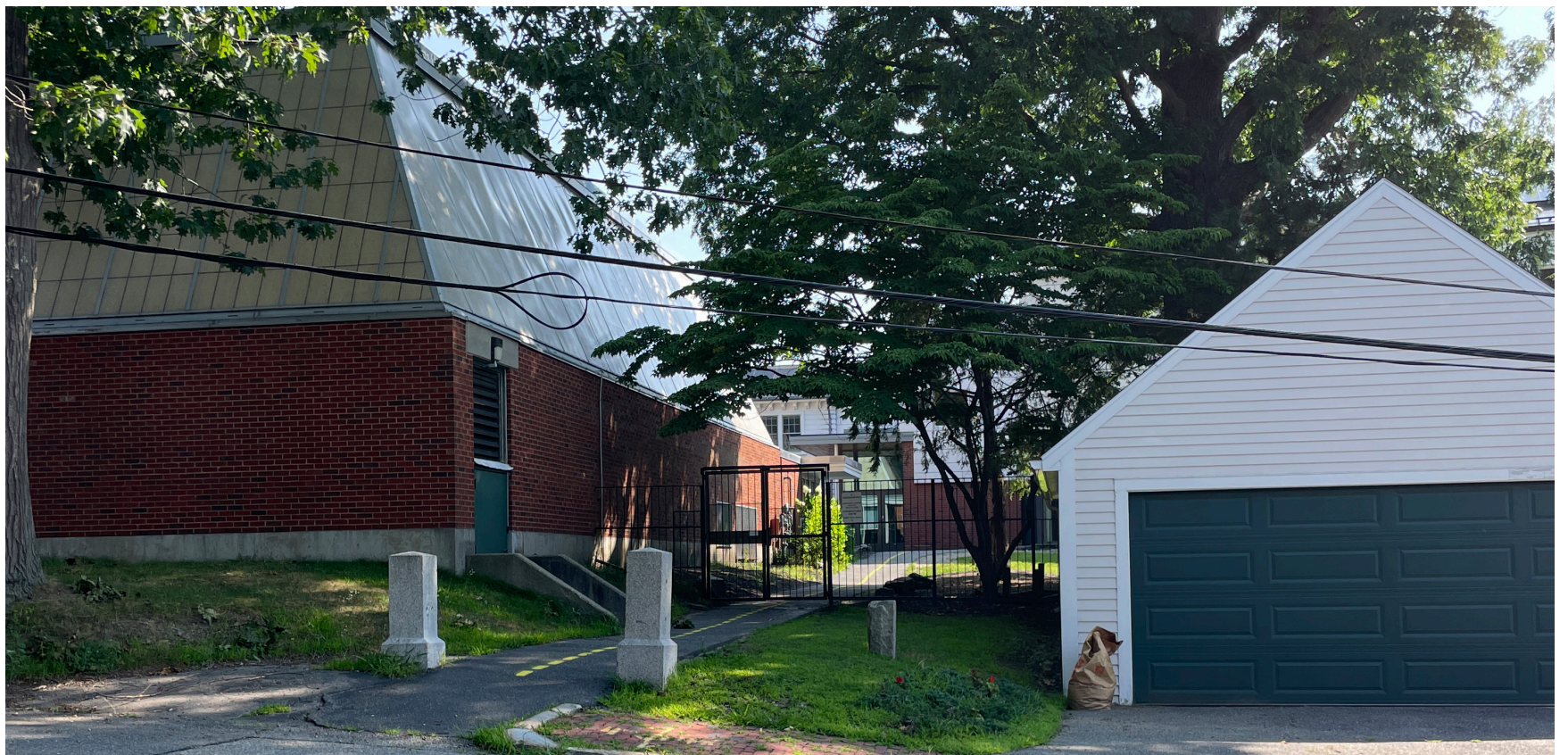
G - Existing Gym - Fletcher Street Campus Entry
