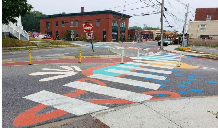
Figure 22: Refuge repainting of painted crosswalk in Woodford corner
