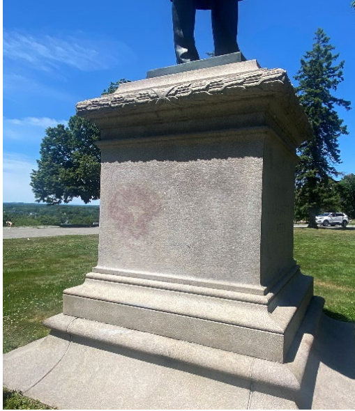
Figure 8: Graffiti removal progress
