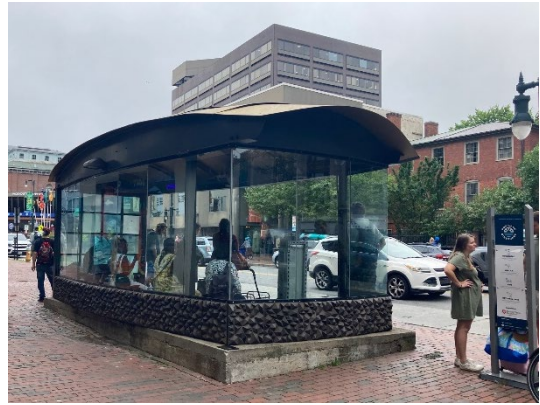
Figure 2: Glass Panels replacement
