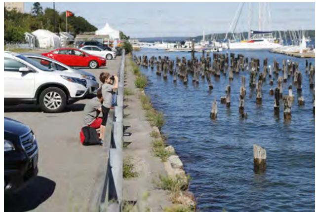
Waterfront view with pilings
