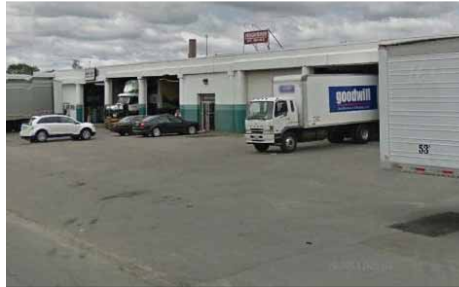
Figure 5-38: Fox Street before driveway improvements
