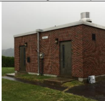
Location 14: Mechanic Street Pump House (South Portland)
