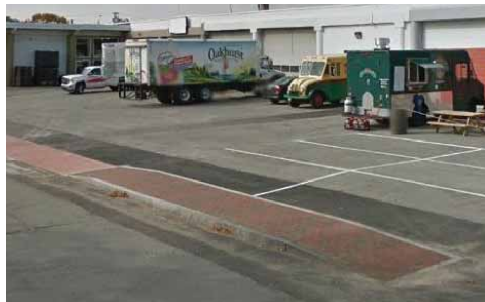
Figure 5-39: Fox Street after driveway improvements
