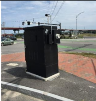
Location 10: Casco Bay Bridge
