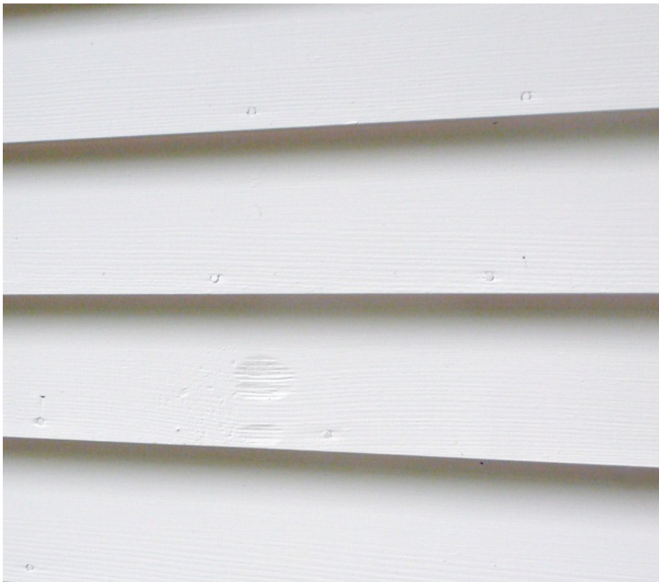
4" reveal painted cedar clapboards with 4.5" corner boards on main structure and dormer. 7.25" fascia boards with 5" soffit.
