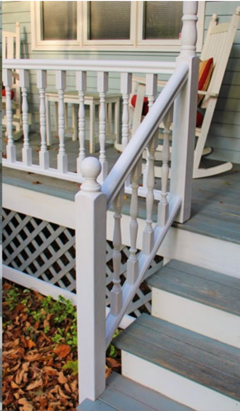
example of porch new porch entrance style. fully trimmed and latticed painted white with clear cedar decking.
