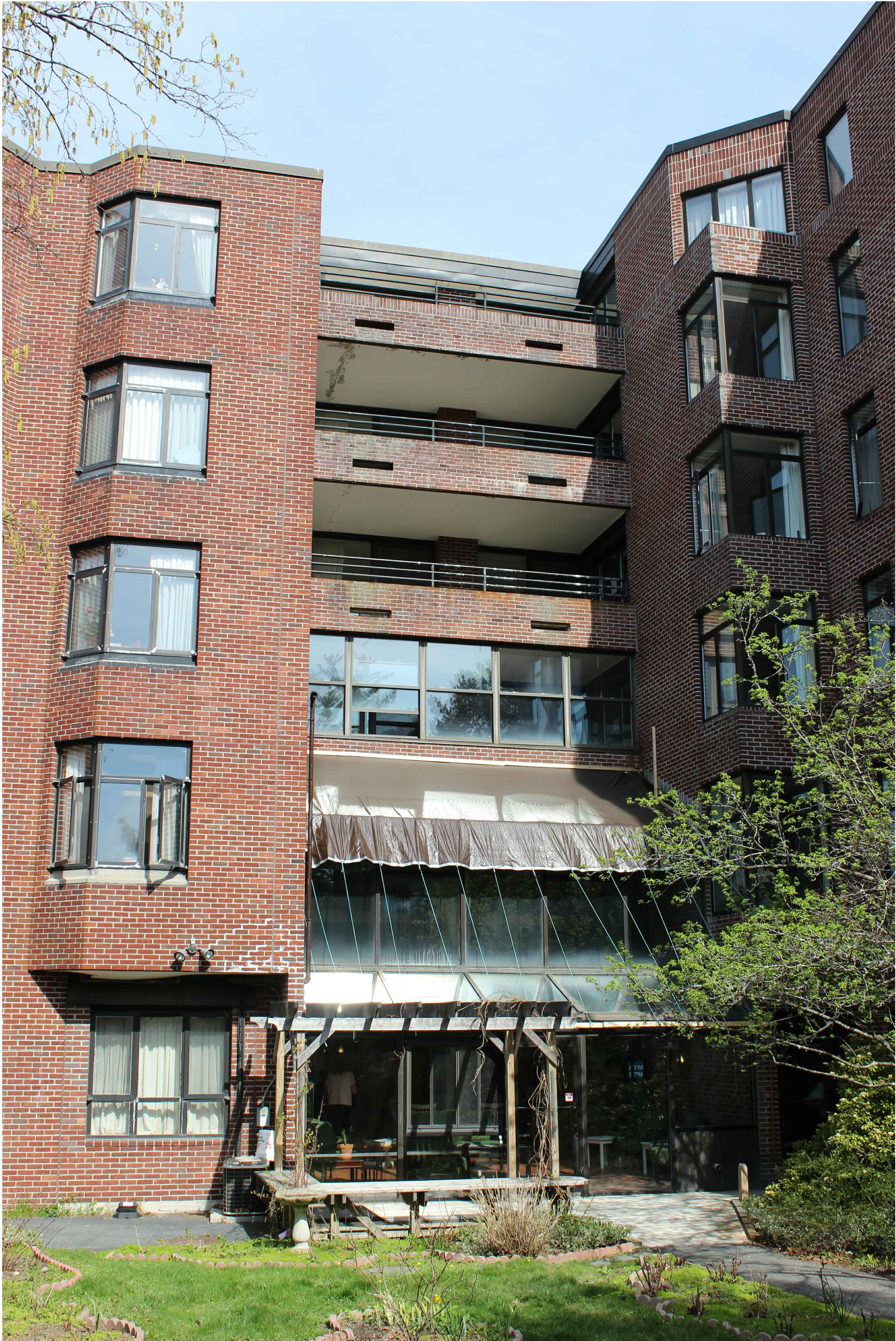
EXISTING GREENHOUSE & PORCHES, VIEW FROM COURTYARD
