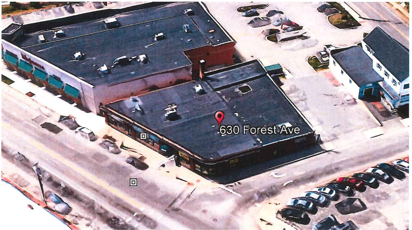
Aerial view showing footprint of later addition
