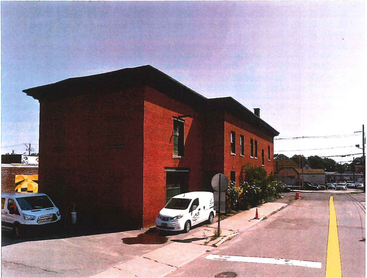
View of building from Revere Street
