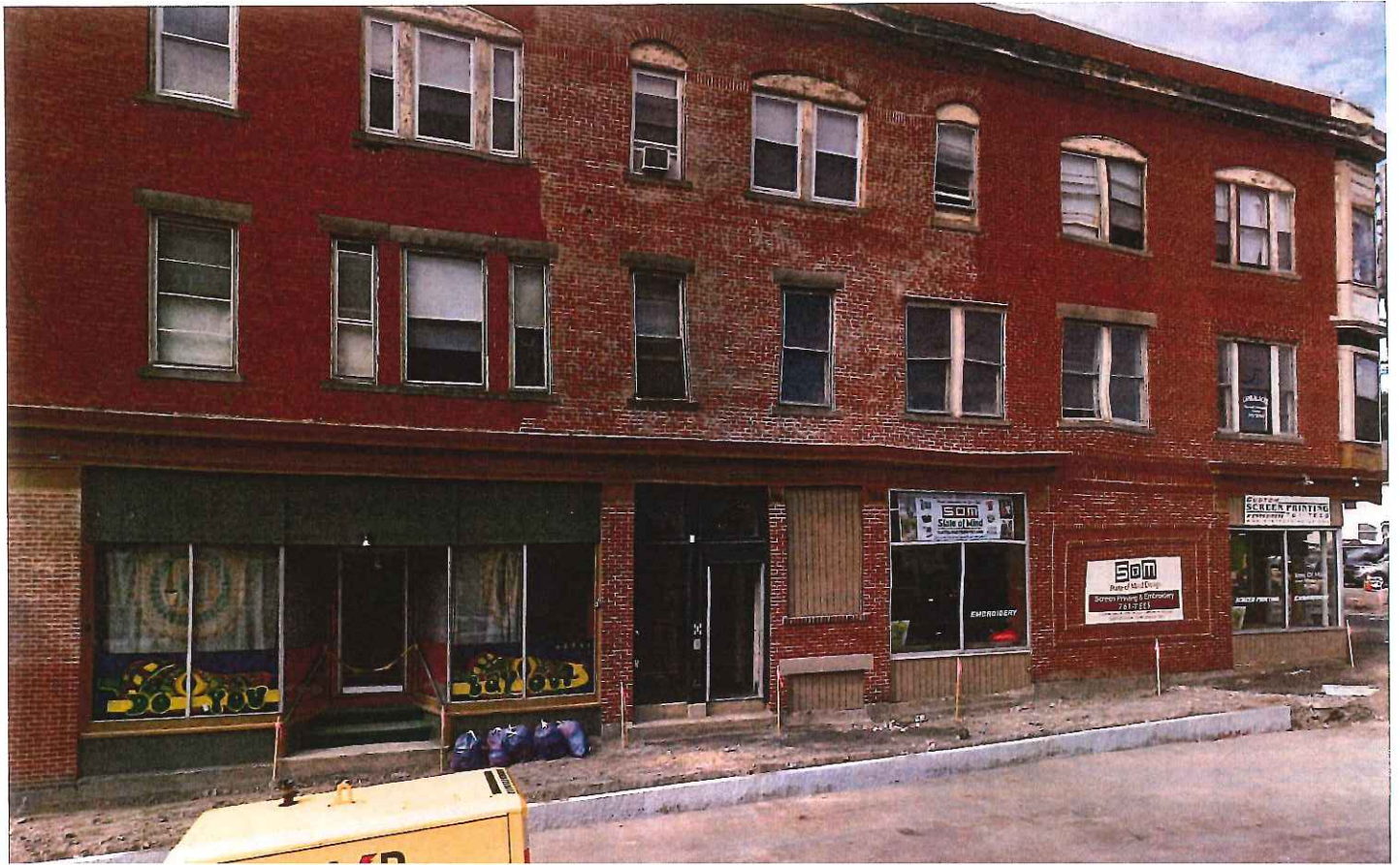
Forest Avenue elevation of Chapman Block
