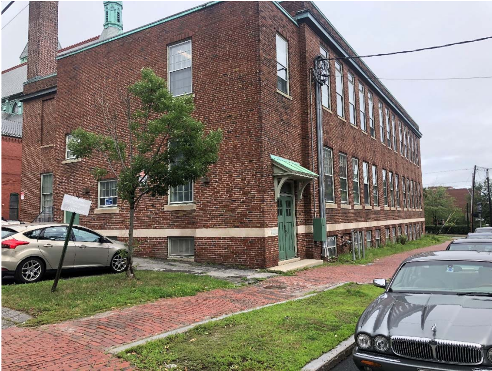
Photo 1 – Existing 66 State Street building taken from Danforth Street looking northeasterly.
