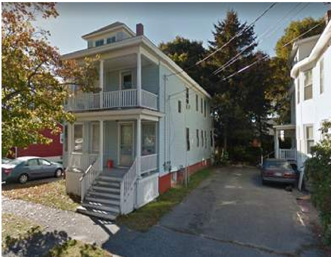
EXAMPLE OF TYPICAL PORCH CONDITION ILLSLEY STREET
