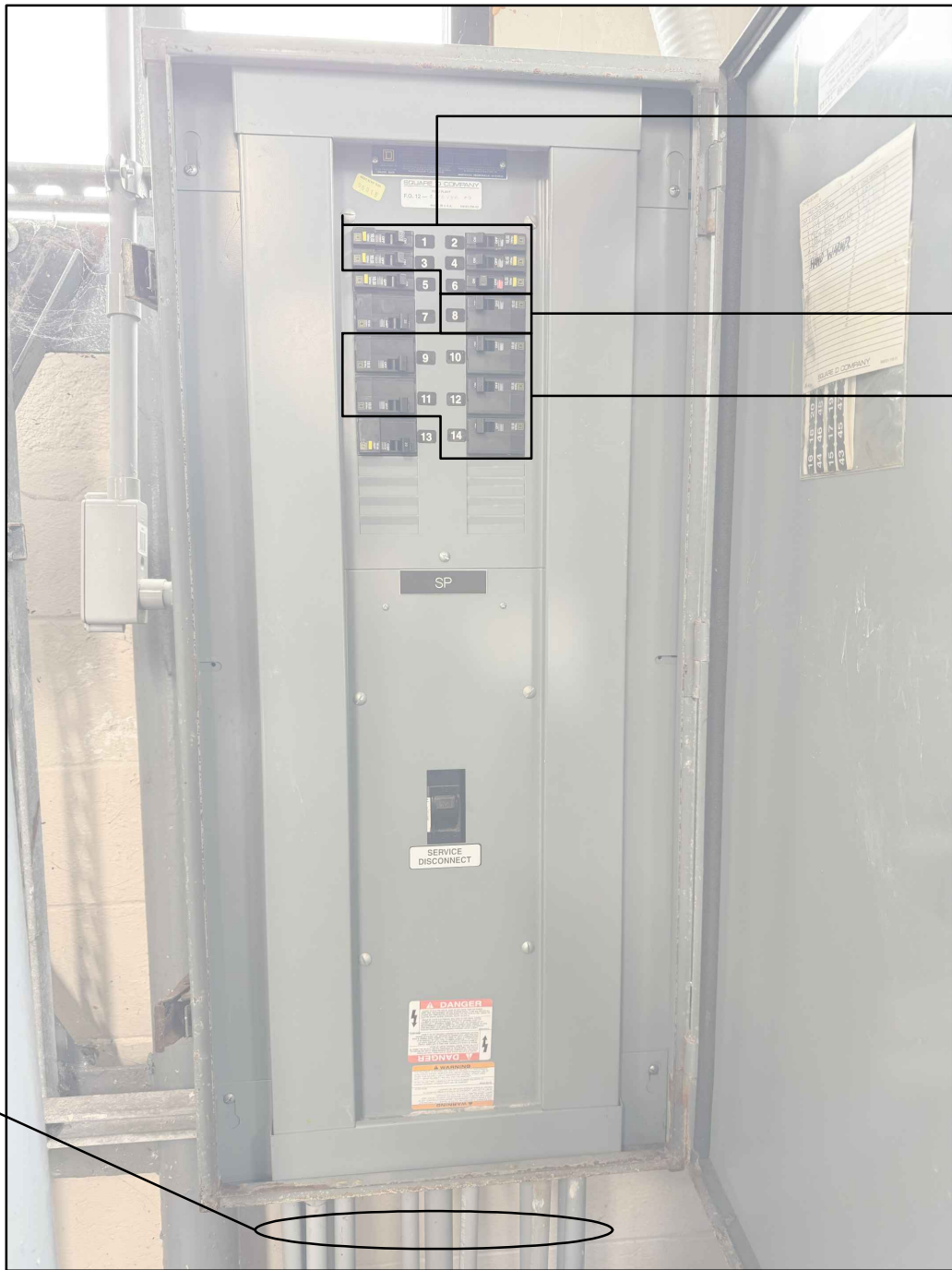
CONDUITS TRANSITION BELOW PIER DECK TO LOADS; SEE SHEET E-001 PHOTOS • (2) 2" - 100A SHORE POWER • (5) 1" - 30A SHORE POWER • (5) 1/2" - 20A GENERAL PURPOSE • (1) 1/2" - POLE LIGHTS • (1) 1/2" - TO BE FIELD DETERMINED
