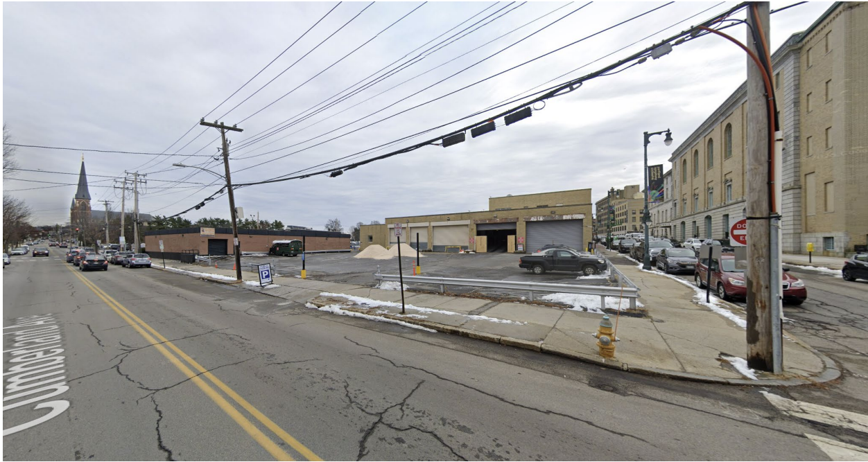
Figure 2. Street view of existing conditions as seen from Cumberland Avenue and Myrtle Street
