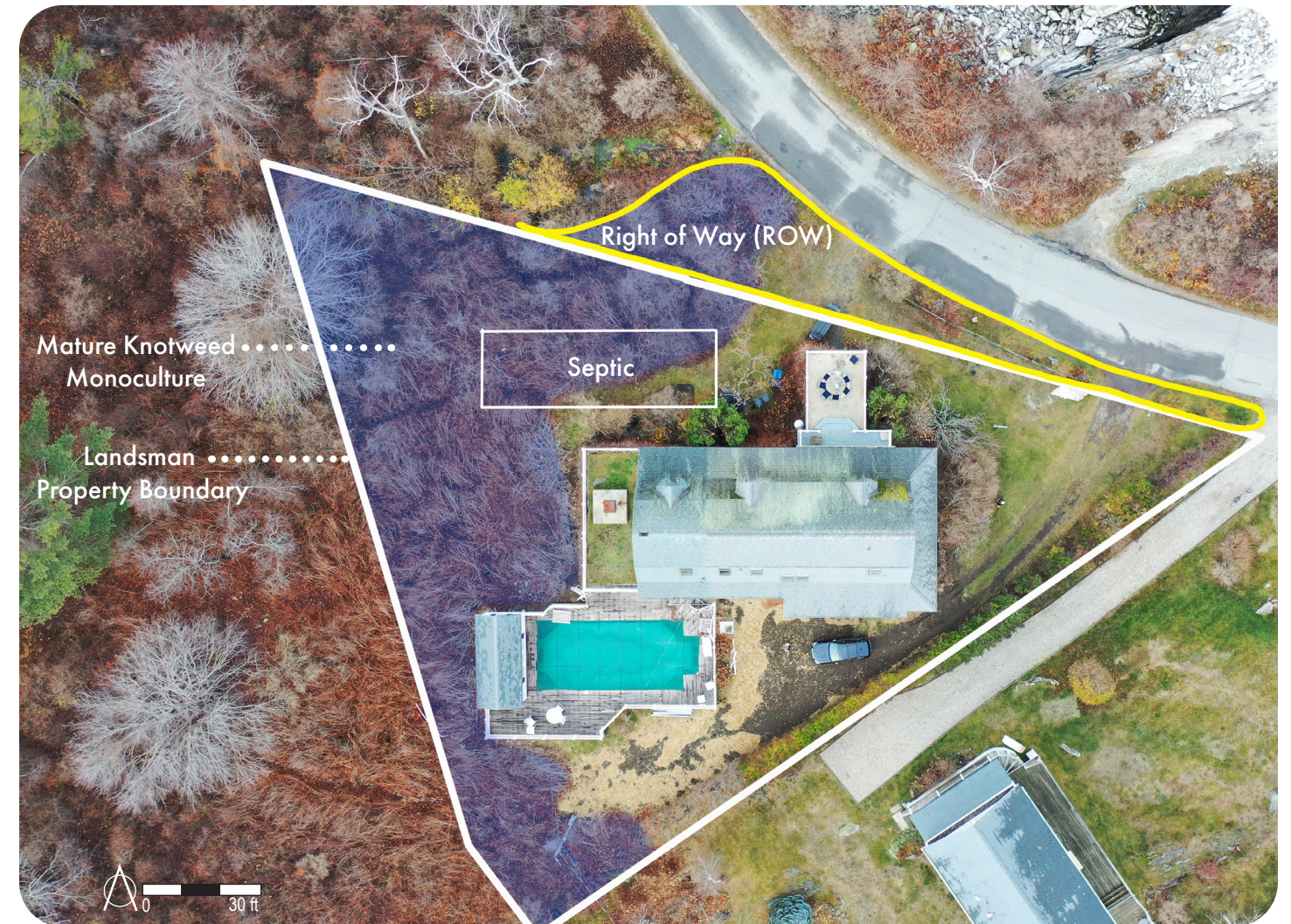
An aerial view of the Landsman property shows the bright orange vegetation of a mature Knotweed monoculture encroaching from the West. The area of Knotweed that this plan proposes for invasive management and removal is highlighted in blue.
