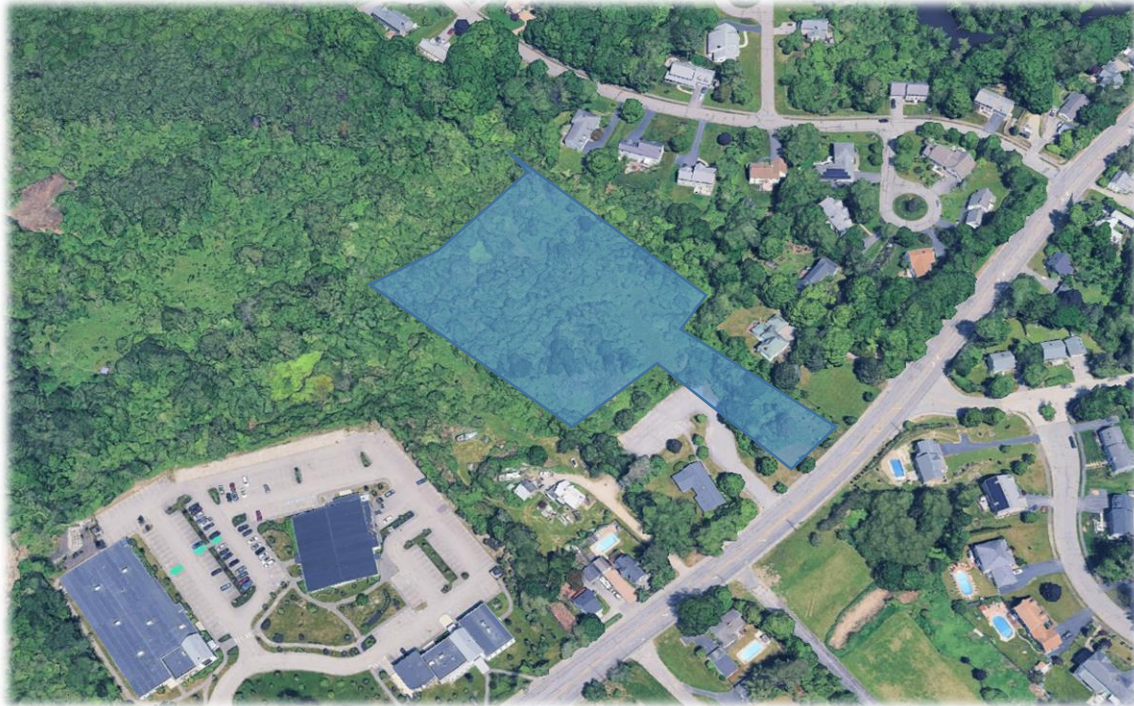
Figure 2: The existing site and surrounding neighborhood
