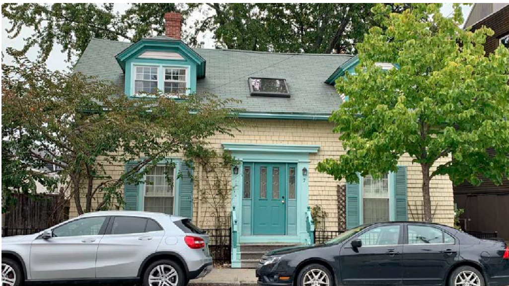
Figure 4: An example of an early, though somewhat altered, cape type house, which would have been common in the early- to mid-nineteenth century (7 Lafayette Street).
