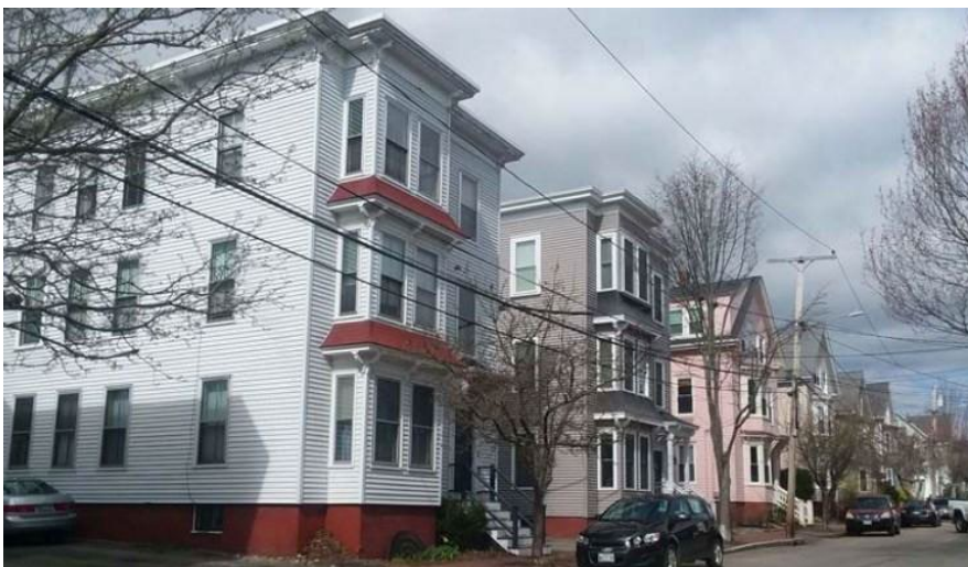
Figure 6: A typical street of triple-deckers and Italianate duplexes (82, 84, 86, & 88 Beckett).
