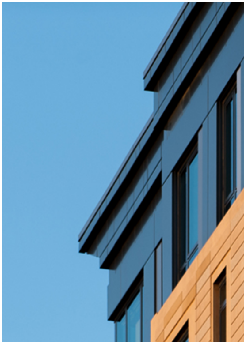
METAL PANEL CLADDING CORNICE
