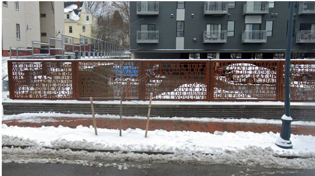
Figure A: Precedent image to screen transformer adjacent to public sidewalk. Image courtesy of Google Maps
