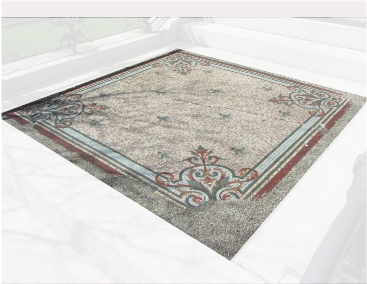
At the Elizabeth M. McDonald House (1882, 161 Pine Street) the front steps include a detailed and colored mosaic landing. A very uncommon exterior feature in Portland’s historic residential neighborhoods, the mosaic was carefully preserved while repairs were made to the surrounding granite entrance stairs.
