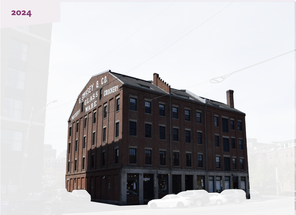
The Swasey Pottery Building (269 Commercial Street) was converted from a warehouse to a mixed use building with retail at the first floor and residential condominiums above. This rehabilitation was completed with minimal exterior alterations
