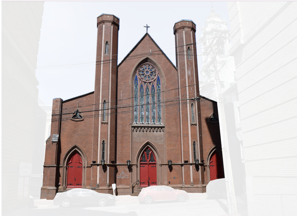
The former Chestnut Street Methodist Church (15 Chestnut Street) has had a number of different uses since it was sold by its parish in the early 2000s, including as a restaurant and an event space. In both of these instances, the rehabilitation took advantage of the large open space of the interior, requiring little to no alterations to significant exterior features such as the ornate stained-glass windows or monumental doors.
