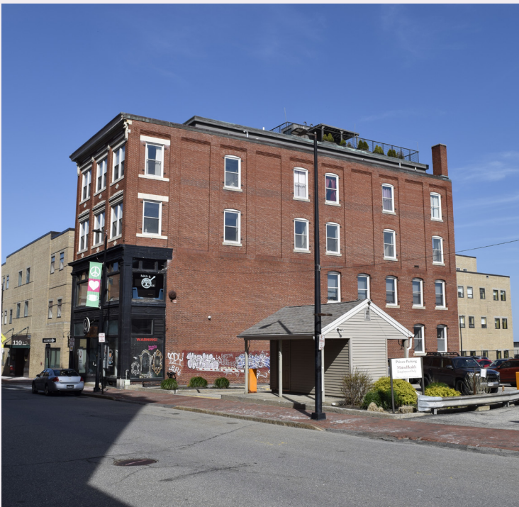
At the Frye Building (1912, 44 Oak Street) an entire floor was added atop the building. In this case, the addition was pulled back from the three sides of the building. Despite its size, because the structure was sensitively placed and clad in recessive materials, it is minimally visible.
