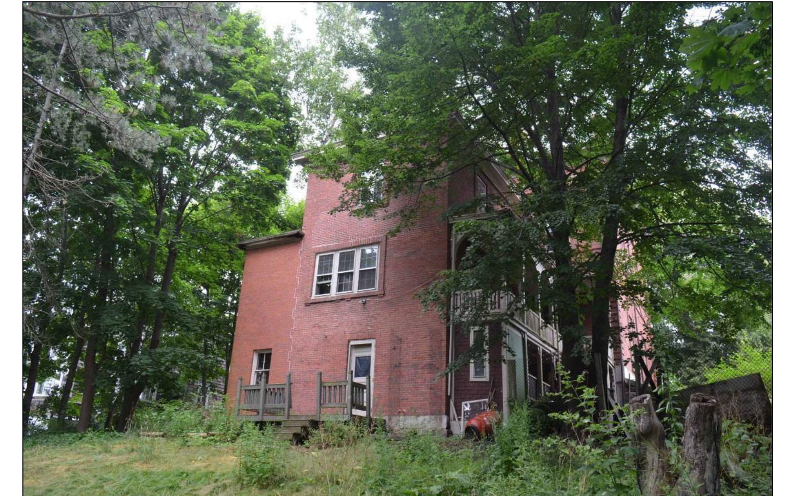
EAST VIEW FROM REAR YARD
