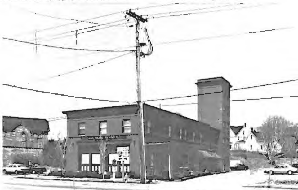
The conversion of the 295 Park Avenue Fire Station to medical offices was done in such a way that necessitated only minimal exterior alterations. The station's form and key features now, as before, communicate its early use. The original doors and hose towers were retained and a new entrance was created on a secondary facade.
