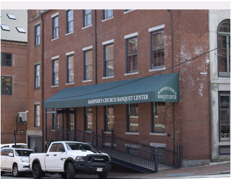
At the Mariner’s Church (1828, 366 Fore Street) a new accessible means of entering the building was required. A new metal ramp was designed to be installed along the side elevation. The ramp was built with its own structure system, minimizing the points of connection to the historic structure. The ramp could easily be removed should a better accessibility solution be developed.
