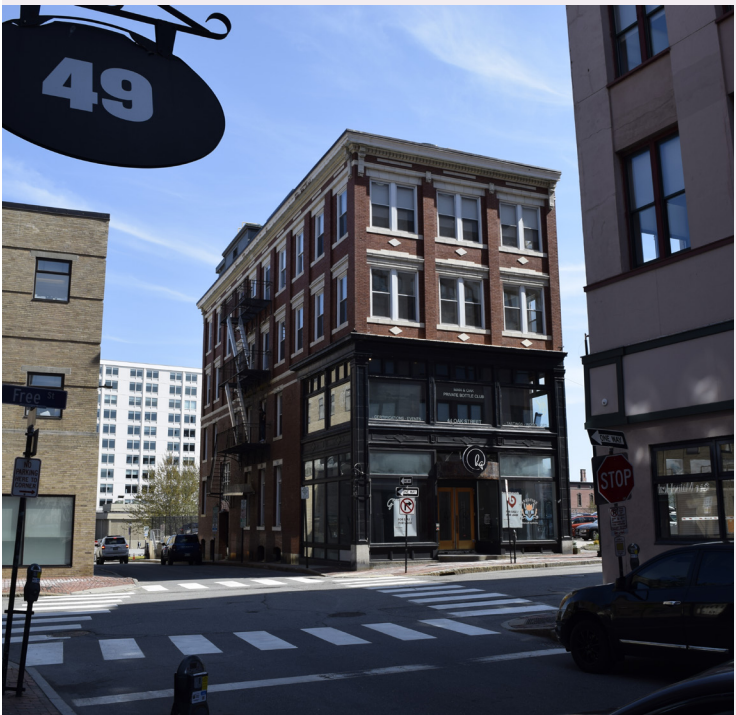
At the Frye Building (1912, 44 Oak Street) an entire floor was added atop the building. In this case, the addition was pulled back from the three sides of the building. Despite its size, because the structure was sensitively placed and clad in recessive materials, it is minimally visible.
