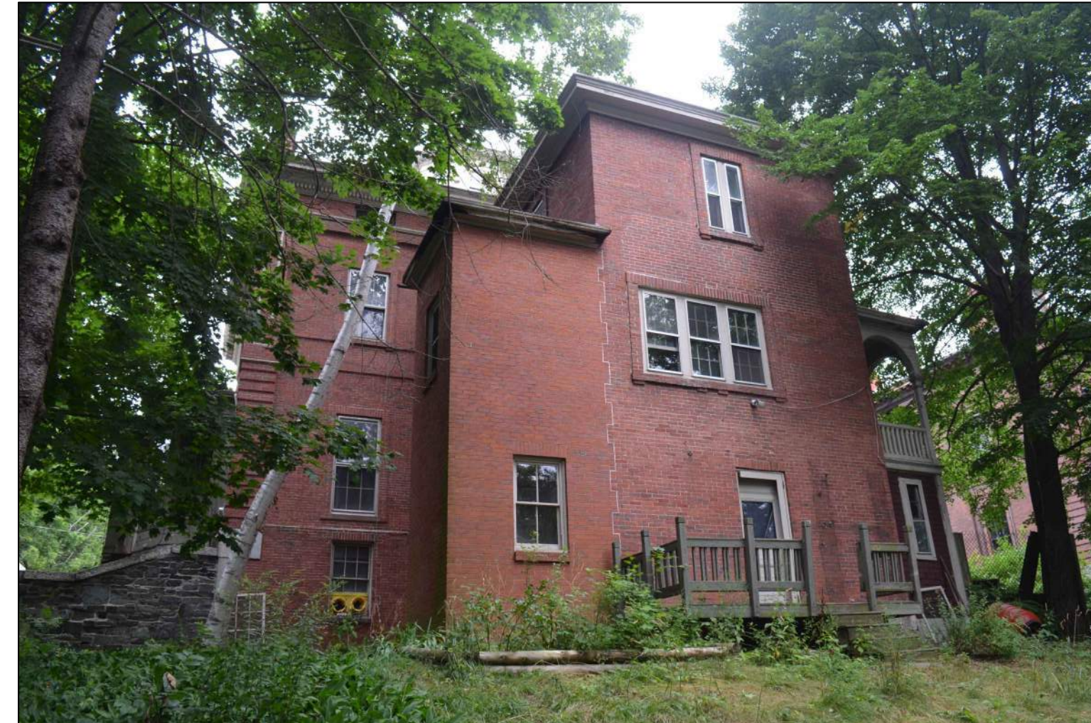
SOUTHEAST VIEW FROM REAR YARD
