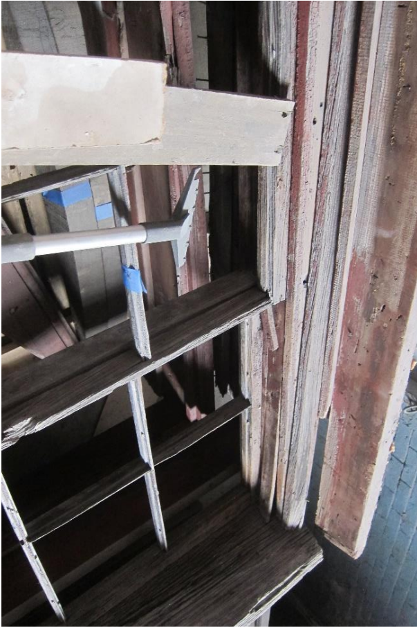
Sixteen-pane double-hung sliding sash exterior with wooden sill
