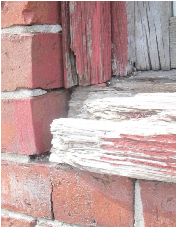
Brick mold and wood sill detail at window opening with brick return exposure. Red paint.
