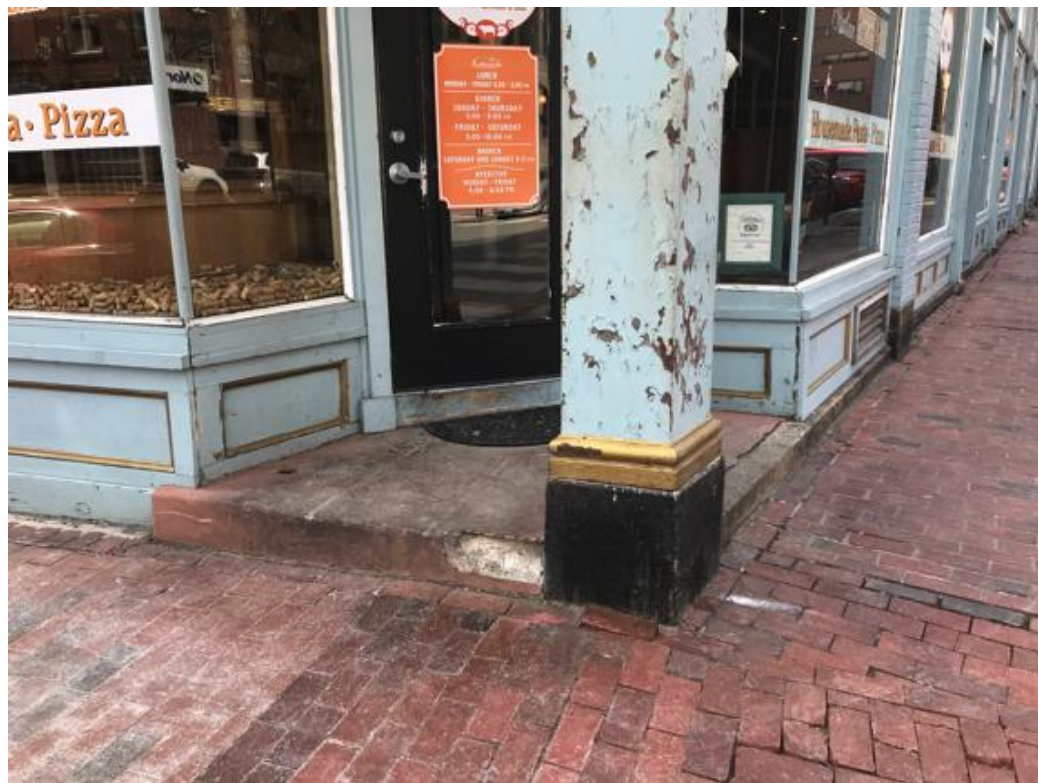
EXISTING RESTAURANT ENTRY
