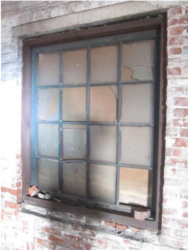
Sixteen-pane fixed sash in original brick opening with non-operable frame.
