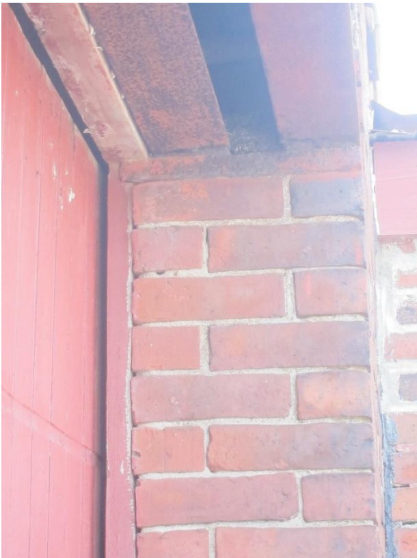
Brick return at large door opening on east façade. Triple wythe under steel channels. No external door.
