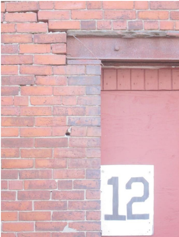
Steel lintel at large door opening on east elevation. Channel is less than three courses deep. Note steel seat and return bricks on alternate courses.
