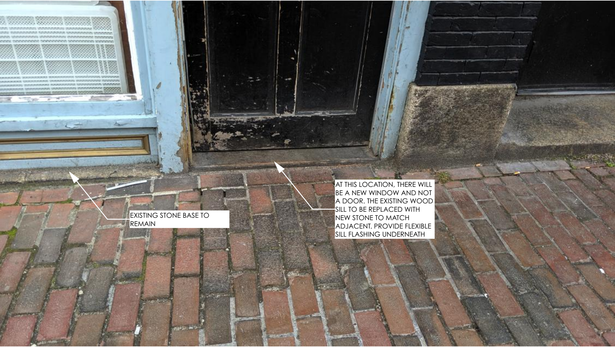
3 At Exterior Former Door Sill at New Window
