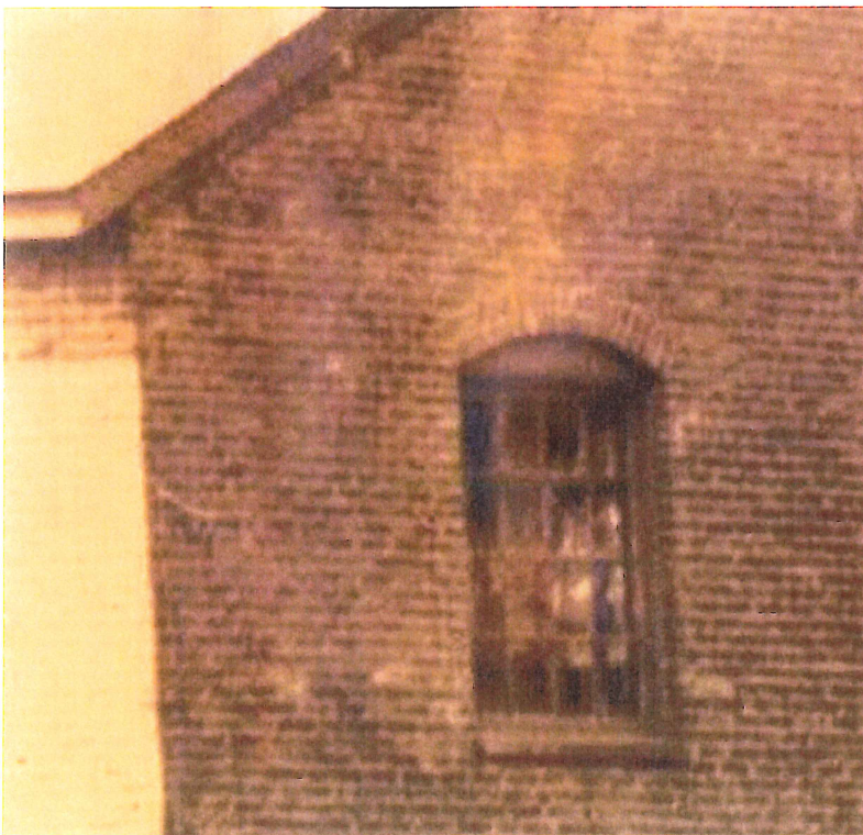
Building #12 – Roof Edge and Window Construction - Excerpted from source image above
