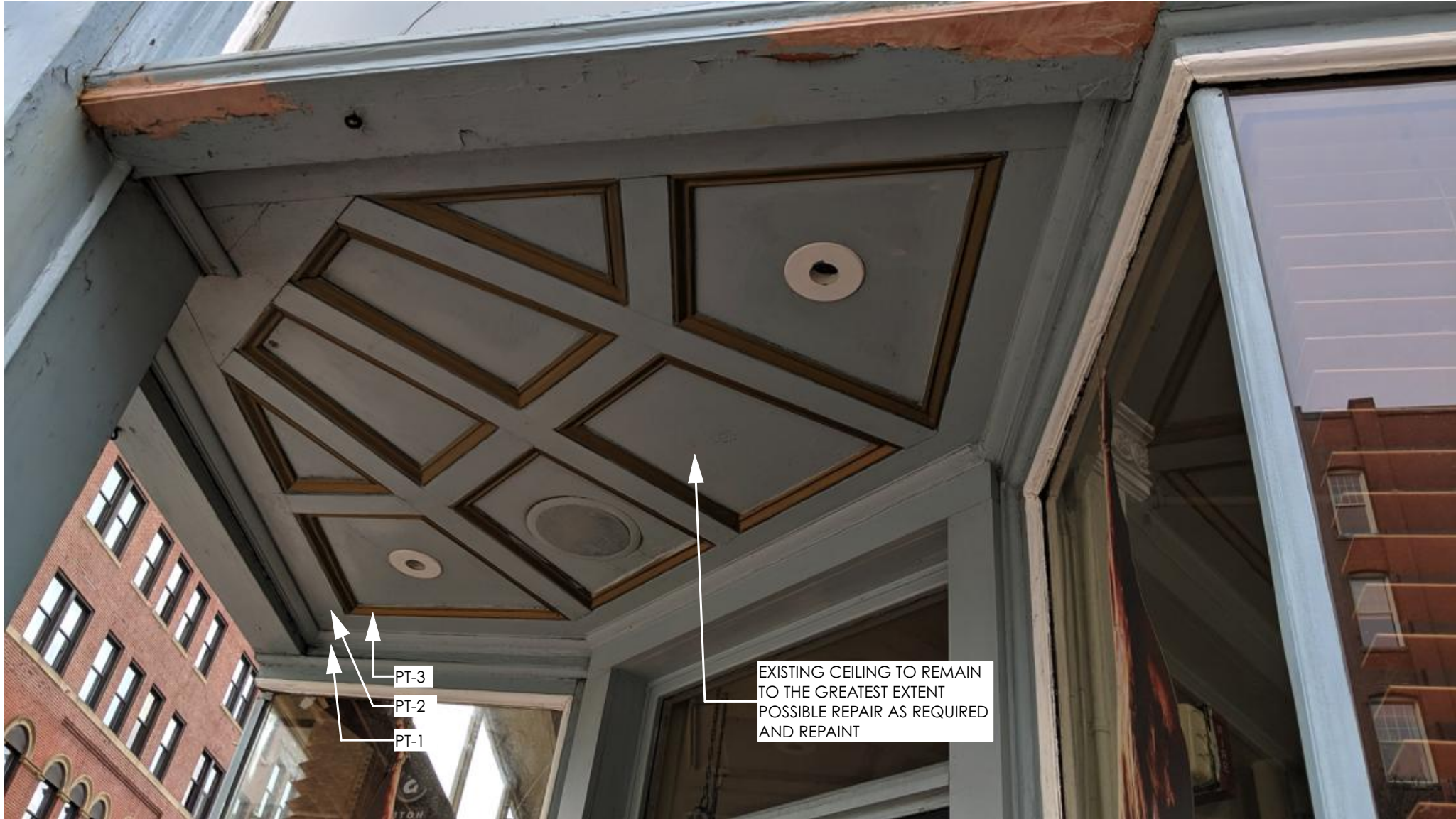
4 At Exterior Ceiling
