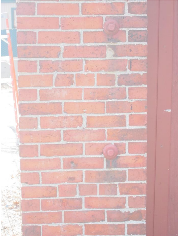
Southeast corner brick at large door opening. Three stretcher bricks. Header bond seven courses apart.
