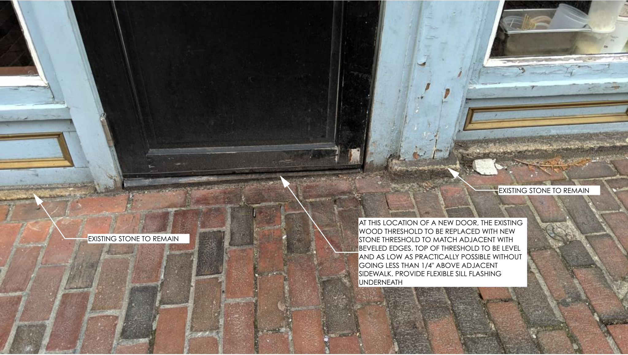
2 At Exterior Door Sill at New Door
