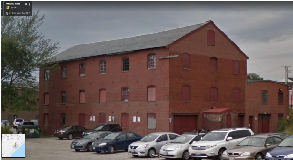
South and east elevations prior to demolition of Building 11 showing window pattern, large door openings at first floor with later vestibule at central door in wall of Building 12. Dark gray slate roof.
