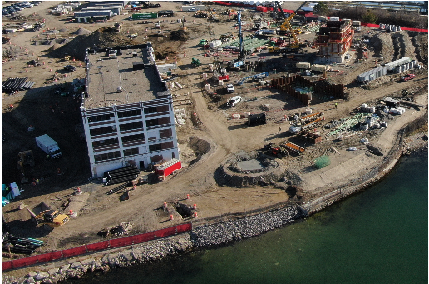
Area of former pier, after demolition, with stabilized shoreline.
