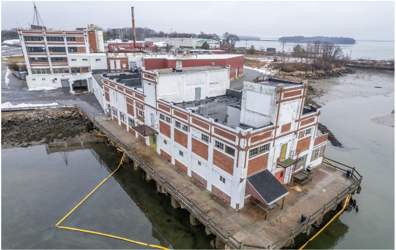
Former pier and Codfish Building
