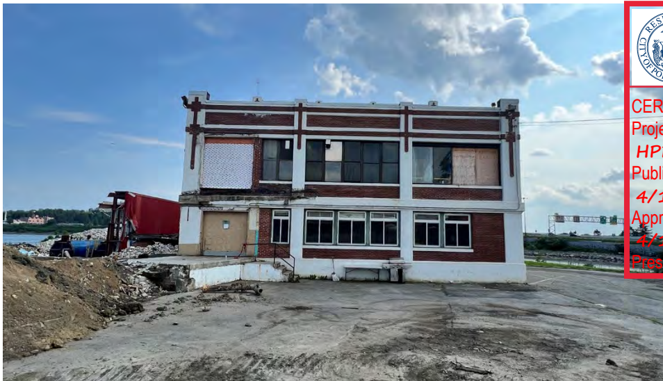
Existing conditions- north façade
