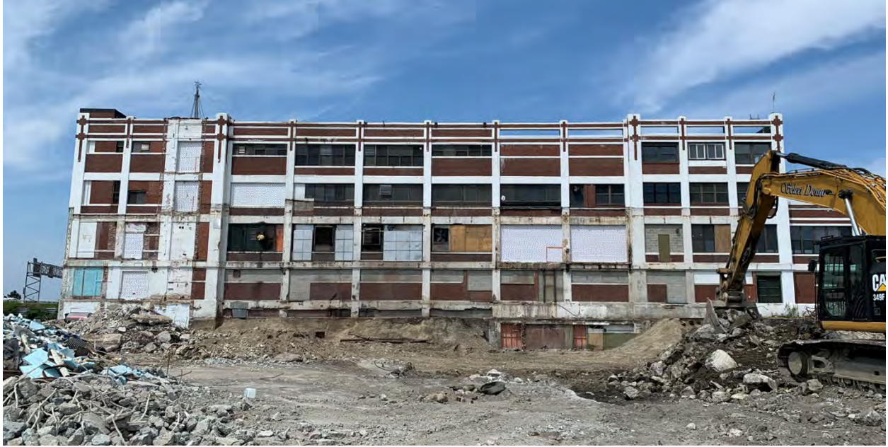
Existing conditions- east façade
