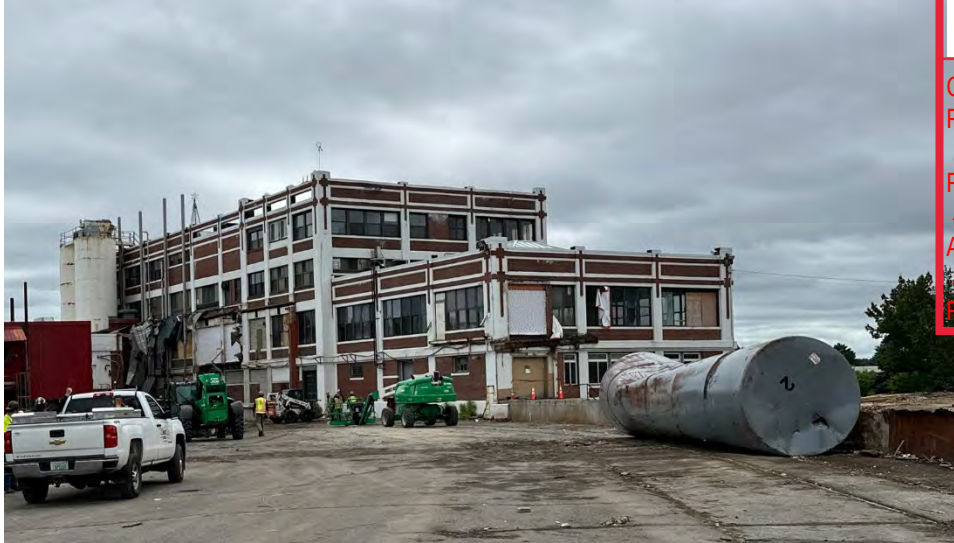
Existing conditions- north facade
