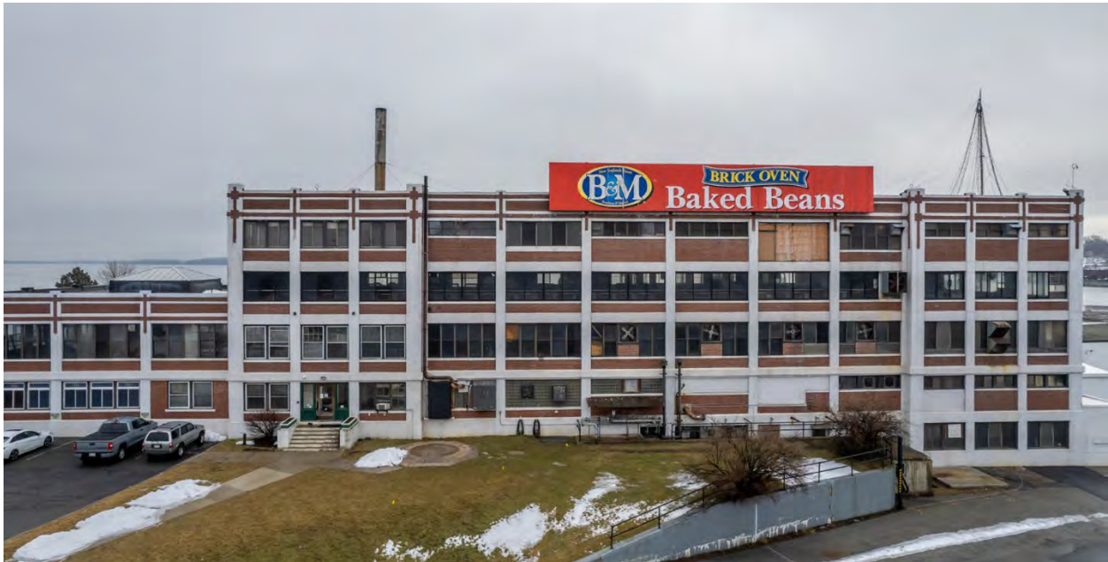
Existing conditions- west façade
