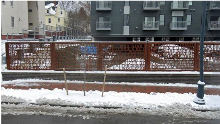
Figure A: Precedent image to screen transformer adjacent to public sidewalk. Image courtesy of Google Maps
