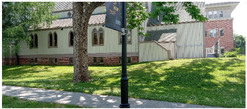
5 PHOTO FROM CAMPUS GREEN LOOKING SOUTH AND SHOWING REAR 1986 ADDITION
