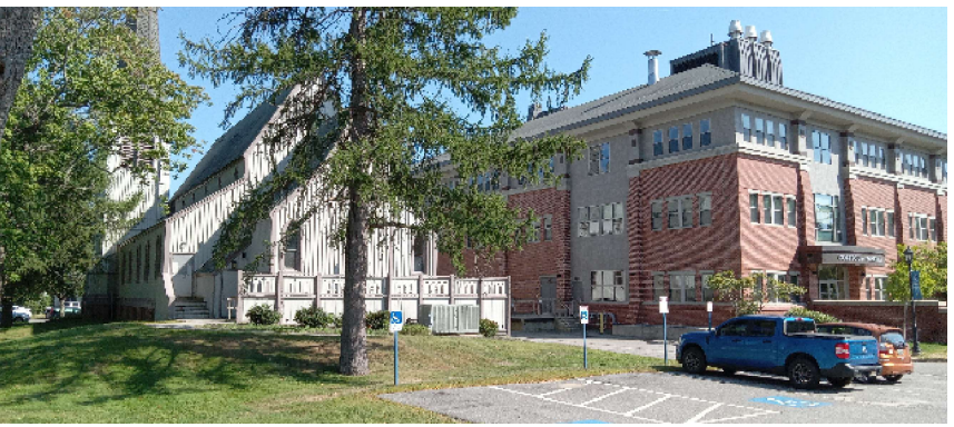
6 PHOTO FROM REAR DRIVE LOOKING EAST - SCHOOL OF PHARMACY TO THE RIGHT
