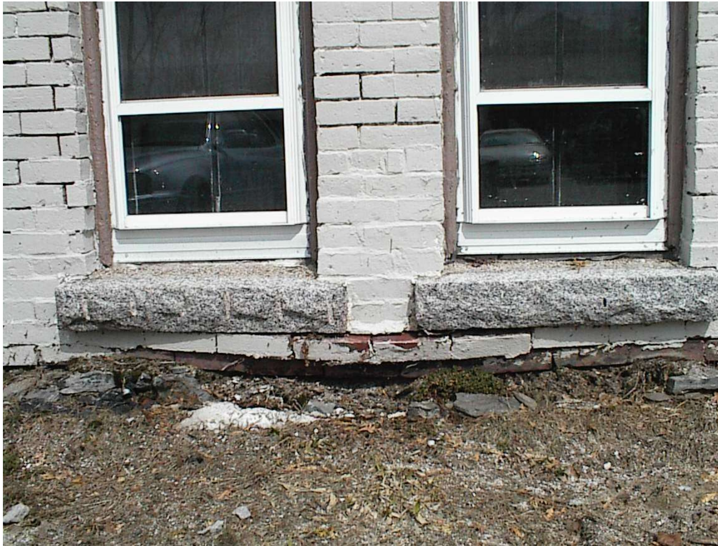
Previously Painted Brick Base
