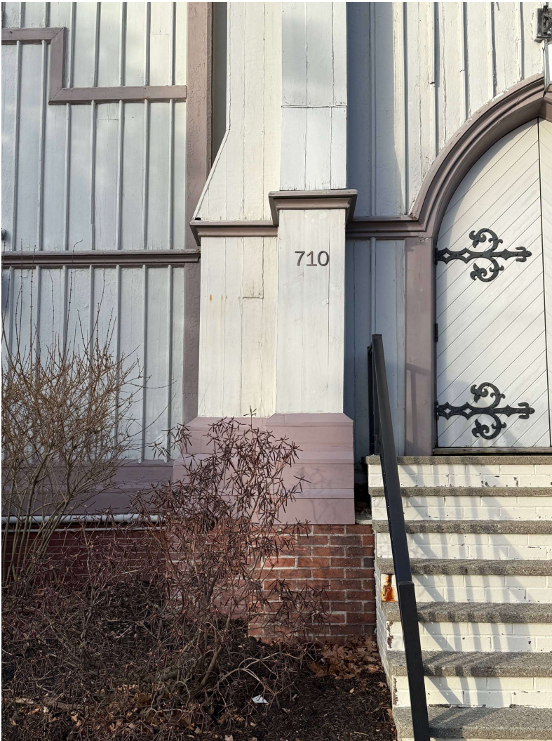
Front Tower Bottom Left Buttress
