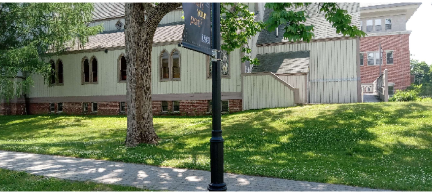
5 PHOTO FROM CAMPUS GREEN LOOKING SOUTH AND SHOWING REAR 1988 ADDITION
