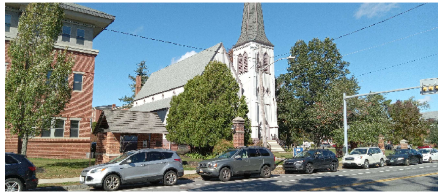
2 PHOTO FROM ACROSS STEVENS AVENUE LOOKING NORTHWEST
