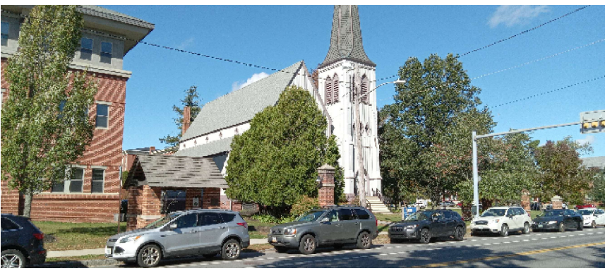
2 PHOTO FROM ACROSS STEVENS AVENUE LOOKING NORTHWEST
