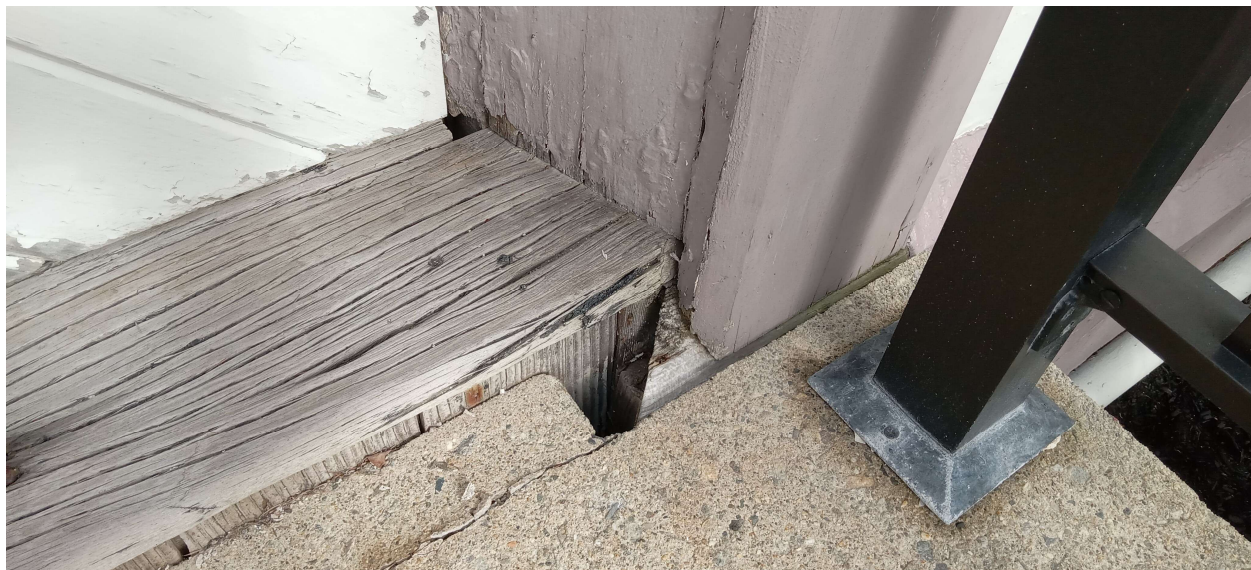
Entry Threshold to be Reworked
