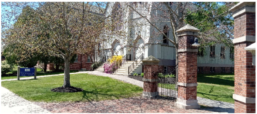
4 PHOTO FROM SIDEWALK LOOKING SOUTHWEST AND SHOWING ENTRY TO CAMPUS GREEN
