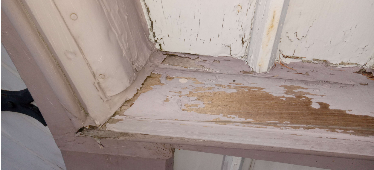
Spring Line at Tower Door
