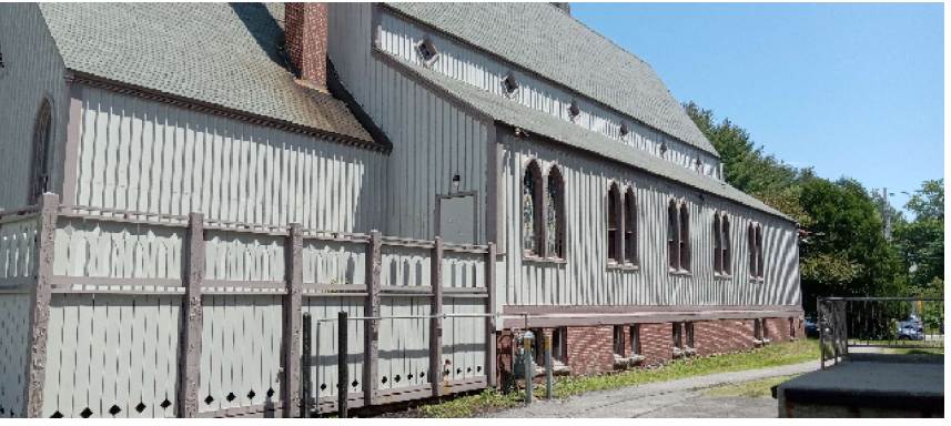
8 PHOTO FROM ALLEYWAY BETWEEN LUDCKE AND PHARMACY LOOKING EAST
