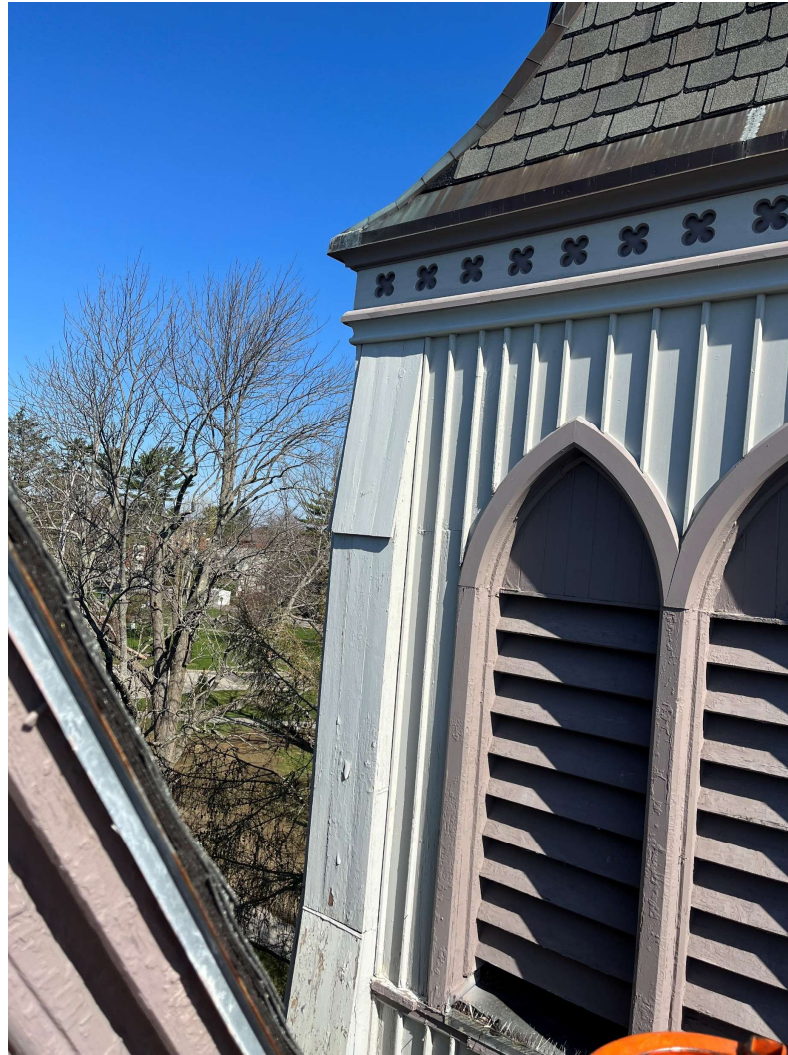
South Facing Louvers and Eave at Tower
