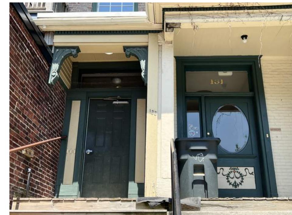
View of 133 and 131 Spring St entry doors
