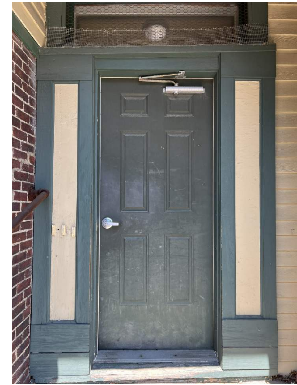
View of 133 Spring St entry door
