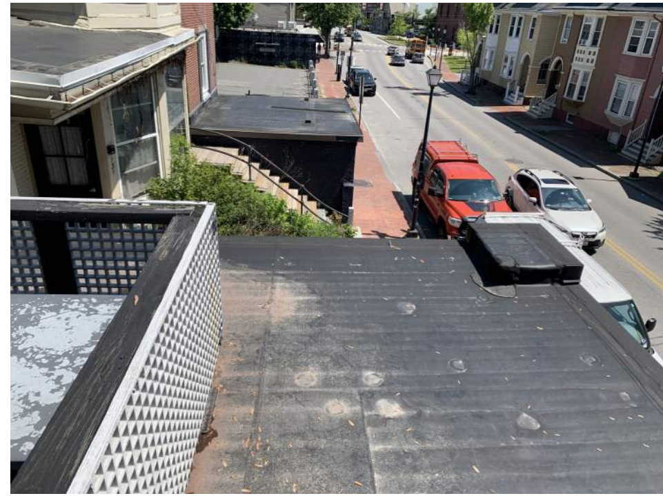
View of restaurant roof
