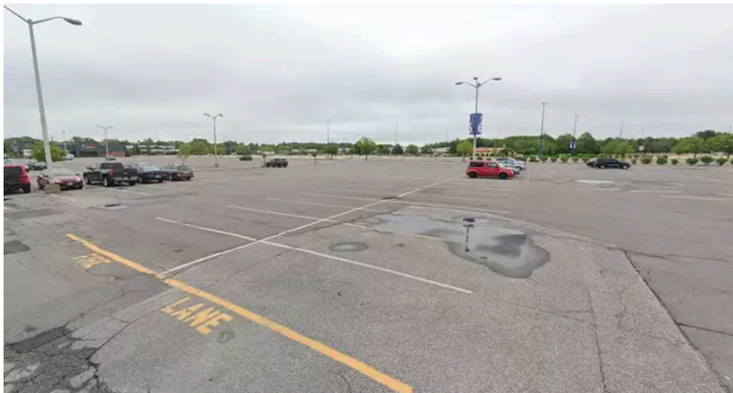
Figure 9: Maine Mall Parking Lot, South Portland, ME
