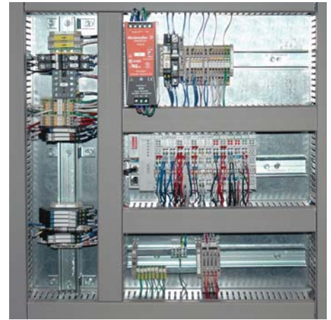
Field connection wiring is easily accessible in a dedicated section (lower left) of the control panel.
