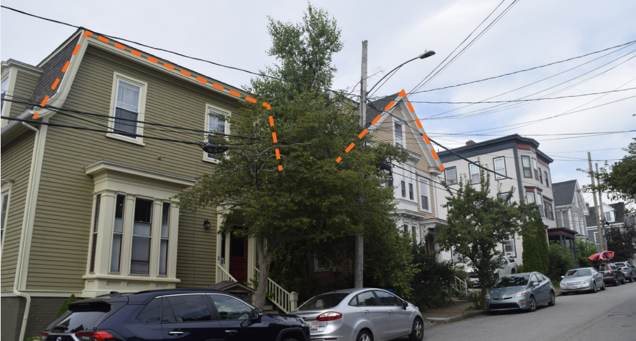
Many areas, such as along this stretch of O’Brion Street feature a wide variety of roof shapes.
