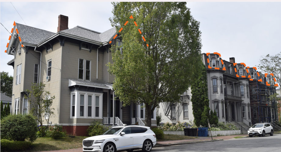
Some areas, such as these sections of Pine (left) and Thomas (right) Streets feature roof forms that are articulated by a variety of dormers and cross-gables.
