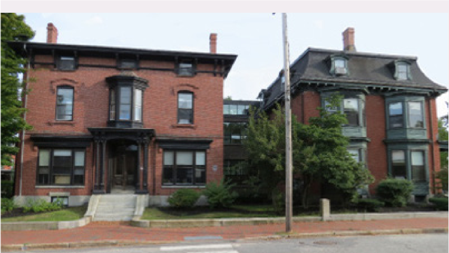
The Seth C. Deyer House (1867, 338 Spring Street, left) and the John Randall House (1860, 342 Spring Street, right) are now a part of the Waynflete School. As part of their rehabilitation to an academic use, a rear addition was constructed to connect the structures. This addition is set well back from the building facades and is recessive in design and color, allowing the two historic buildings to continue to read as separate structures. The addition also uses a higher proportion of glass and simple contemporary details to differentiate itself from the more solid and ornate historic structures.
