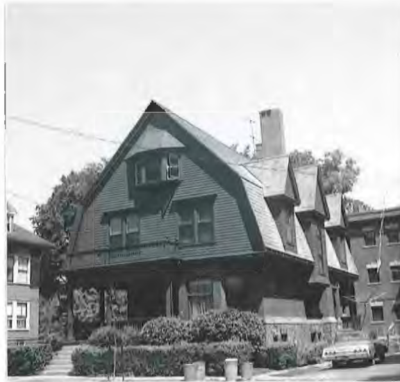
Architect Frederick Thompson designed and built his own Shingle style residence at 33 Carroll Street in 1901. Characterized by a gambrel roof, deep dormers, shadowy porch cut out of the main block of the building and a variety of materials including brick, shingle, and stone, this landmark quality is similar in scale, mass, setback and materials to its compatible but less architecturally distinguished neighbors.
