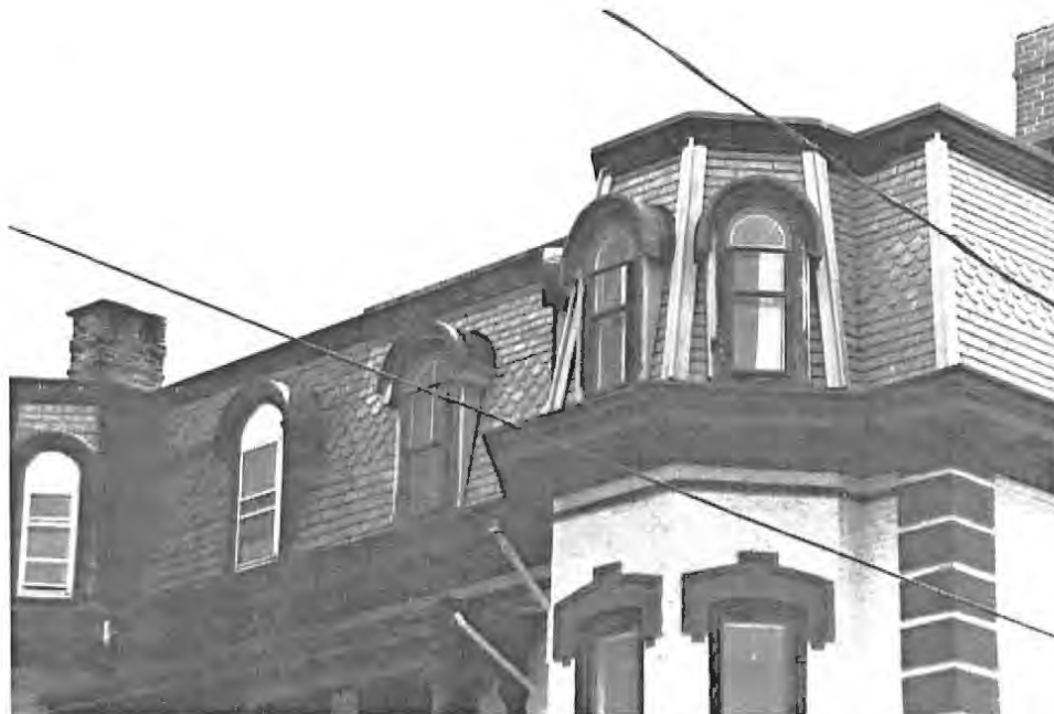
Sometimes a substitute material may be used to replace a deteriorated feature. The mansard roof on this double house retains its original slate on the left side while that on the right side has been replaced with "Supra-Slate", a mineral fiber-shingle product. This new material matches closely the design, color, and texture of the original slate.
