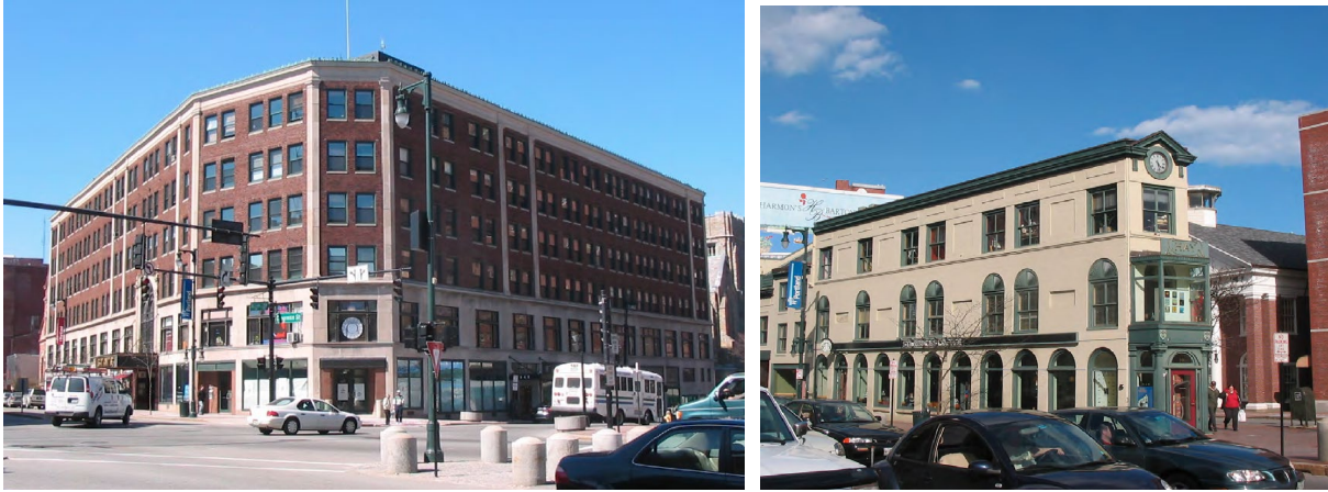
Figure 4: 2006 views of the Congress Building (left) and Charles Q. Clapp Block (right).
