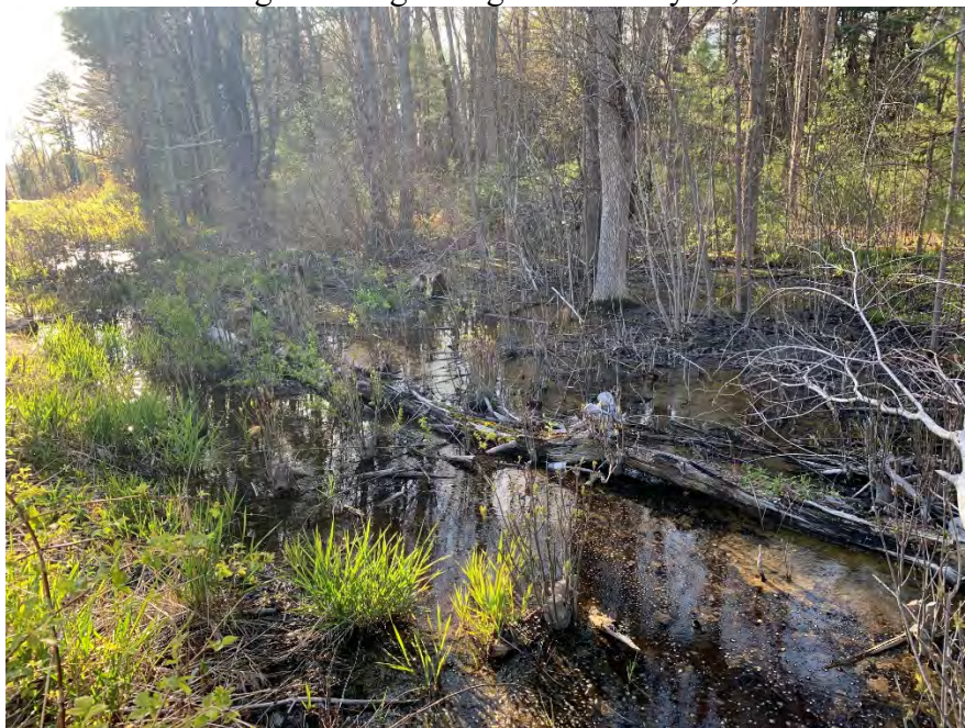
Drainage/Pooling Along Road – May 12, 2020
