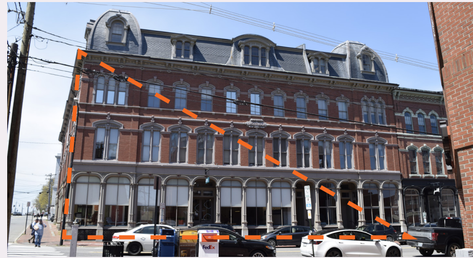
Along Middle Street, many properties exhibit consistently horizontally proportioned facades.
