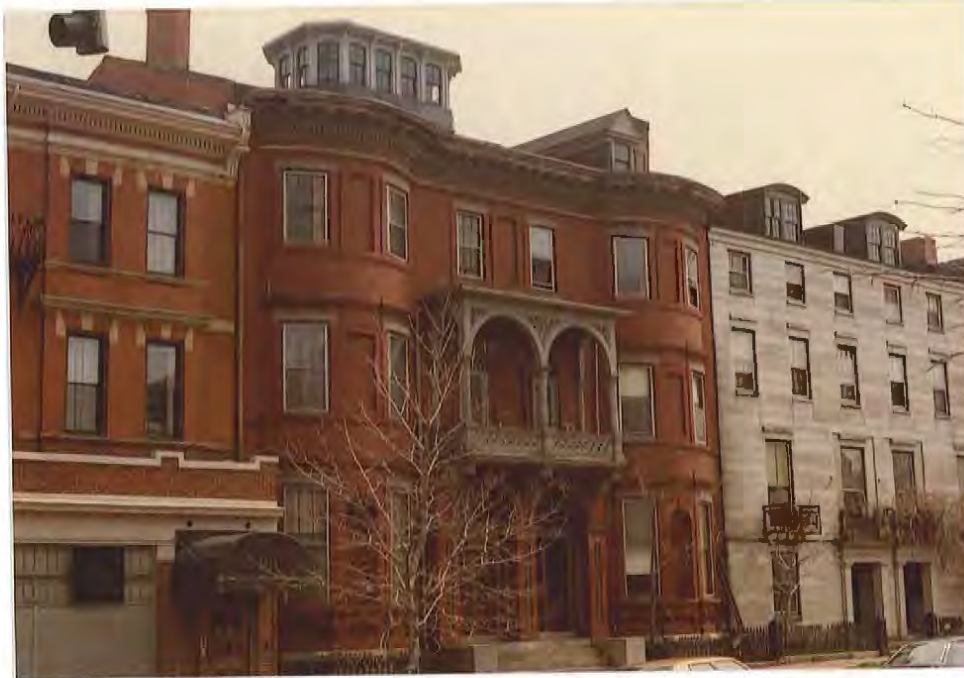
Building types represented in the district include many variants on the double house. Two quite different examples of this type, the Fitch-Swan House (1859) and the John Neal Block (1836) are located on State Street near Longfellow Square. The Greek Revival granite Neal Block seems almost severe next to the undulating bays and pierced wood balcony of the Italianate painted brick Fitch-Swan house. Although the buildings share a similar height, width, and setback, the marked differences in their ornamentation and detailing makes for a visually stimulating streetscape.
