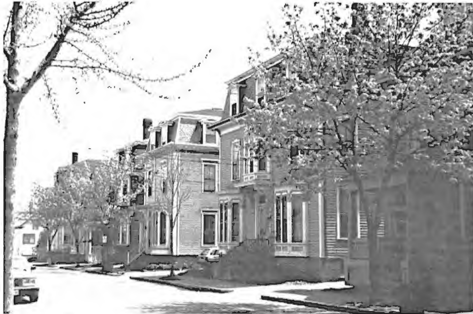
The spacing of these detached houses on Cushman Street is consistent for the entire block. Even though the sideyards are minimal, they create a very different rhythm from that of a block of rowhouses, one that is important historically and architecturally.
