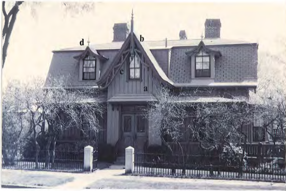
Gothic Revival Style William Goodwin House, 75 Vaughan Street, built 1859 a) board and batten; b) gable; c) bargeboards; d) finial
