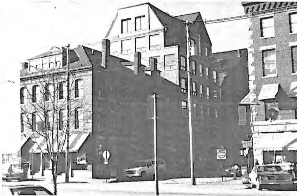
This new commercial building in the Old Port is located on a crowded site on Moulton Street, but is perhaps most visible from Commercial Street. The multi-faceted roofline is successfully used to reduce the apparent height of the building and to harmonize with the gable, hip and gambrel roofs of its neighbors on Fore Street and Commercial Street.
