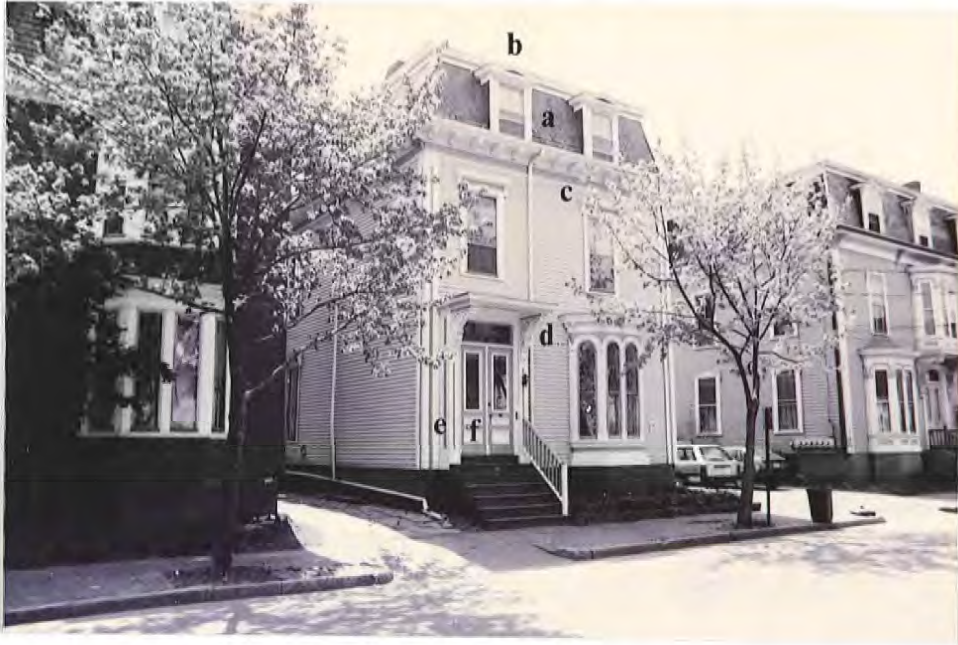
Second Empire Style Stephen R. Small House, I, 18 Cushman Street, built 1870 a) mansard roof; b) pediment; c) cornice; d) brackets; e) corner boards; f) double leaf entrance
