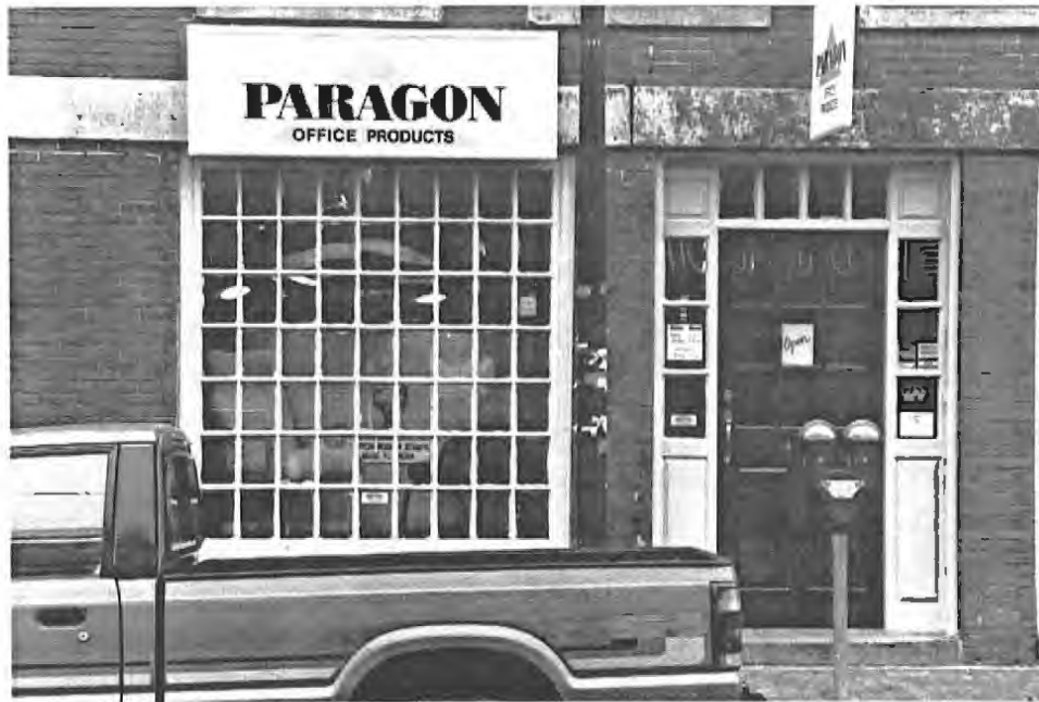
Small-pane storefront windows and residential entrances were not used historically in commercial buildings. Simpler window and door designs would complement the straightforward Federal lines of this building.
