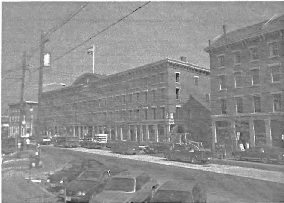
The Thomas Block on Commercial Street is a uniquely wide building with a commanding presence and remarkable consistency on the street. At the pedestrian level, this width is broken down to a more human scale by the steady march of granite piers. Within the piers, storefront windows and doors establish another unit of width for pedestrians to relate to.
