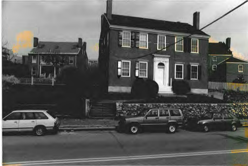
The Daniel How House, 23 Danforth Street, was built in 1799 in the post Revolutionary War expansion of Portland economy. The dwelling is, in style, conservative late Federal. The outstanding feature is the entrance surmounted by entablature and cornice supported on Doric pilasters. To the right and left in the background are the two other How Houses.
