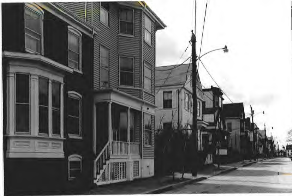
The area comprising Brackett and Winter Streets was once part of Anthony Brackett's farm and was subdivided in the 1840's and 50's following his widow's death. Winter Street, shown above, includes both brick and frame structures, predominately in the Greek Revival and Italianate styles. Most structures in this section of the district were built by local carpenter/builders in vernacular adaptations of the fashionable architectural styles of the day. The vernacular houses tend to exhibit less elaborate trim details and materials than their high style counterparts.
