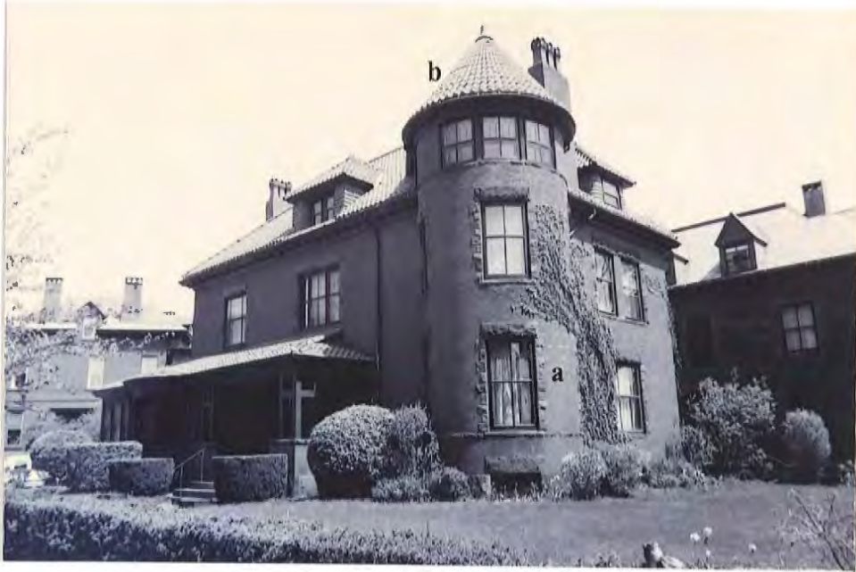
High Victorian Gothic Style Harry Butler House, 1 Thomas Street, built 1892-1894, designed by John Calvin Stevens, I a) molding; b) conical roof
