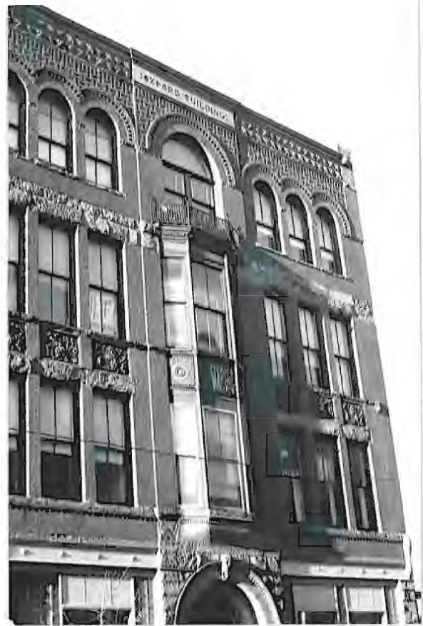
The Oxford Block, 183-187 Middle Street. John Calvin Stevens I's Romanesque Revival business block built in 1886-87. Decorative brickwork, terra cotta panels, carved stone and metal balcony extend the richness of the arched openings and projecting bay. Whether articulated in this later Romanesque style or in earlier styles, this richness of detail is characteristic of much of the architecture of the waterfront district.
