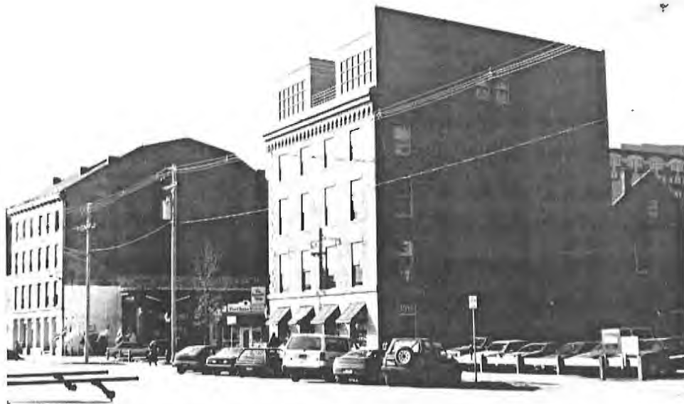
The roofline is often an important character defining feature that should be respected. Here, the once prominent gambrel roof, typical of warehouses in the waterfront district, has been irreversibly altered by this rooftop addition which sits flush with the plane of the perimeter walls. The change is brick on the extended side wall is the only indication of the original roofline. Were the addition pulled back from the perimeter walls and integrated within the gambrel roof form, a more successful solution would have resulted.
