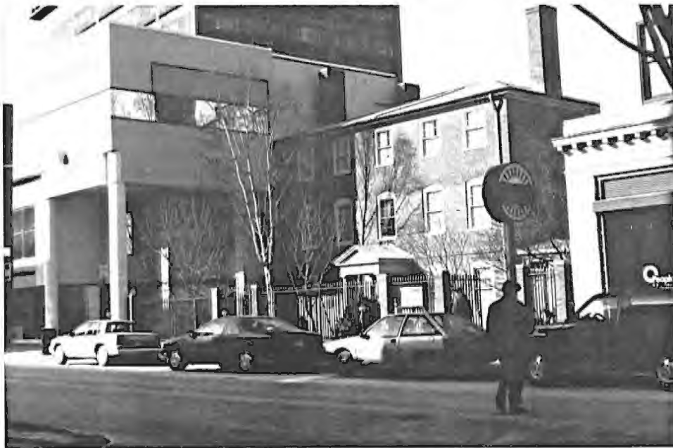
While the use of modern building materials in historic districts is not discouraged, their compatibility with their immediate context should be carefully considered. Here, at 489 Congress Street, both the materials themselves and their coloration stand in sharp contrast to those of the Wadsworth-Longfellow House and serve to overwhelm the more restrained landmark building.
