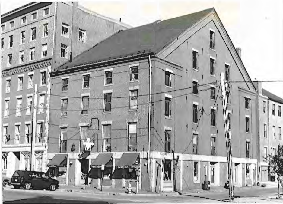
William Moulton Block, 157-163 Commercial Street. In 1851 it was one of the first blocks built on Commercial Street. The Greek Revival stylistic features are the wide granite lintel which separates the first story from the upper floors and the heavy granite lintels over each window. Noteworthy on the side elevation is the deep return of the gable which is supported on each side by brick pilasters.
