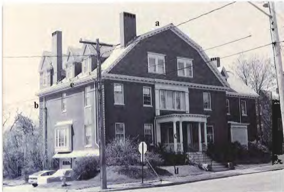
Colonial Revival Style Franklin C. Payson House, 28 Bowdoin Street, built 1901, designed by John Calvin Stevens, I a) gambrel; b) quoins; c) column; d) balustrade; e) modillions
