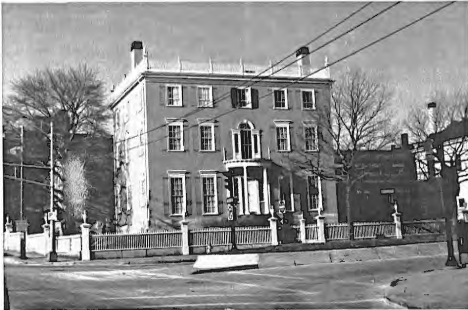
The proportions of Federal-style houses contribute to their elegance. The ratio of width to height of the entire facade and of windows and doors within the facade of the McLellan-Swett House was based on ancient principals going back to the Romans. These proportions were standardized to a degree by the builders of the day, and can be seen in the large Federal houses along State and High Streets and on Danforth Street.
