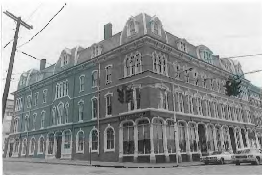
Woodman Building, 133-141 Middle Street. The tall cast iron columns, the elliptical arches, the prominent belt courses, and window hoods enliven and break into smaller components an otherwise massive building. Noteworthy are the groupings of windows which define the corners and the centers of the two facades.
