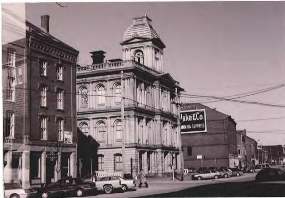
The Customhouse on Fore Street replaced a structure lost in the 1866 fire, and was finished in 1871 from designs by architect, Alfred B. Mullett. It is an outstanding example of the Second Empire Style. Here grey granite is used to create strong light-dark contrasts in the projecting columns, the recessed windows, fine roofline, balustrade and surrounding fence. A building of this scale and richness needs generous views -- this was designed to be seen from four sides.
