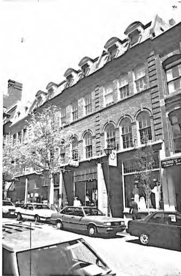
The same is true for many smaller buildings in the Old Port. In this photograph a large commercial building is divided into typical storefront bays by storefront piers, upper story pilasters, and roof parapets to correspond with the more common single-bay structures along Exchange Street.
