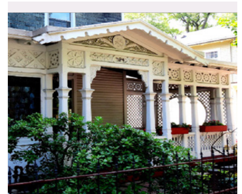
The Edward A. Noyes House (1870, 394 Danforth Street) features elaborate wooden details at the porch and cornice. Additionally, the building is clad in slate siding, which was an unusual and distinctive design choice.
