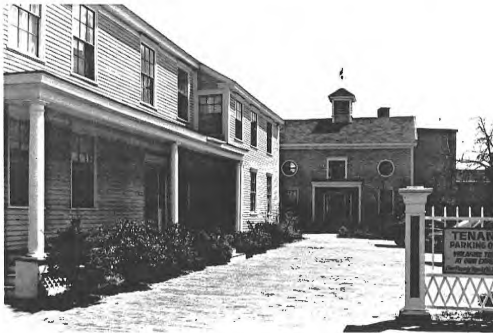
Here, although there has been an intensification of use, changes to the building and the site are not readily apparent from the street. Additions have been made off the sides and rear of the building and parking has been limited to an area obscured by the fence. The sense of an open courtyard leading up to a carriage house has been retained.
