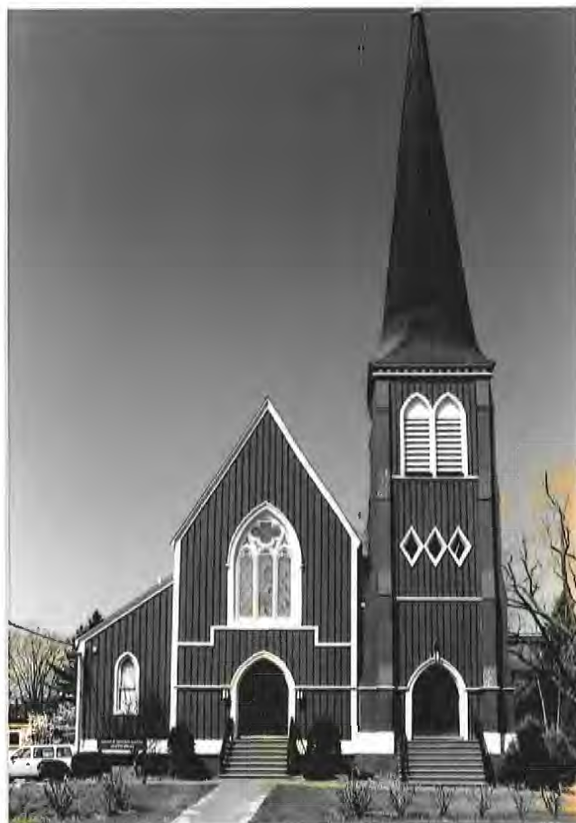
Universalist Church (Westbrook College Auditorium) of 1867, designed by Francis H. Fassett is a Gothic Revival structure with characteristic board and batten exterior, pointed arched openings and steep roof. Fassett designed many masonry structures in Portland as well as a quantity of wooden buildings. This structure stands apart from the other campus buildings and faces directly on Stevens Avenue thus emphasizing its direct relation to the community historically and in the present.
