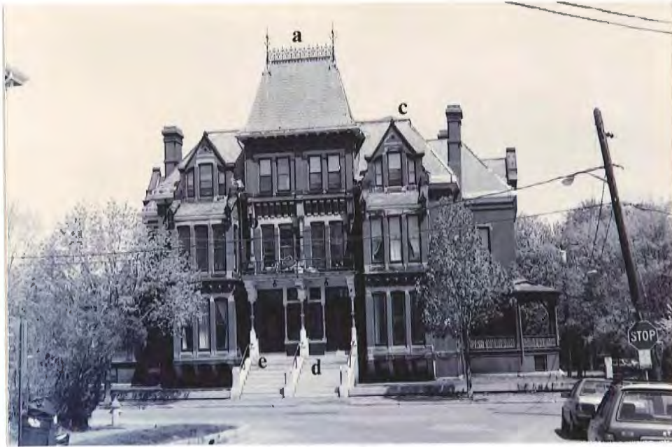
Francis H. Fassett Residences, 117-119 Pine Street, built 1876, designed by Francis H. Fassett a) cresting; b) brackets; c) gables; d) portico; e) colonette; f) string course
