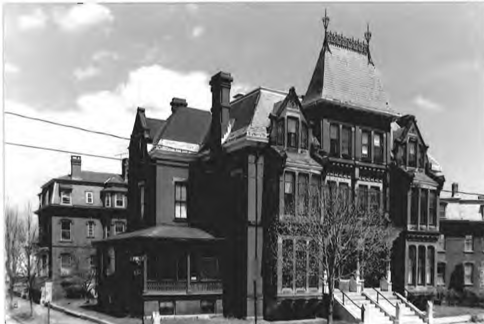
Many architects built homes for themselves in the fashionable Western Promenade district. Architect Francis Fassett chose a Pine Street location for his own imposing High Victorian Gothic residence, built in 1876. A catalog of architectural detail, the double house features very tall narrow windows, pointed gables, a steep slate roof with crested tower, and red marble columns to support the entrance portico. Site prominently on the corner of Pine and Carleton Streets, the building is a landmark both for the quality and richness of its architecture and also because it serves as a visual terminus from a number of streets.
