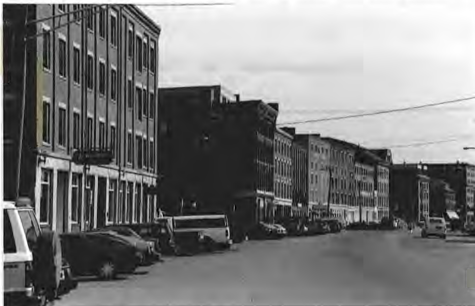
Commercial Street is flat and unusually broad. Wide blocks of four and five storeys balance the breadth of the street. First floor facades and strong cornice lines are important unifying features in this wall of buildings. Because of the breadth of the street, changes to rooflines are especially noticeable. Some of the recent rooftop additions have broken the consistency of the street.
