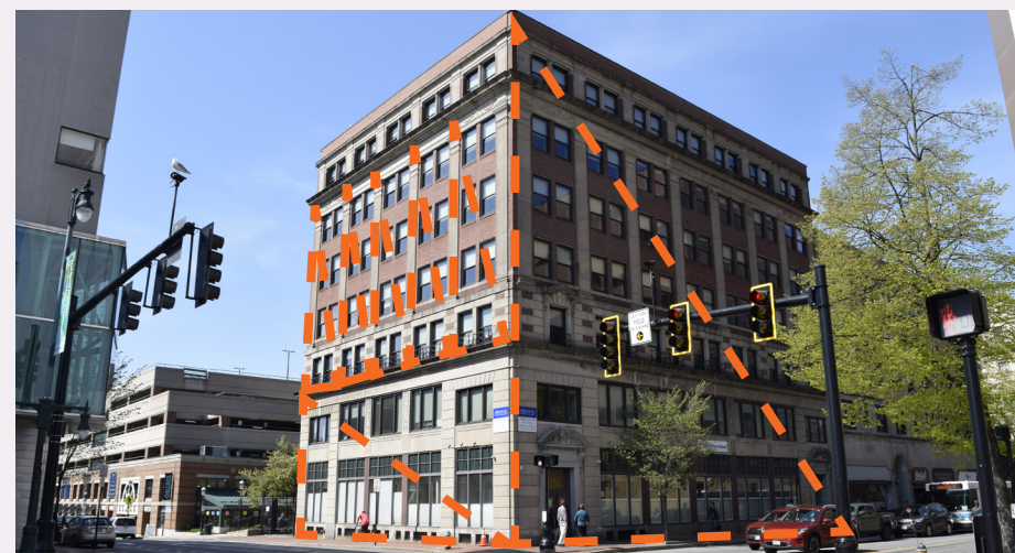
Some buildings, such as these along Congress (left) and Exchange (right) Streets exhibit a mix of proportions.
