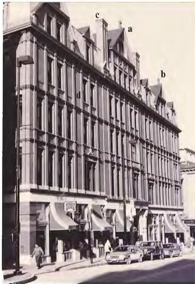
Queen Anne Style John B. Brown Memorial Building, 1882-1883, 523-543 Congress Street, designed by Francis H. Fassett a) gable; b) finial; c) chimney stack; d) pilaster
