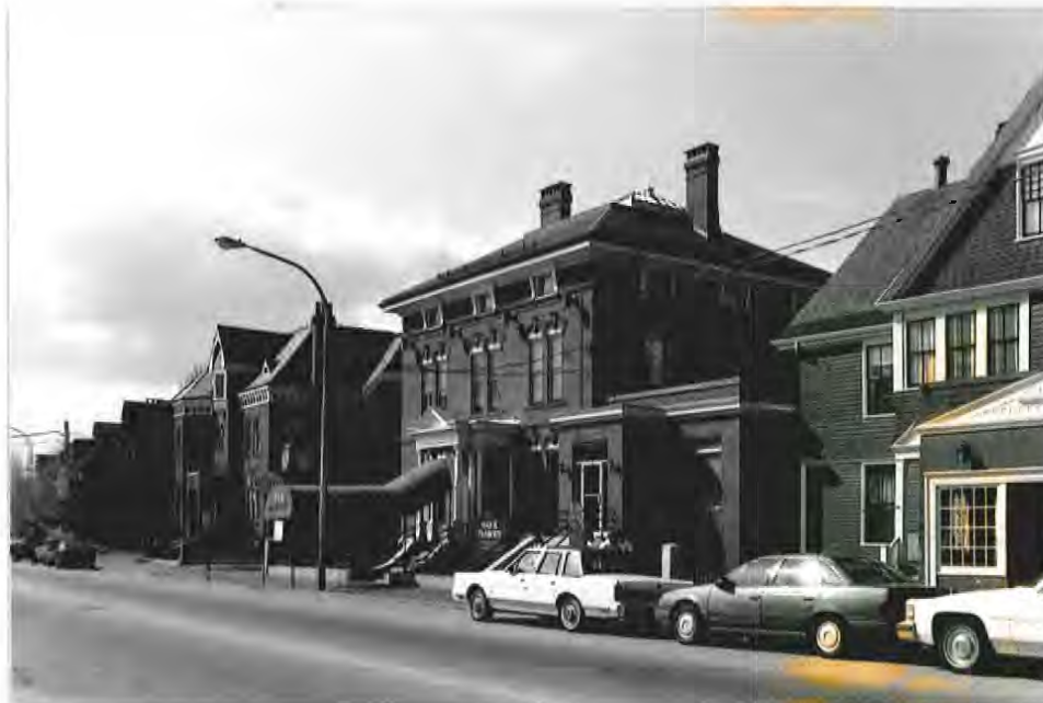
Several architectural styles and building materials are displayed in this group of Congress Street converted houses. Nevertheless, the shingle and clapboard Queen Anne style Samuel T. Pickard House on the right is similar in setback, scale and building height to the brick Italianate house in the center and to the brick Queen Anne style house on the left.
