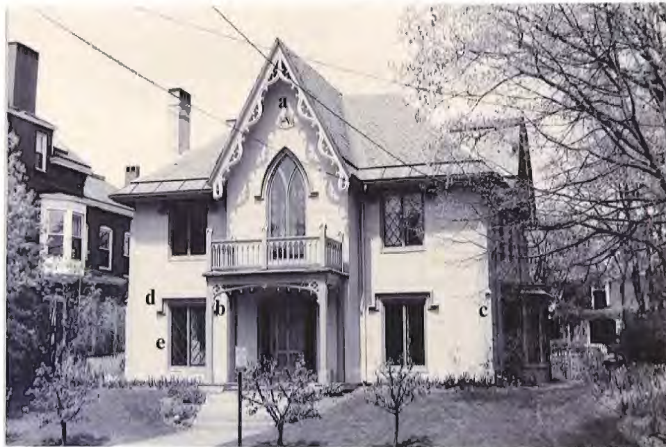
Gothic Revival Style John J. Brown House, 387 Spring Street, built 1845, designed by Henry Rowe a) gable; b) portico; c) pier buttress; d) drip molding; e) leaded panes
