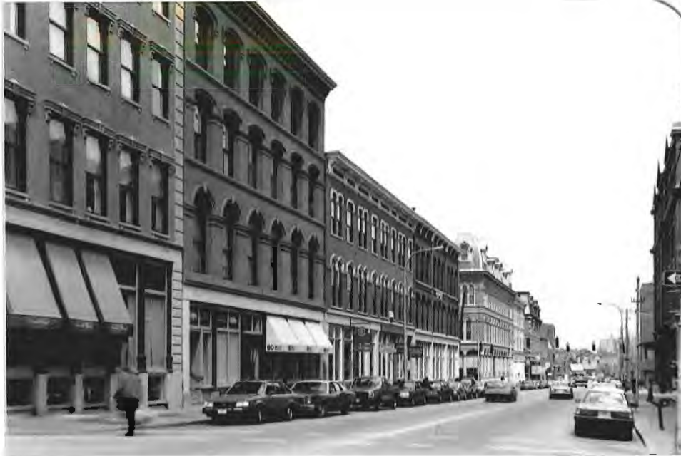
Middle Street. The Woodman, Thompson and Rackleff blocks are visible on the lower left. The importance of the first storey definition is apparent as is the rhythmic repetition of vertical window openings. The depth of the windows and the projection of the moldings are important design elements which provide relief and richness of detail.
