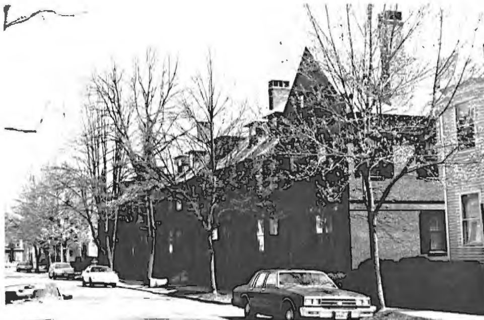
Attached rowhouses like these on Neal Street can have both horizontal and vertical expression. In this case, the vertical line established by projecting bay windows and projecting wings at the center and both ends are counteracted by the sweeping roofline. Walking along the sidewalk in front of the building, one senses the vertical nature of individual townhouses. From across the street, however, the overall image of a single building dominates. This dichotomy could become a primary design determinant of a sensitive new design in an infill situation.
