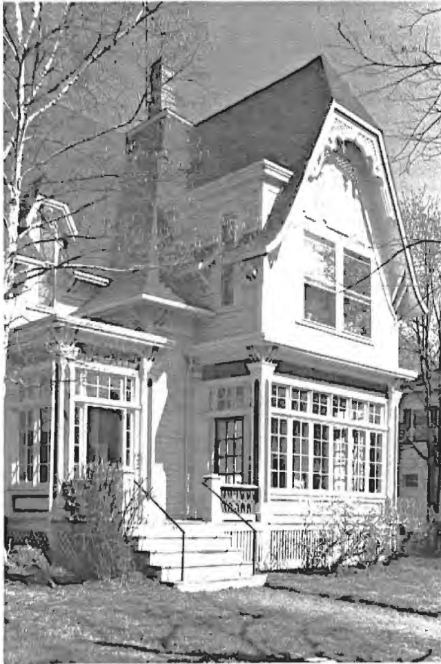
The skilled craftsmanship displayed in this Swiss style house is evident in many of its features. Its complex massing and roofline, its pierced vergeboard and gable panels, its sawn balusters, its multi-part windows, and its polychromatic paint scheme all help to define its historic character.
