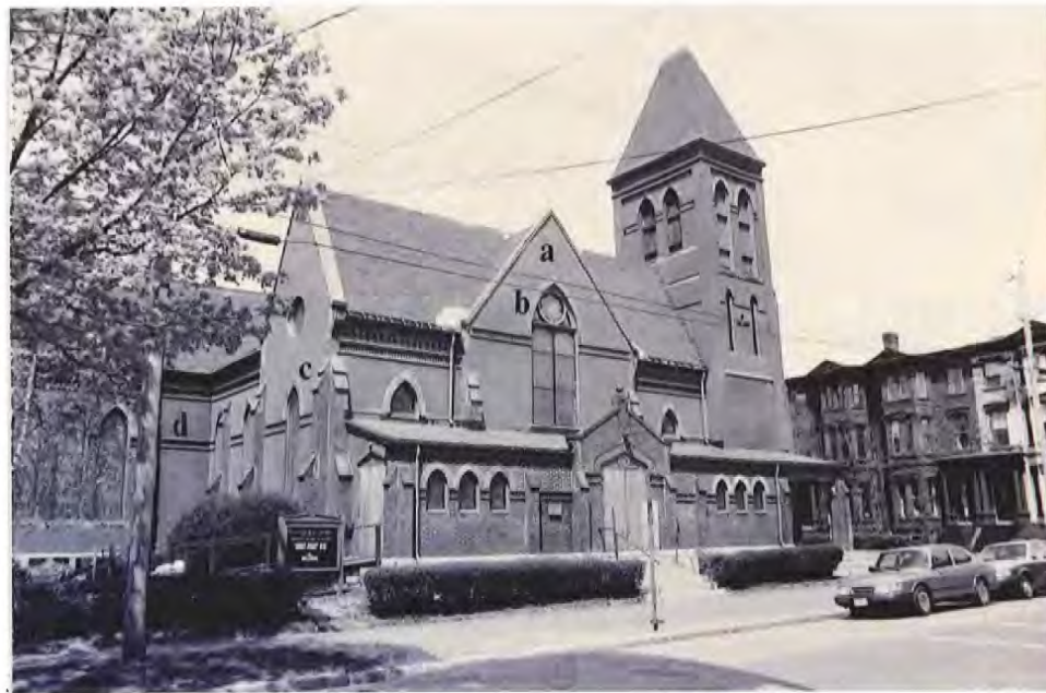
High Victorian Gothic Style Williston Congregational Church, 32 Thomas Street, built 1877, designed by Francis Fassett a) gable; b) pointed window; c) pier buttress; d) string course
