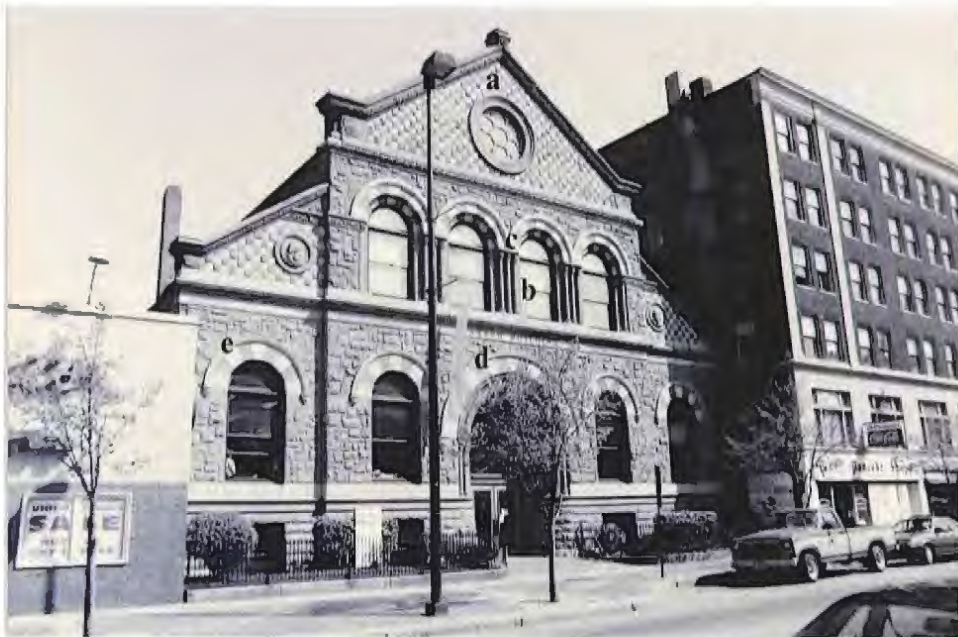
Romanesque Revival Style Baxter Building, Congress Street, built 1888, designed by Francis H. Fassett a) gable; b) colonette; c) capitals; d) "nave"; e) "side aisles"
