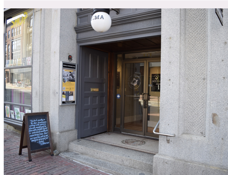
When a new air-lock entry was needed to improve the functionality of the main entrance at Mechanic's Hall (1857, 519 Congress Street), it was constructed inside the building, leaving the original wood paneled doors intact. The wood doors remain visible when open, and are pulled shut after business hours.
