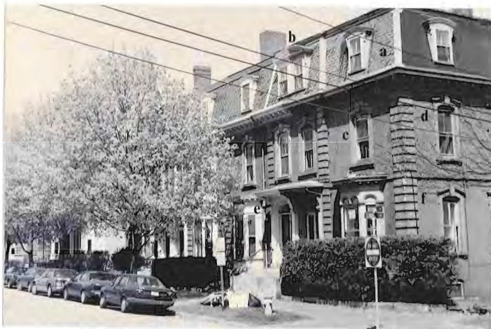
Second Empire Style Simon H. Libby Block, 33 - 39 Deering Street, built 1866 a) mansard roof; b) pediment; c) moldings; d) key stone; e) brackets; f) quoins
