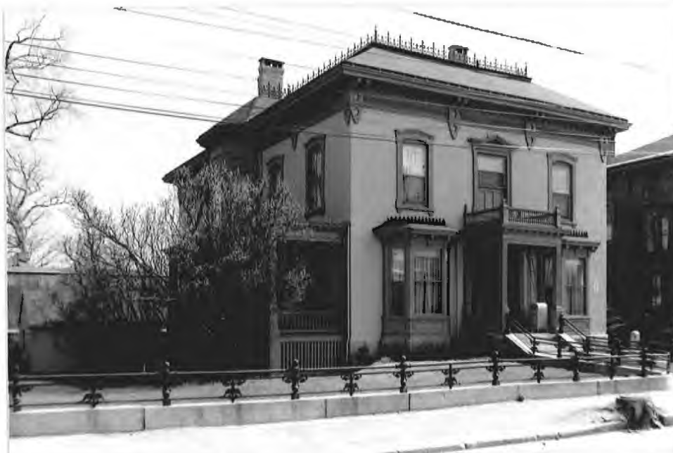
The George P. Westcott house at 364 Spring Street is a symmetrically planned painted brick Italianate style residence built in 1874. It exhibits the shallow setback with wide side yards, the large mass, and the careful articulation which are characteristics of numerous buildings in the district. Remaining original details, such as the granite and iron fence, delicate iron cresting on the hipped roof, balustrade surmounting the portico, and pierced brackets at the eaves are important to the integrity of the design.
