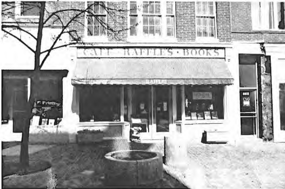
This close-up of a commercial facade at 565 Congress Street shows how an individual storefront relates to the pedestrian. The width of the storefront, the size of the door, the height of the display windows, even the placement of the door within the storefront represent traditional design patterns that humans relate to from years of use and familiarity. This is a new storefront, built with modern and traditional materials, that adheres to traditional storefront design patterns while presenting a clean contemporary look.
