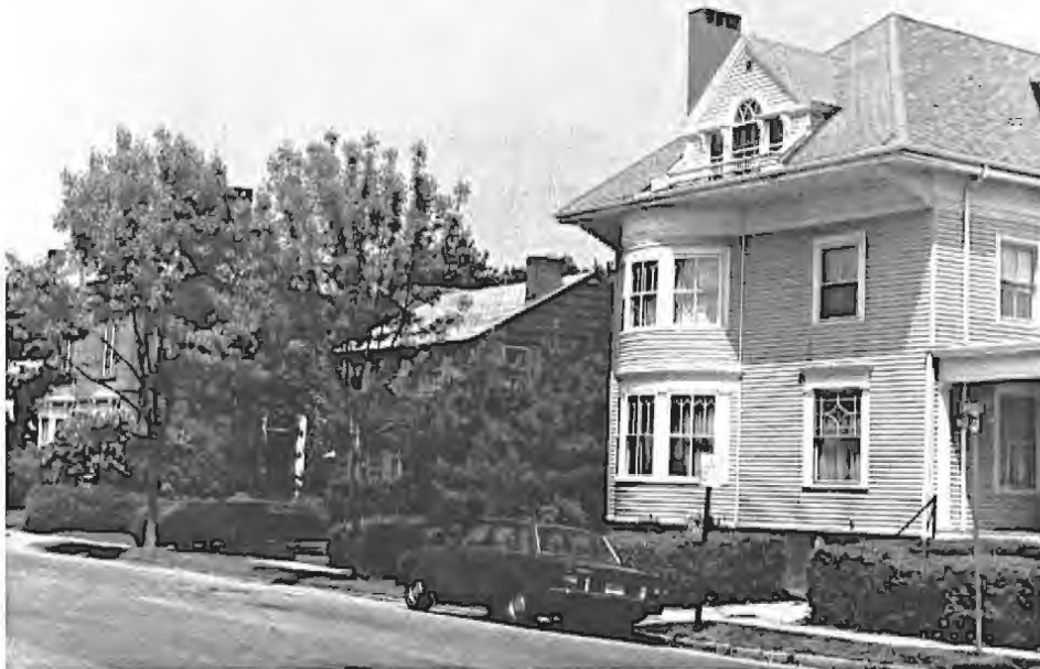
Just as new buildings can be too large for their context, too small a structure can also break the continuity of an established district. The garrison colonial style residence on Vaughan Street in the center of this photograph is significantly smaller than its historic neighbors, not only in terms of its height, but also in its width, overall scale and mass.
