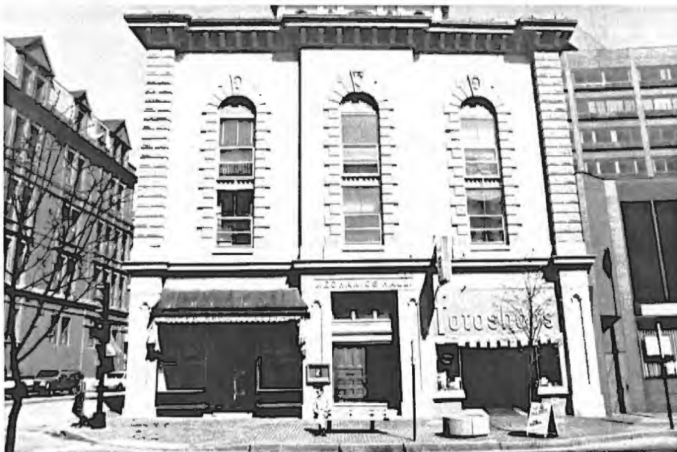
To acquire significance of its own, an altered storefront must be of high quality and an excellent example of its own design period. Also, it should generally be compatible with the rest of the building. Although it was constructed of good quality materials, the storefront on the right has not acquired significance because it is not an outstanding example of its own design period nor is it compatible with the original design of the building. In this case, the left storefront might serve as a template for a future redesign of the right storefront.
