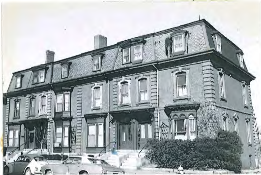
One of several house types found in this district is the rowhouse. 33-39 Deering Street was built as four adjoining homes separated by party walls with individual entrances for each family. Its symmetrical design, height and materials are similar to that of neighboring homes of single family and duplex types.
