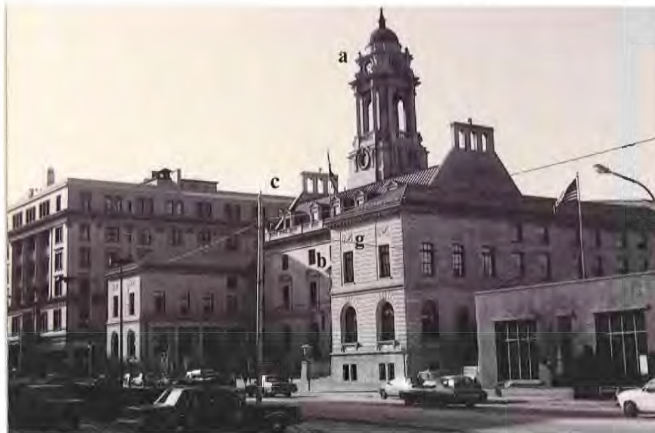
Classical Revival Style Portland City Hall, built 1902-12, designed by Carrere and Hastings; John Calvin and John Howard Stevens, local associates a) cupola; b) pediment; c) balustrade; d) column; e) pilaster; f) console; g) panel
