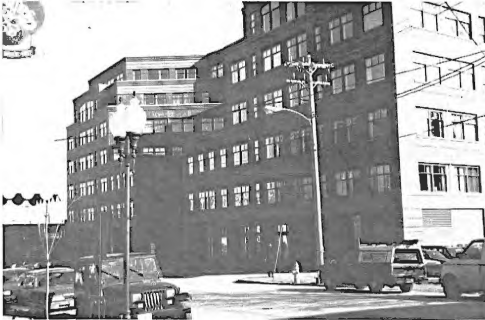
New office buildings at 100 Middle Street are at least two stories higher than any adjacent historic buildings; yet they have a comfortable presence on Middle Street due to their set backs and angled facets. In addition, the strongly-detailed first floor creates a base that anchors the building to the street. Breaking the height of the building into horizontal bands can reduce the perceived height of a large building.
