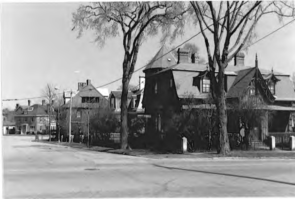
This photograph, taken from the corner of Bowdoin and Vaughan Streets, depicts homes of varying architectural styles and periods. Despite this diversity, the Gothic Revival William A. Goodwin house (1859) in the foreground is in its height, mass, setback, quality of materials and attention to detail similar to both the Second Empire James Olcott Brown house (1860) and the Colonial Revival Edward H. Daveis house (1890).
