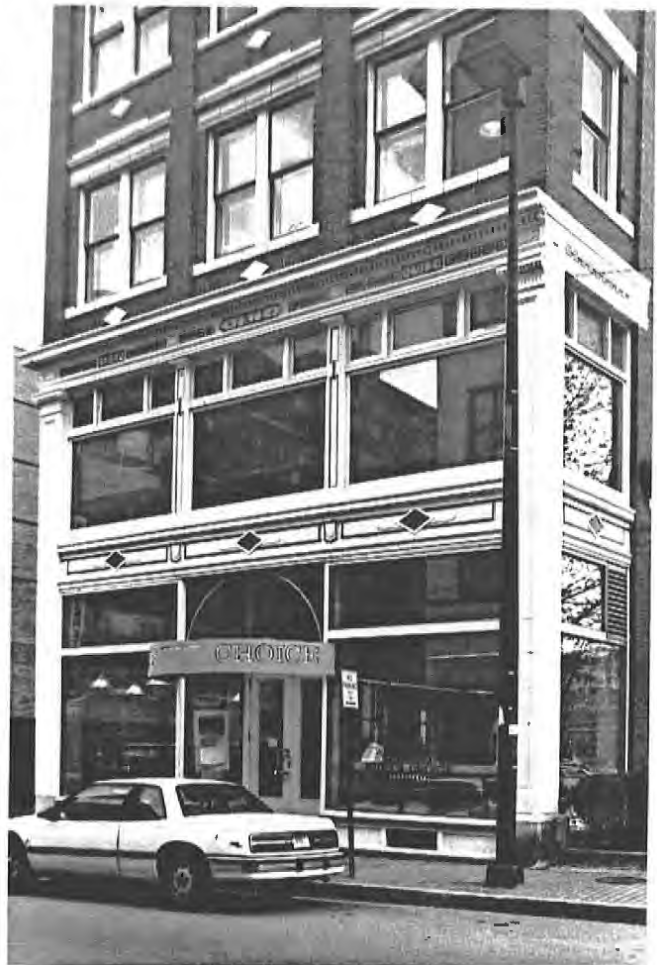
A contemporary design for a storefront in a historic building will be compatible if it follows the spatial organization of traditional storefront design. The proportions of the new storefront at the Frye Building were determined by the existing lower cornice and the vertical divisions in the upper stories.
