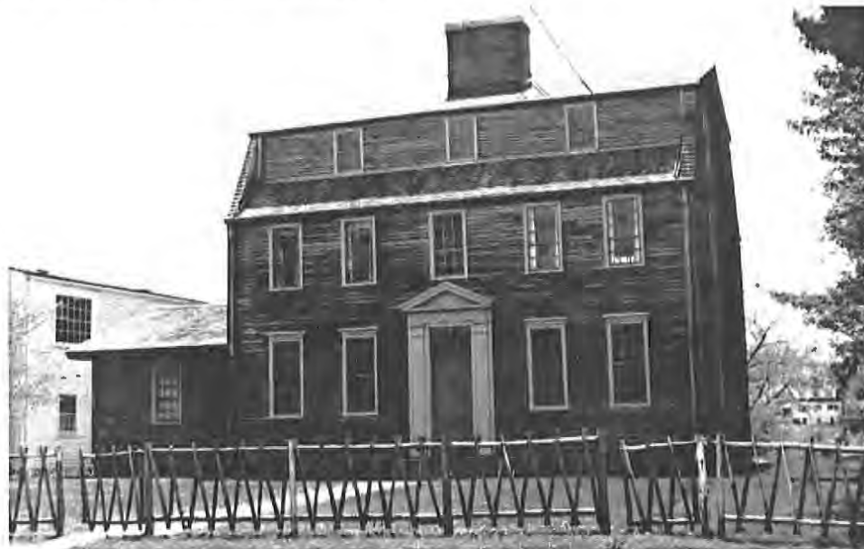
George Tate House, 1270 Westbrook Street, 1755. Built for the Royal Mast Agent George Tate, this dwelling was designated a National Historic Landmark in 1972, is one of the four earliest remaining structures and summarizes the importance of this village. The pedimented entrance door flanked with pilasters and crowns on the lower windows are typical mid-eighteenth century architectural details. The dormer cut into the gambrel roof is unusual, while the central chimney indicates the placement of the interior fireplaces.
