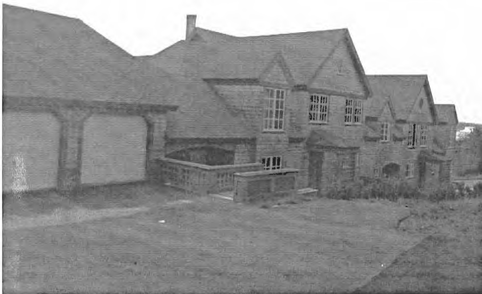
This group of condominiums on Danforth Street, the overall width of which is considerable, is divided by roof forms and entrance canopies into units of width that fit comfortably with other residences nearby.
