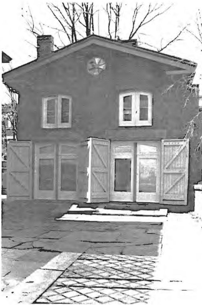
When the carriage house at the Victoria Mansion was adapted to become an architect's office, the original doors were fixed in an open position and new glass panelled doors were inserted in the openings. A second means of egress was located on the side elevation, not visible from the street. The new use was accommodated successfully without obscuring original key exterior features.
