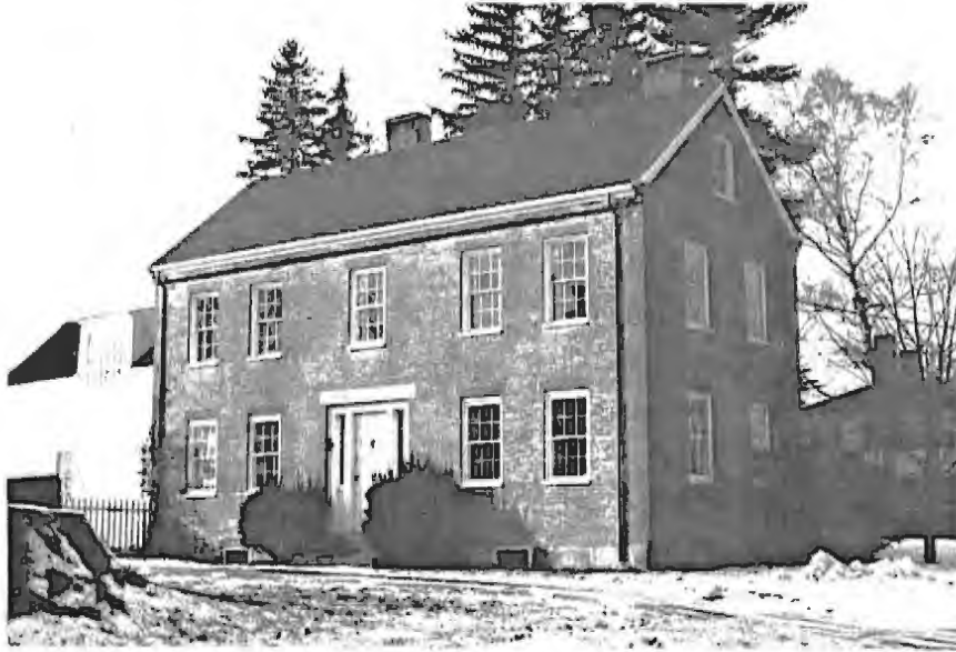
Martin Hawes House, 1266 Westbrook Street, 1835. This dwelling is sited with its gable end facing the street, is made of brick and is, in style, transitional from Federal to Greek Revival. The straight stone lintels are of the newer style while the height of the house and doorway configuration are more old fashioned. Its building coincided with the opening of the Cumberland and Oxford Canal.
