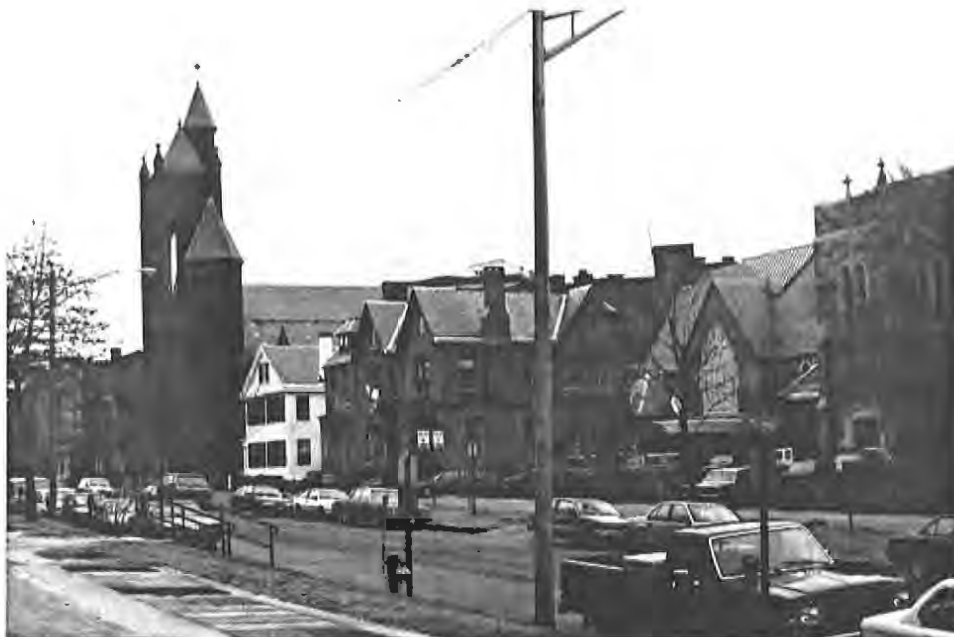
The substantial structures along State Street represent a diversity that can allow a great degree of freedom of design for infill construction. The many towers, turrets, dormers and cupolas set a precedent for any number of roof designs. As important in this case is the overall scale of these buildings, overall proportion of width to height, and the substantial amount of open space in front of and between each building.
