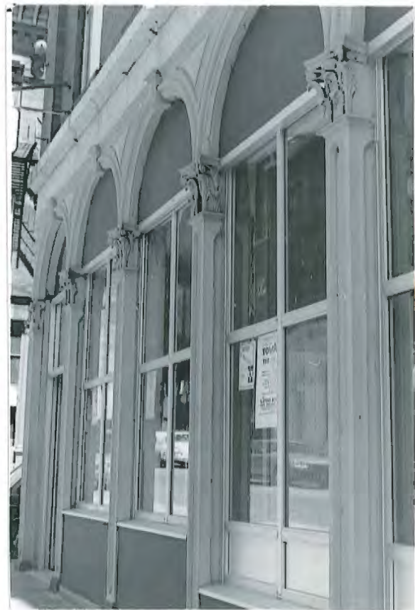
Ocean Insurance Company Exchange Street Block. Completed in 1867, the year following the Great Fire. The first story arcade is cast iron, an affordable material for such fine details as the corinthian capitals on the pilasters. Many commercial buildings in the waterfront district feature cast iron storefronts.
