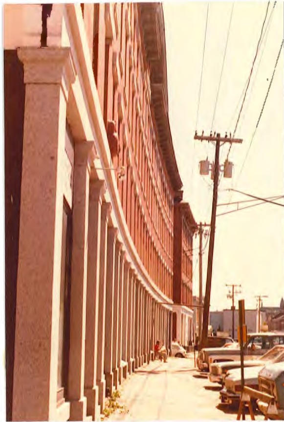
The Elias Thomas Block, 102-132 Commercial Street. Built in 1860, this granite and brick Greek Revival block is unusually long and was designed to reflect the curve of the street.
