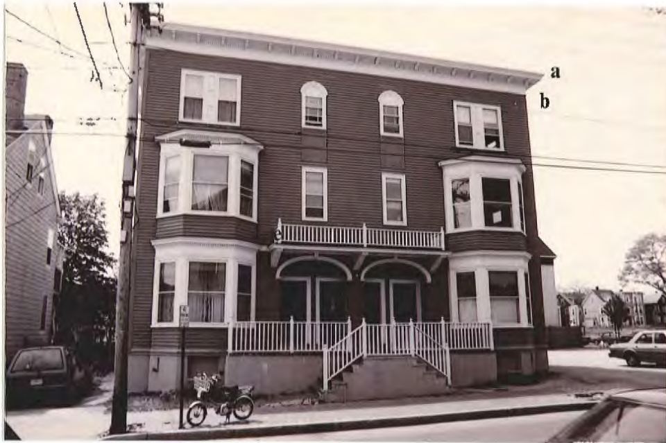
Colonial Revival Style 122-124 Brackett Street, built around 1897 a) cornice; b) modillions; c) elliptical arch; d) keystone; e) balustrade
