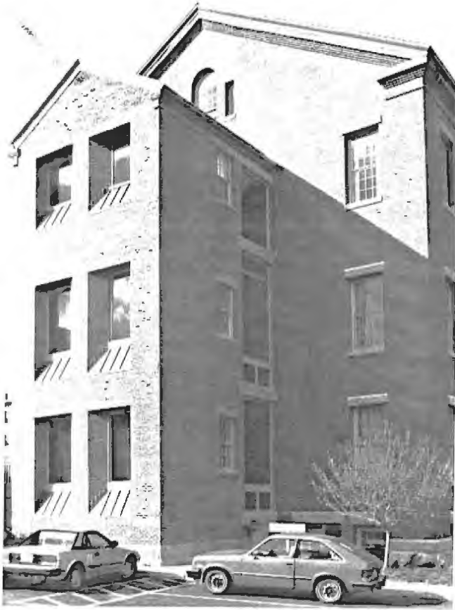
When a second stairway or an elevator cannot be accommodated within a historic building, a contemporary addition may be built for this purpose. Here the roofline, mass and fenestration pattern of the new Staples School stair tower compliments that of the main building. The point of connection where the addition meets the original building is clearly defined by an almost continuous wall of glass.
