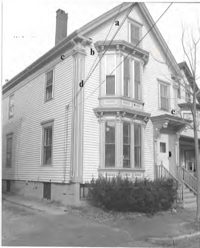
Italianate Style Elihu Hasty House, 53 Spruce Street, built 1874 a) gable; b) brackets; c) entablature; d) corner boards; e) hood
