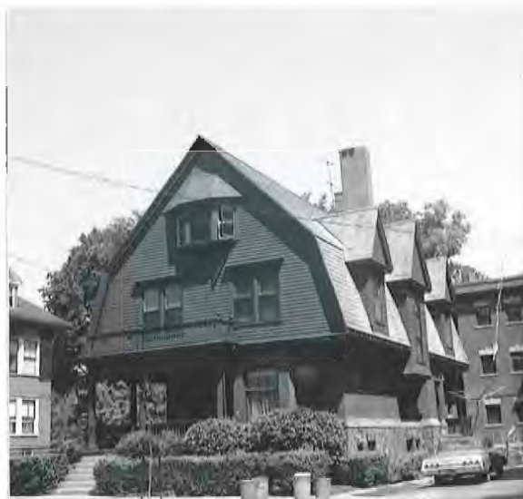
Architect Frederick Tompson designed and built his own Shingle style residence at 33 Carroll Street in 1901. Characterized by a gambrel roof, deep dormers, shadowy porch cut out of the main block of the building and a variety of materials including brick, shingle, and stone, this landmark quality is similar in scale, mass, setback and materials to its compatible but less architecturally distinguished neighbors.
