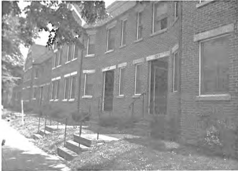
The ratio of width to height of the projecting and recessed portions of this facade are carefully related to each other and to the width and height of neighboring houses in the West End.
