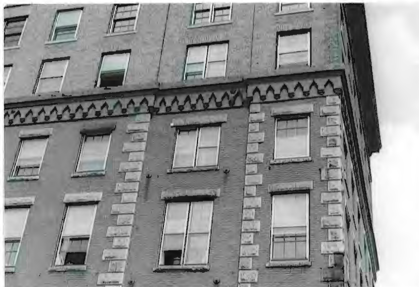
William Moulton Block, 165-169 Commercial Street. Two years later Moulton had the neighboring building, partially visible in upper photograph, built (the three upper floors are a later addition). This builder added quoins and a corbelled cornice, architectural features of the Italianate style. In both buildings the first floor is set off by a heavy granite cornice and granite piers. This delineation of the first floor unifies the buildings in the waterfront district.
