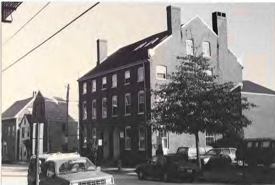
The Joseph How House, 30-32 Pleasant Street, built in 1818 by Daniel's brother as a two family structure. The tradition of constructing duplexes was to continue throughout the nineteenth century in Portland. Like the other two How Houses, this structure has four chimneys on outside walls, but the window tops are elliptical and the elevation is three and one-half storeys. This enclave of late Federal red brick dwellings is coherent in general form in material and in details.
