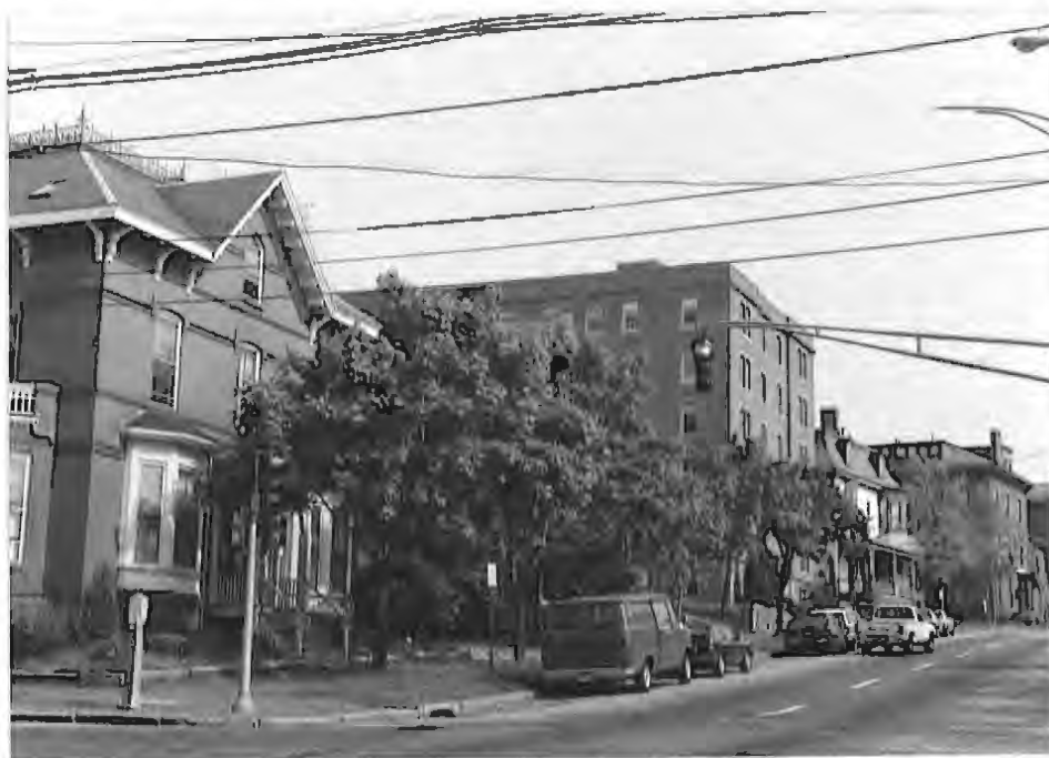
State Street features the most diverse collection of building types and styles in the district. Here one finds early 20th century apartment buildings, duplexes and single family residences. Architectural styles range from Victorian Gothic to Italianate to Colonial Revival. With few exceptions, buildings face State Street, rather than the intersecting streets. Again, the relative uniformity of scale and the sophistication of the architecture itself serve to unify the street. As this corridor is a key gateway into the inner city, changes should be carefully considered.
