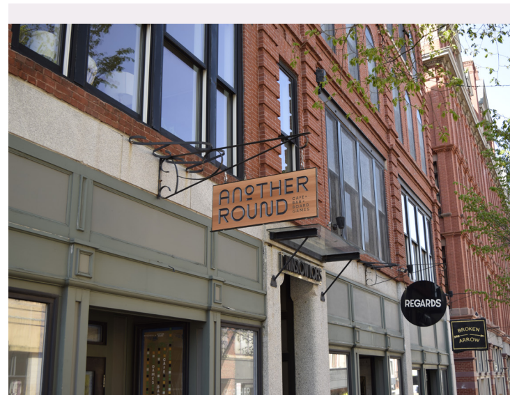
At 549 Congress Street (1880) durable brackets were installed that can hold a variety of sign types as the commercial tenants change over time. This approach minimizes damage to the historic masonry by only requiring replacement of the sign panel.
