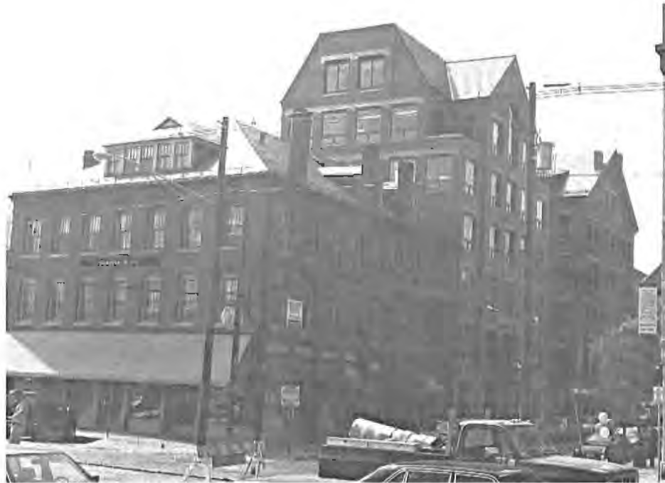
Ten Moulton Street illustrates how the height of infill construction can serve as a bridge between the heights of surrounding structures. While the infill building is taller than its immediate neighbor on Commercial Street, it is roughly the same height as the adjacent building that fronts on Fore Street. The roof also contributes to the impression of proper scale relative to its neighbors by echoing the dormer shape of the building in the foreground and the gable shape of the building behind it. Details, such as the cut-out balconies, also help to reduce its apparent height, especially from the street.
