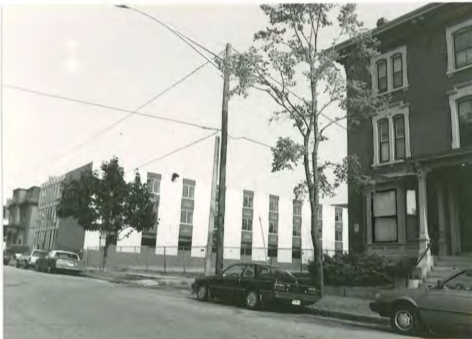
Few intrusions are present in the Deering Street Historic District. Any new construction in this district should respect the prevailing qualities of the existing buildings to avoid the jarring effect created by the former hotel annex. Here, while the height and scale is similar to that of its neighbors, the flatness of the facade and the lack of ornamentation makes this a poor solution for its infill site.
