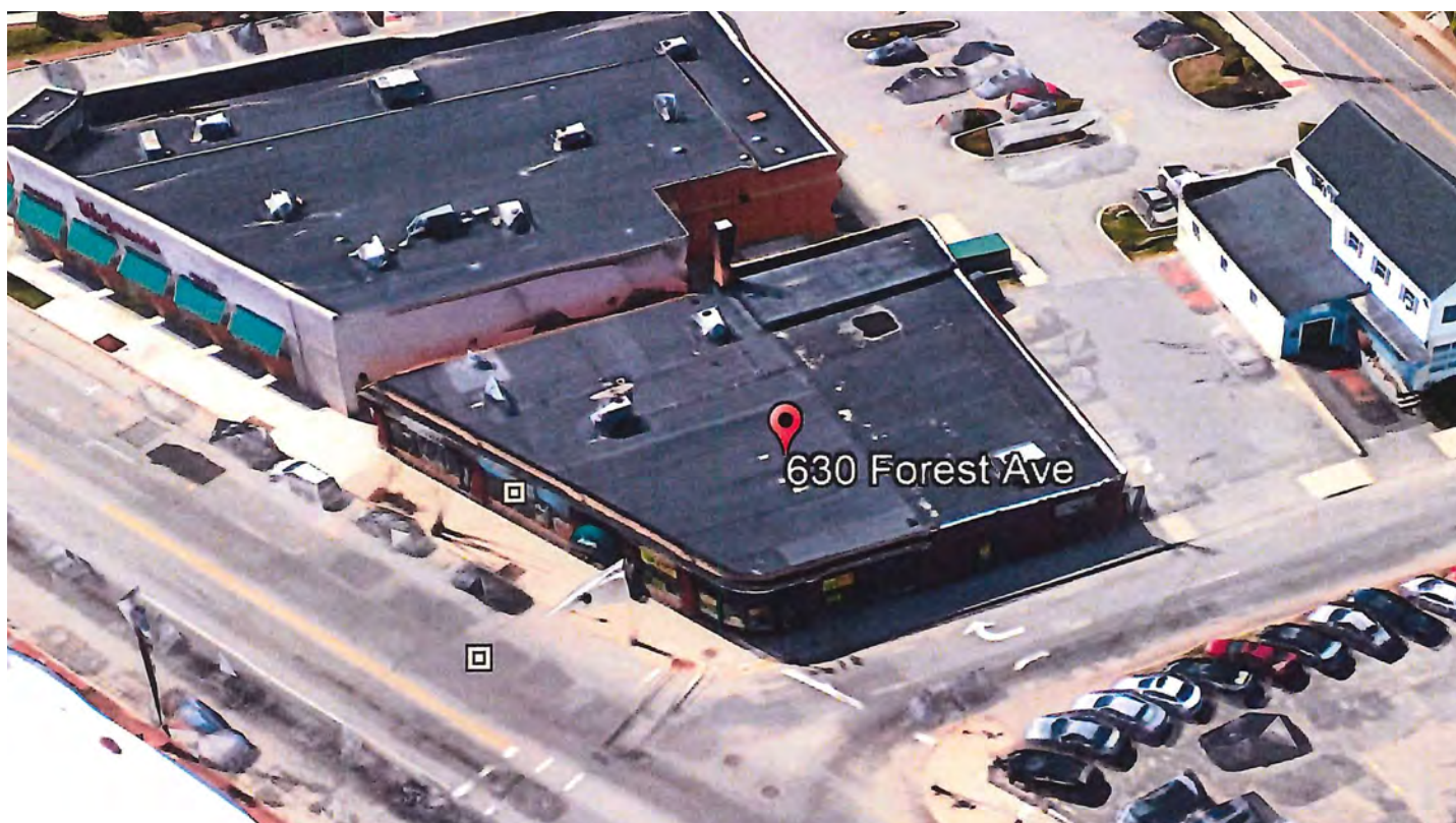
Aerial view showing footprint of later addition
