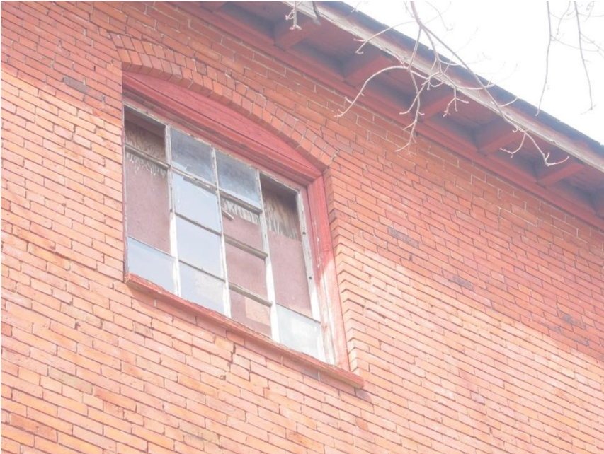
Original brick opening for third story window. Molding under oversailing rafters and eave boarding with 3" deck and slate projection. Fixed sash with sixteen panes. Brick bonding with headers eight courses apart.
