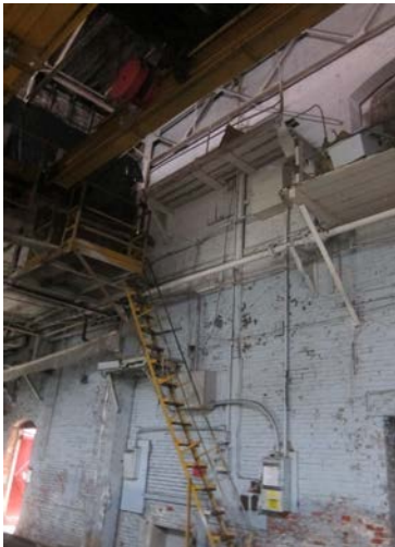
Building 4 bay & Building 3 east
