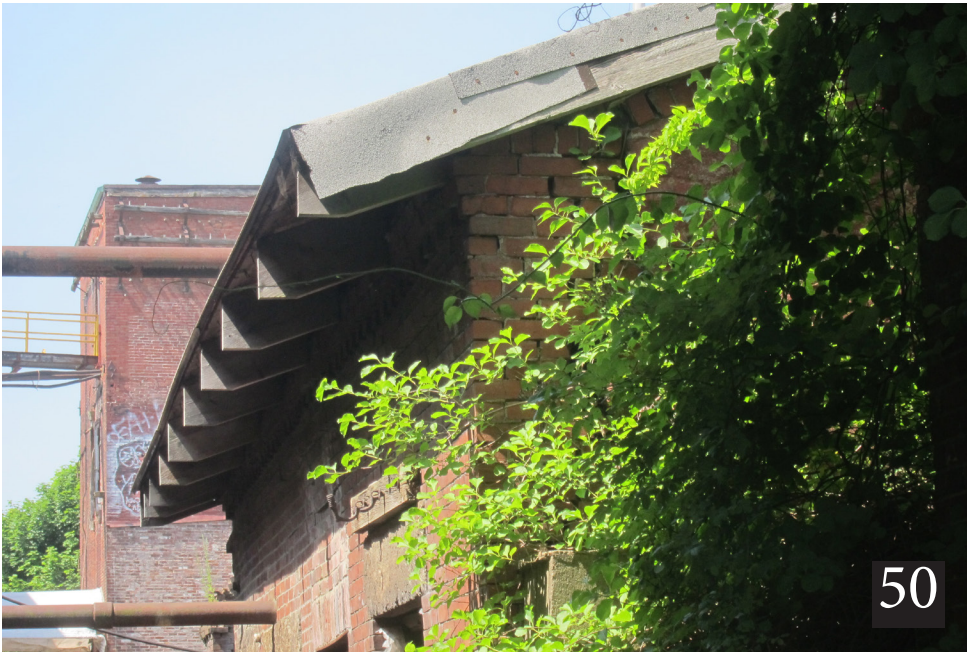
50. Roof rafters oversail the main façade of Building 16 and may be retained. Fascia boards will be reinstated.
