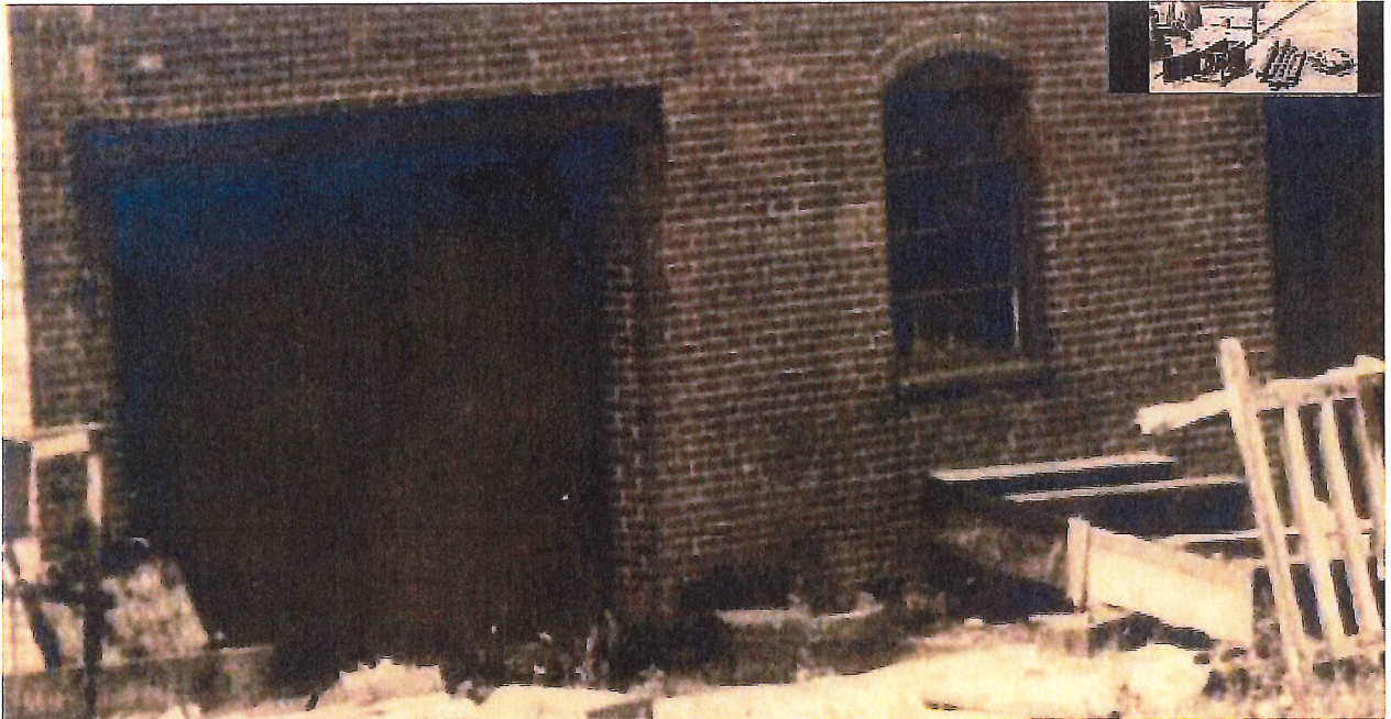
Building #12 – “Garage Door” and Existing Window at Grade - Excerpted from source image above
