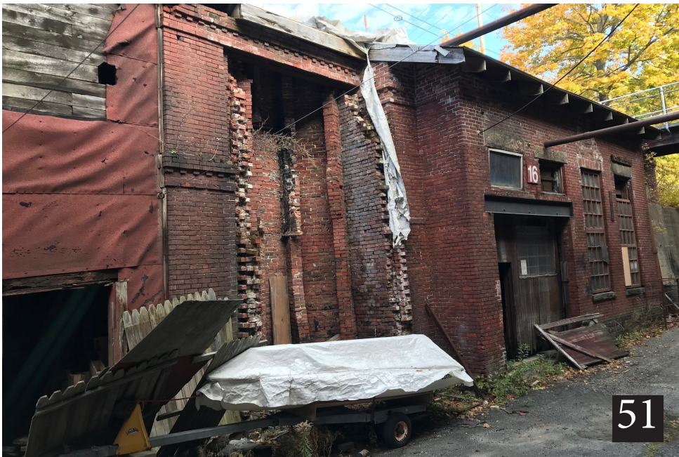
51. Overall façade image from the east pier of Building 15 through the chimney base remnant and Building 16 facade that projects into the narrow alley.
