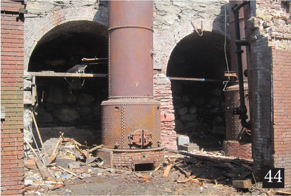
44. Original boilers and tank room at coal vaults. Central pier (left of photo) collapsed and removed. Current planning studies include feasibility of retaining one boiler when space is converted to retail/dining behind new glazed façade along the Narrow Alley.
