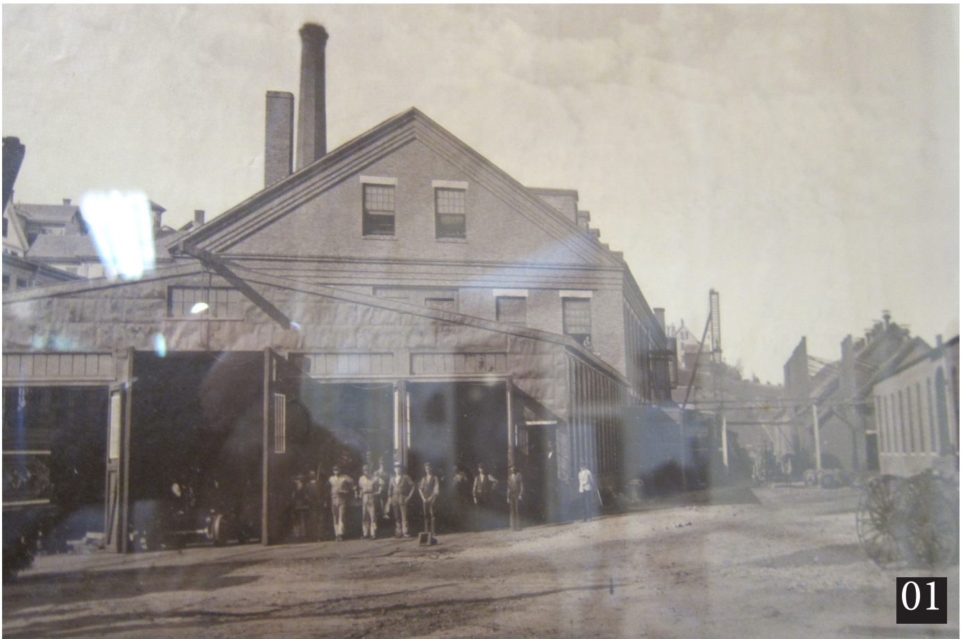
01. Early view of Building 2 west façade with Building 16 chimney in background and north wall of Building 6B. Granite cobbles on site surface. Final brick erecting shed, Building 1, Building 6A, and bridge all yet to be built.
