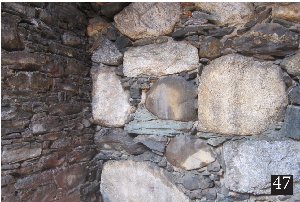
47. Fieldstone buttress wall abuts the massive, coarse stonework of the sea wall. The design intent is to allow views of these material surfaces through the glazed façade of Building 15.
