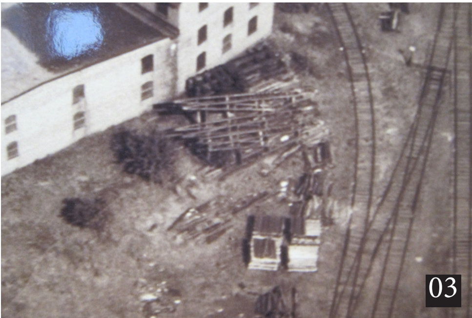
03. Industrial site condition at pattern storehouses, Building 11 and Building 12 showing stacked materials, rough landscape, and rail lines.
