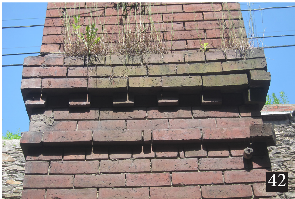
42. Brick entablature detail in the piers of Building 15 continues across the party wall of Building 16.
