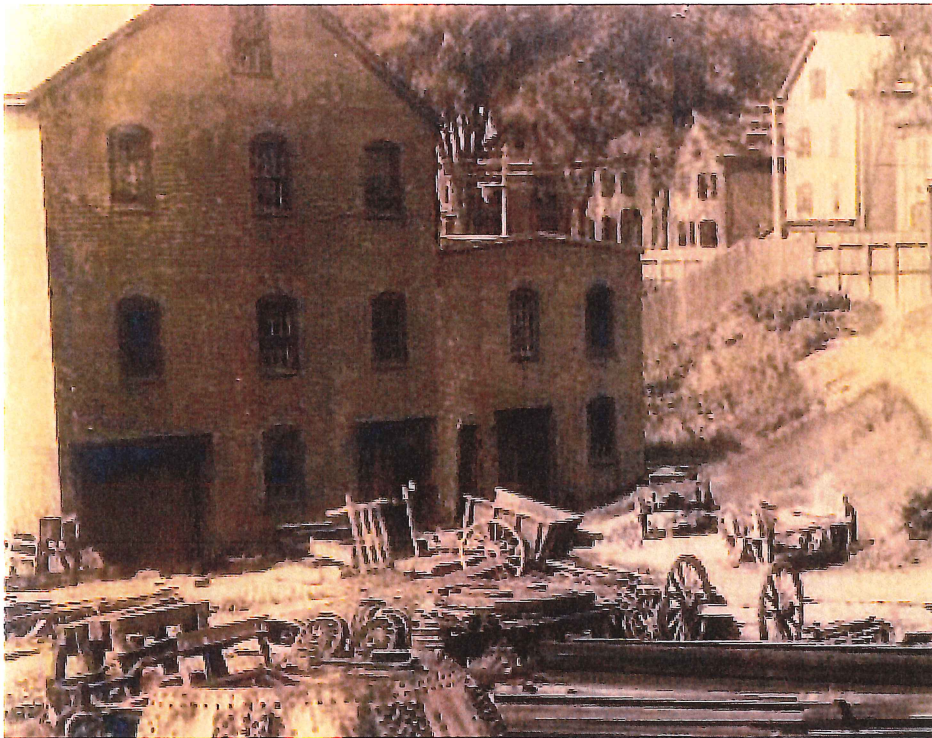
Building #12 Excerpted from source image above
