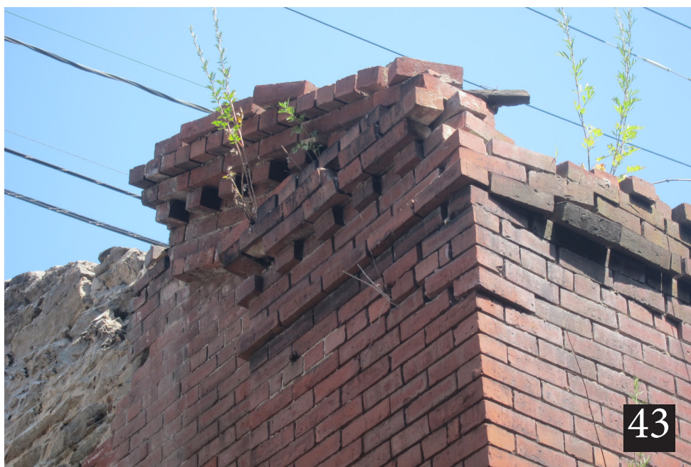
43. Brick entablature and cornice detail of Building 15 marks the original roof slope. Existing fragment will be reconstructed.
