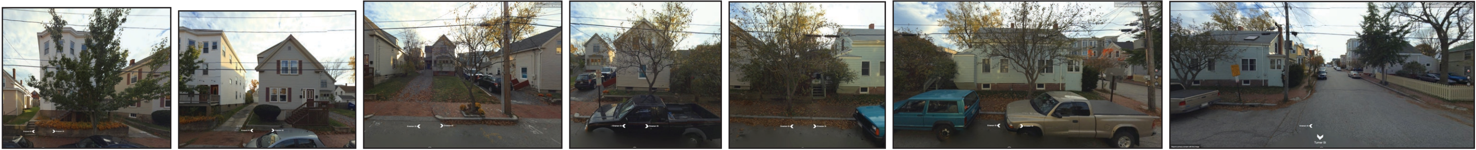
16 Emerson 20 Emerson 22 Emerson 24 Emerson 38 Turner Turner Street
