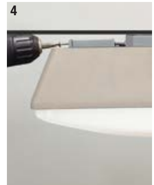
4 Two mounting screws close and secure fixture to the mounting bracket.
