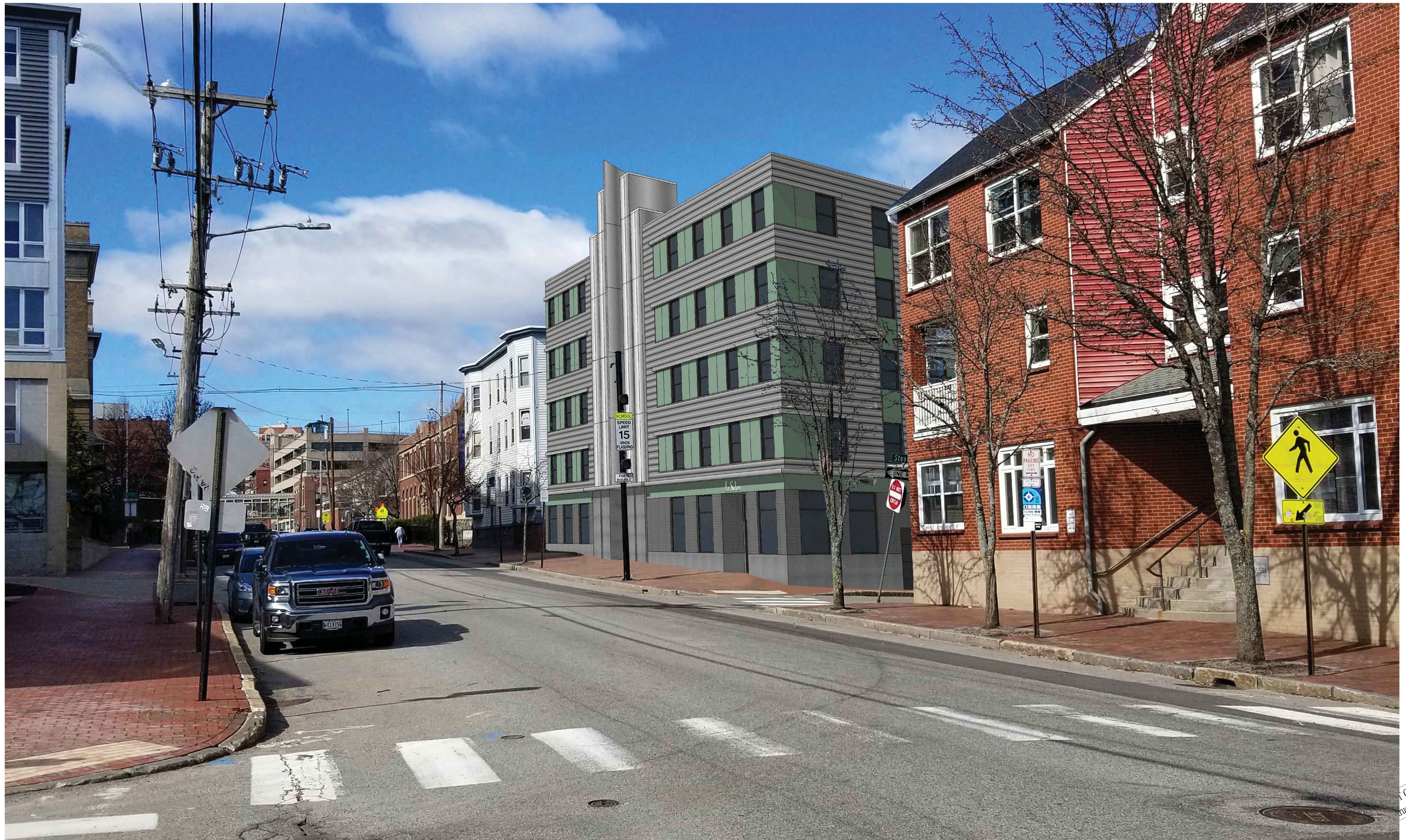
1 VIEW LOOKING WEST ON CUMBERLAND AVE
