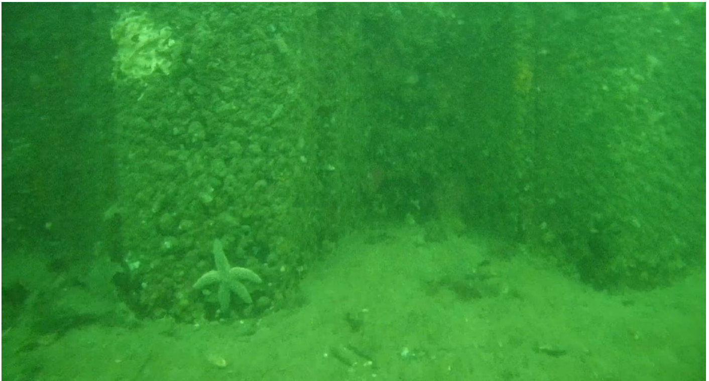
Picture #20 Underwater Drone Photo of Typical Sheet Pile at Mudline
