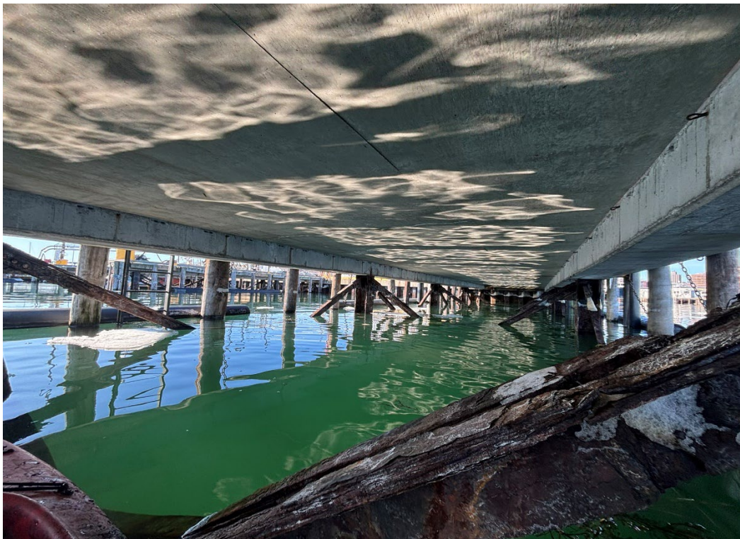
Picture #4 Looking South at Service Pier #1
