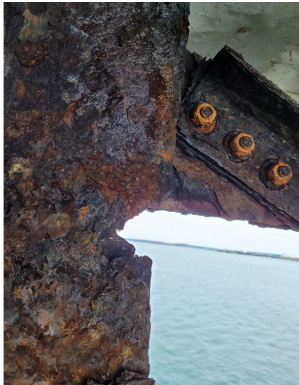
Picture #15 Service Pier #1 Bent 5, Pile 2
