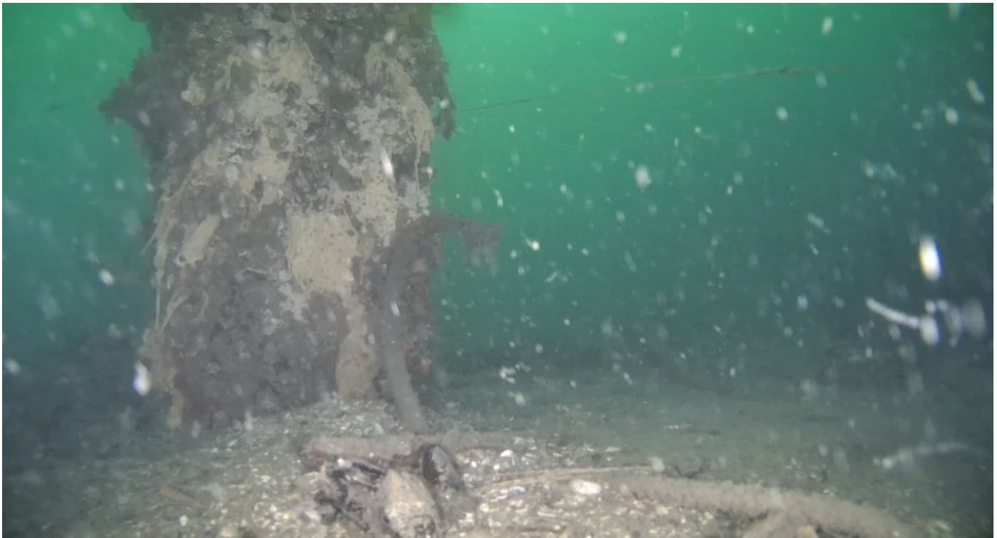
Picture #19 Underwater Drone Photo of Typical H-Pile at Mudline
