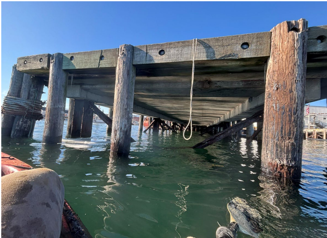
Picture #3 Looking South at Service Pier #3
