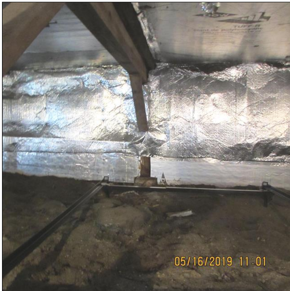
6.0 Item 7(Picture) Crawlspace
