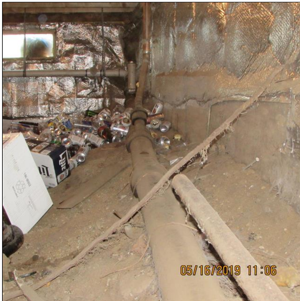
6.0 Item 13(Picture) Crawlspace
