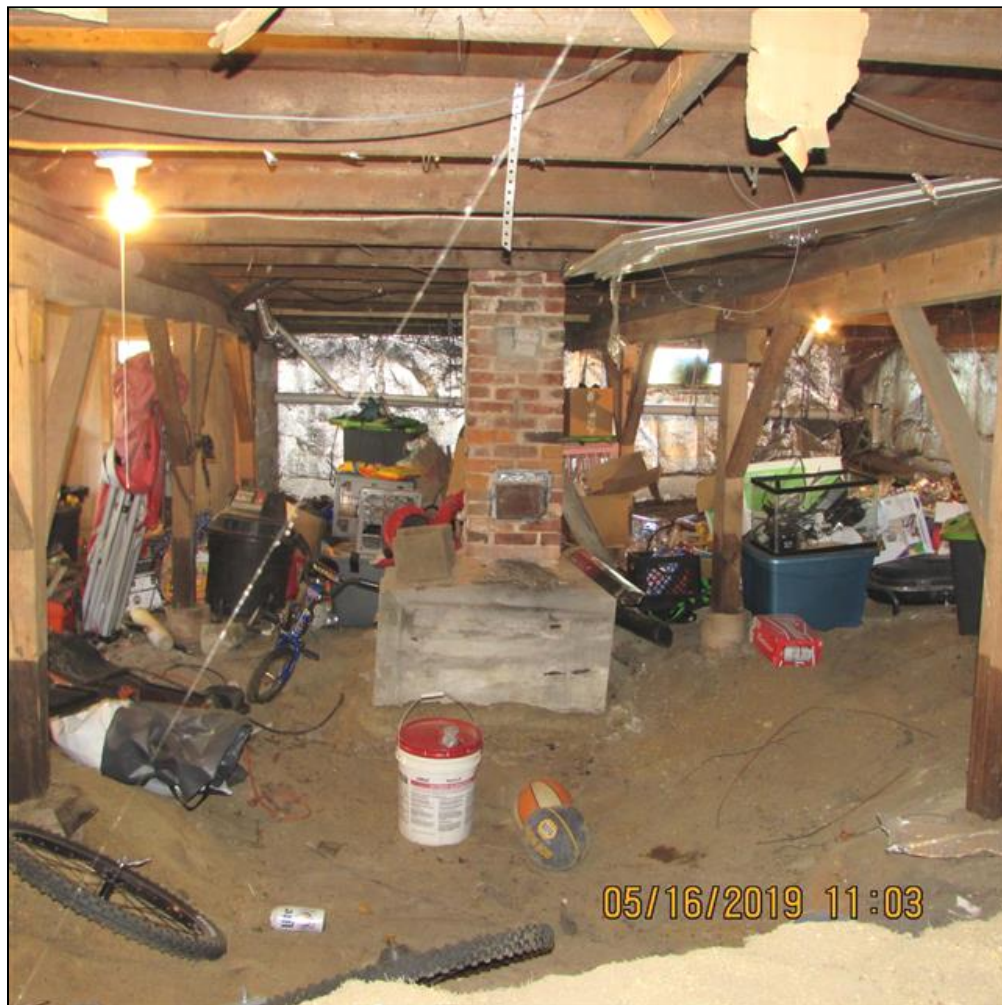
6.0 Item 10(Picture) Crawlspace
