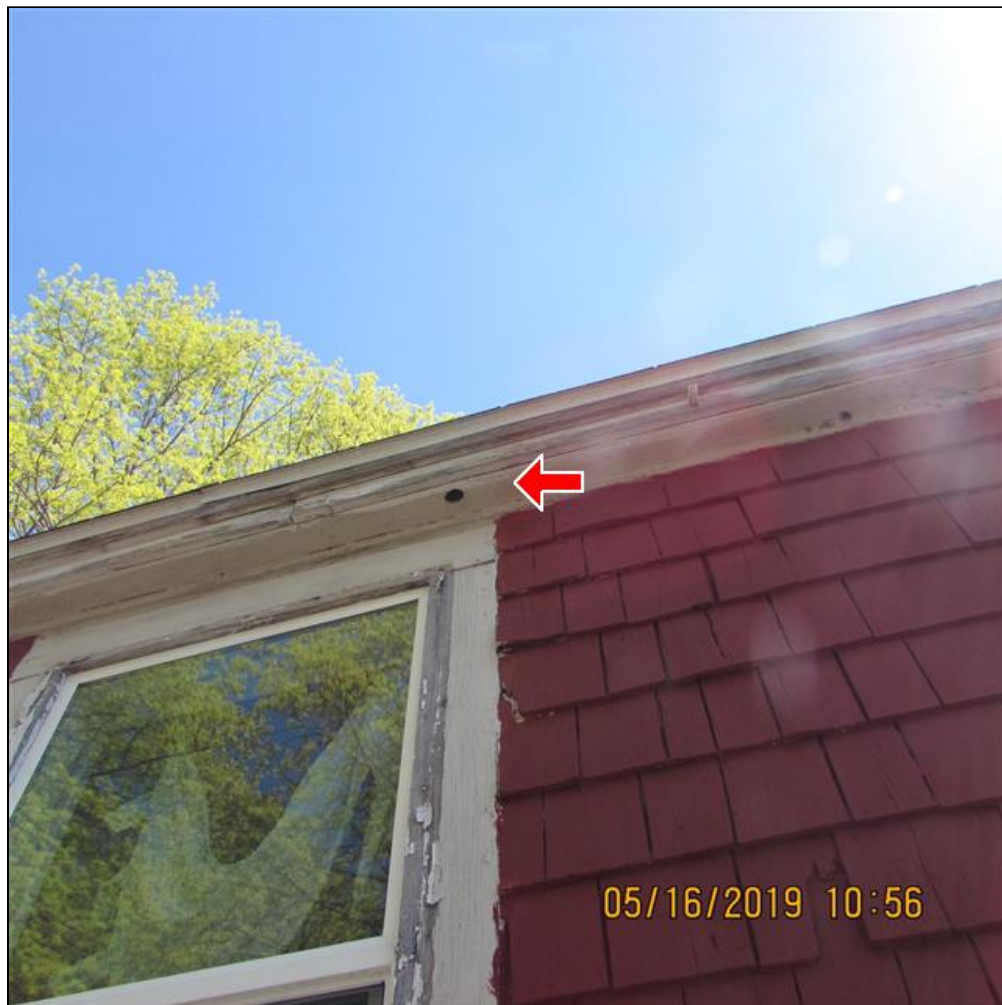
2.1 Item 3(Picture) Seal holes in soffits
