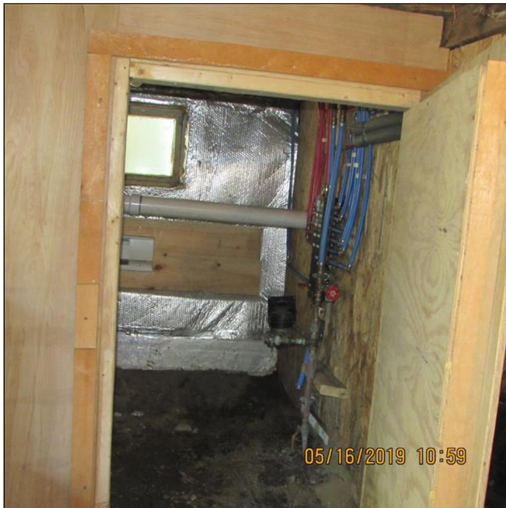
6.0 Item 6(Picture) Crawlspace
