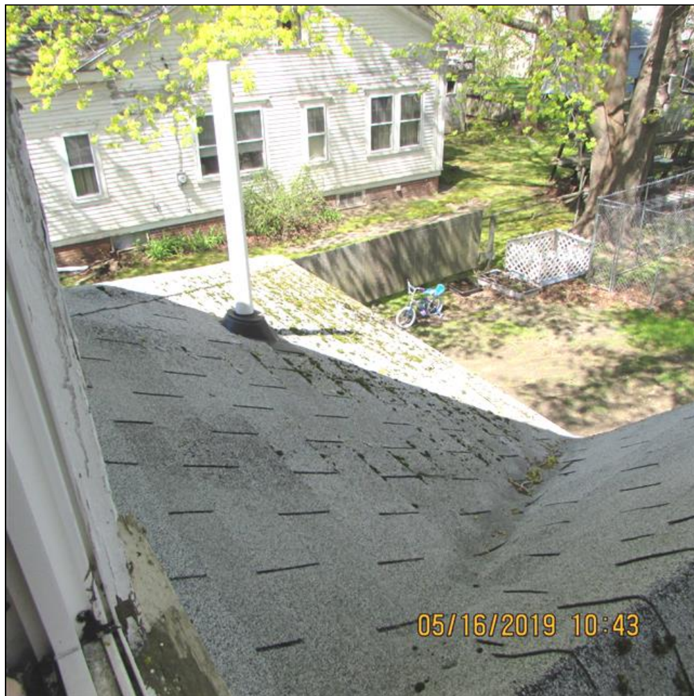
1.0 Item 2(Picture) Roofing
