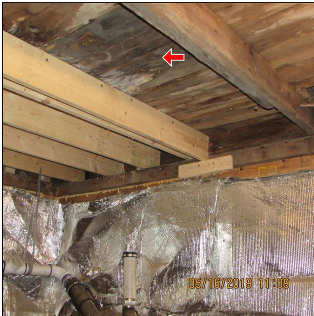
6.3 Item 1(Picture) Monitor sub flooring below bathrooms and kitchens
