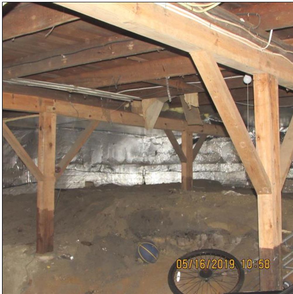
6.0 Item 2(Picture) Crawlspace
