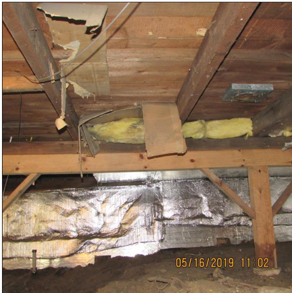
6.0 Item 8(Picture) Crawlspace
