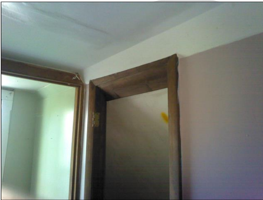
13.0 Item 13(Picture) 2nd floor without thermal image
