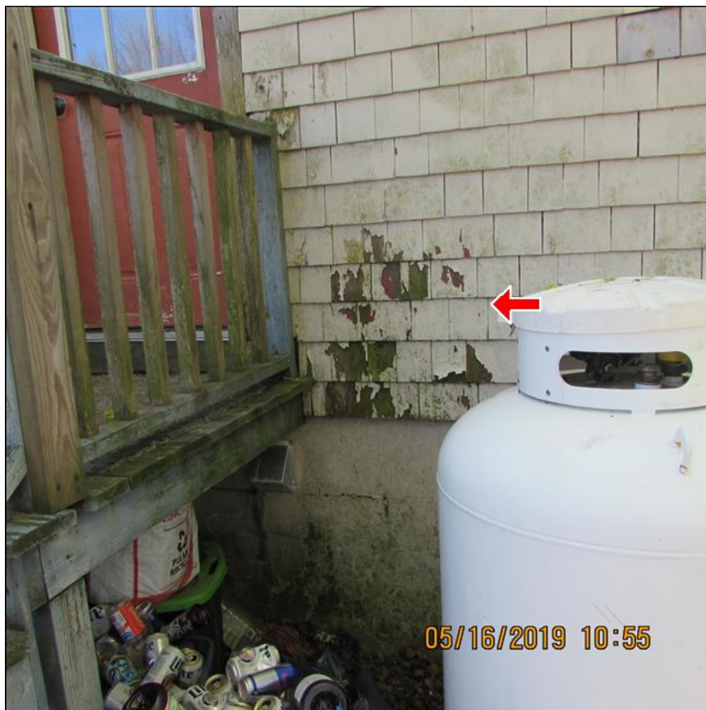
2.0 Item 5(Picture) Paint siding where needed
