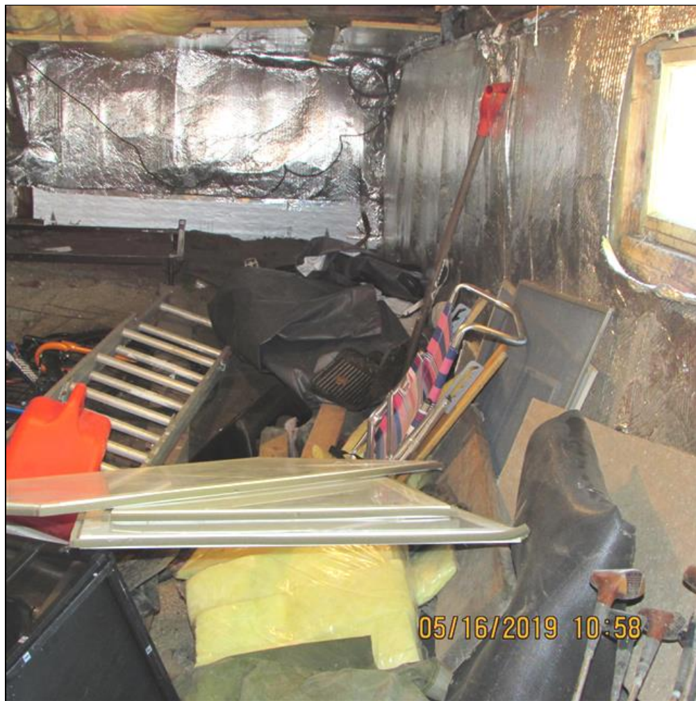
6.0 Item 1(Picture) Crawlspace
