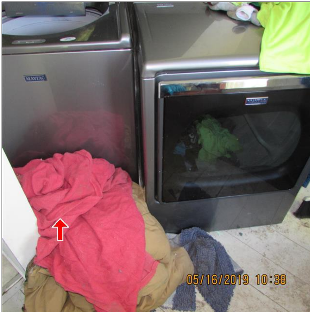
3.7 Item 1(Picture) Drip pan recommended under the washer
