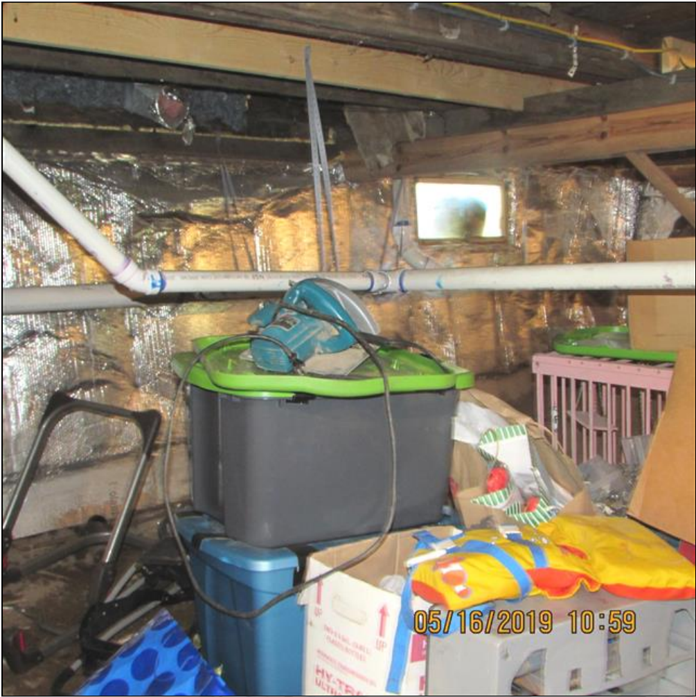
6.0 Item 5(Picture) Crawlspace
