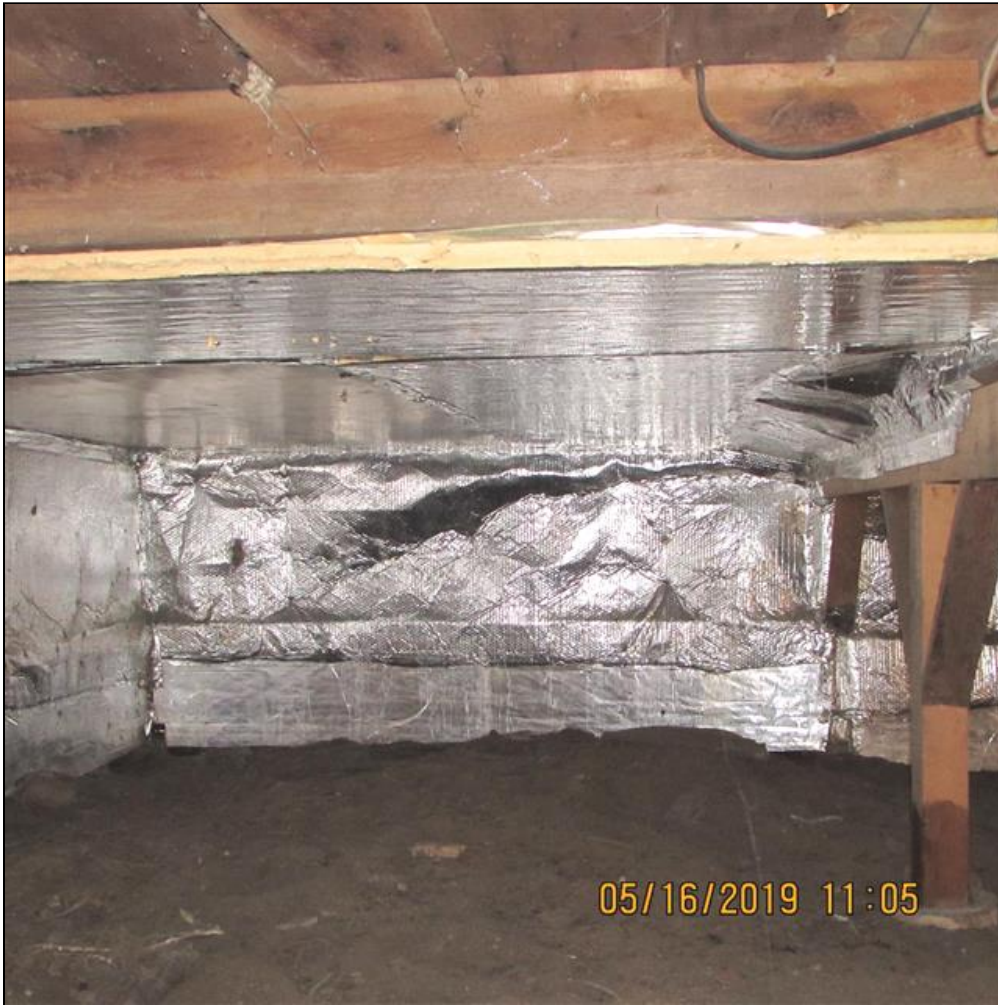
6.0 Item 12(Picture) Crawlspace
