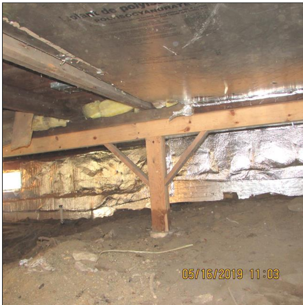
6.0 Item 9(Picture) Crawlspace
