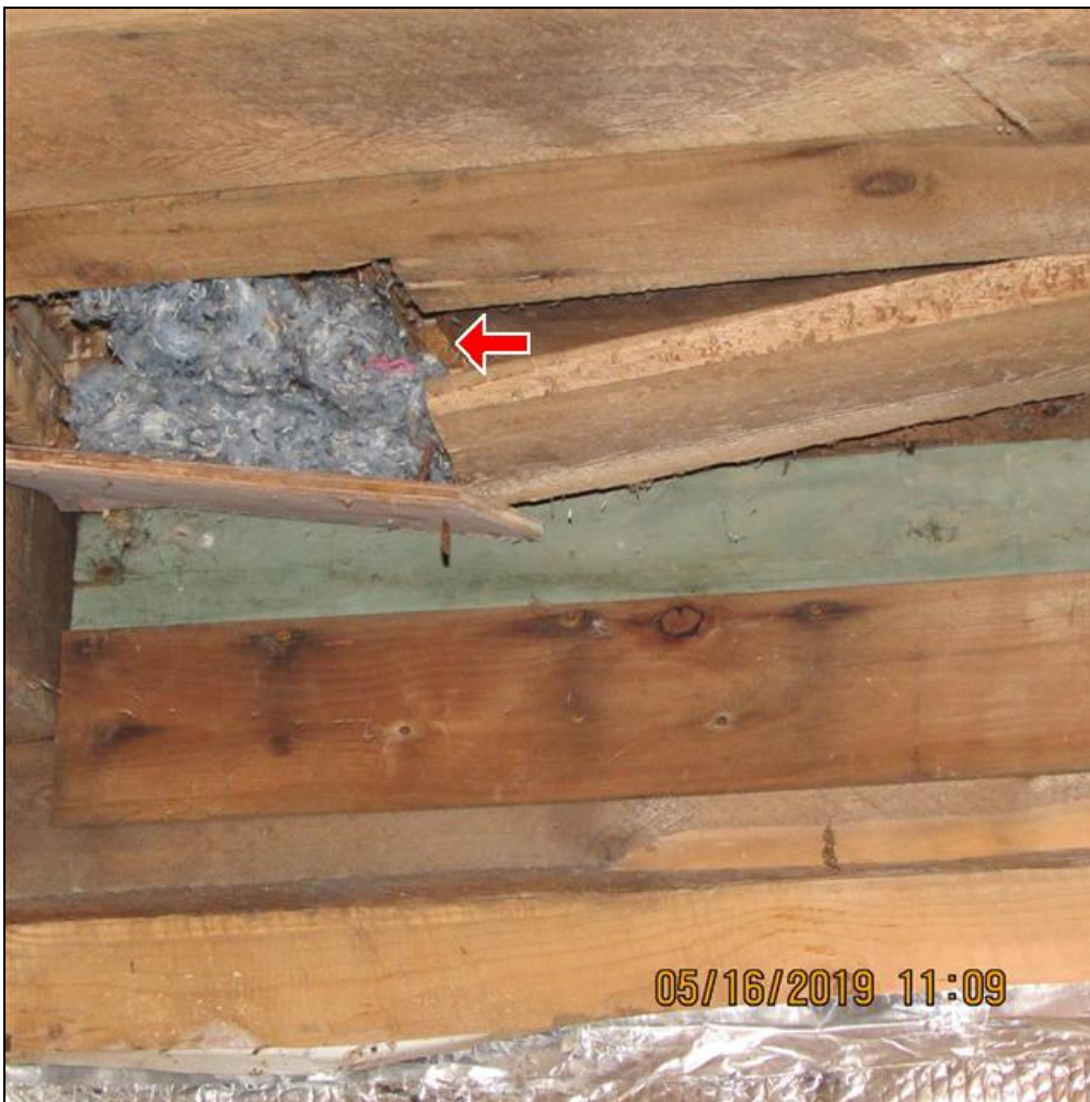
11.2 Item 1(Picture) Mouse nest in crawlspace
