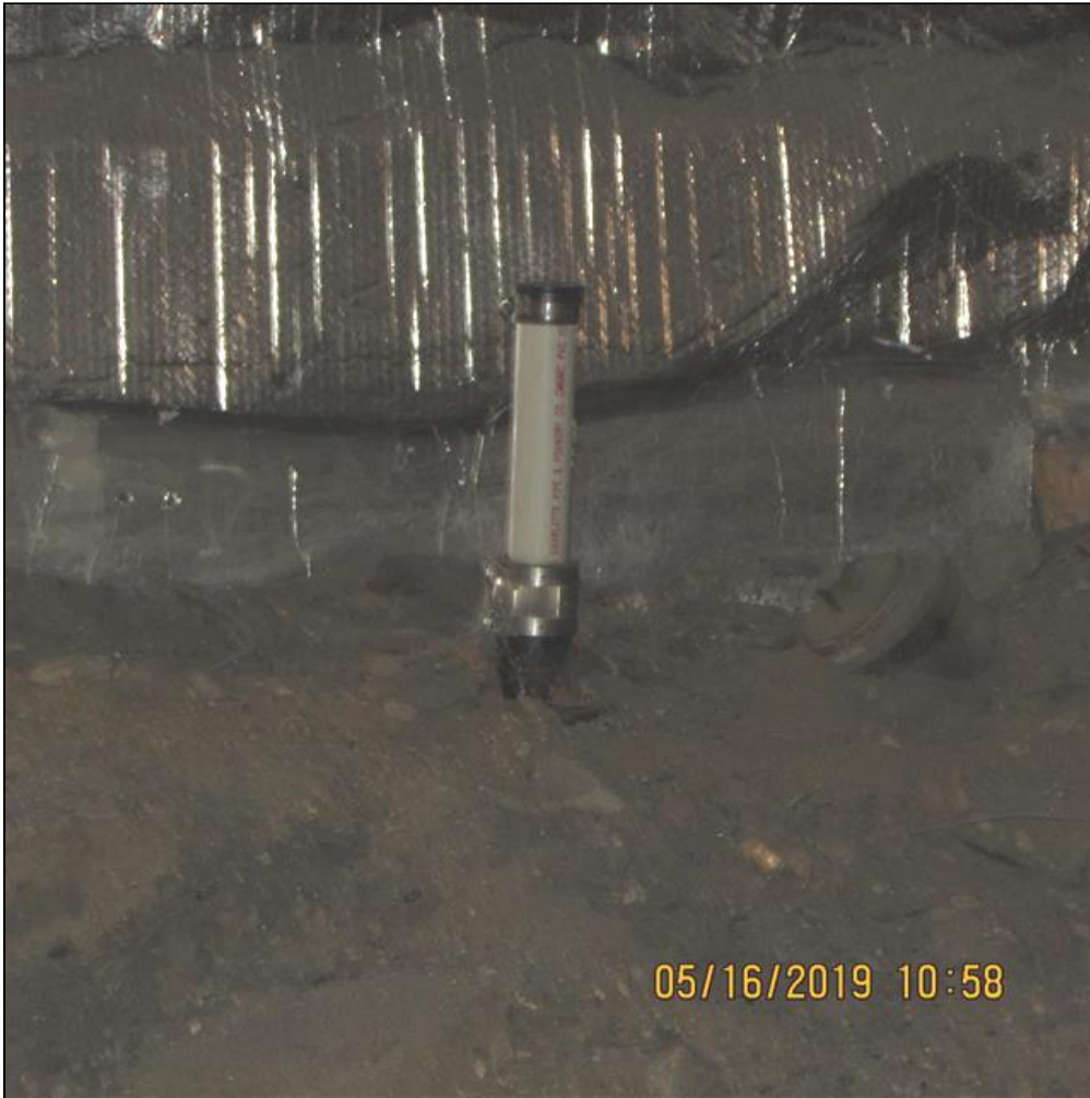
6.0 Item 3(Picture) Crawlspace
