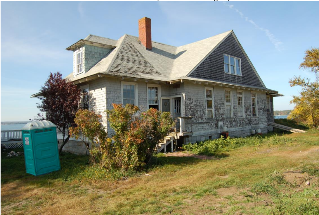
The small Detention Barracks – Before and After (known as Building #1)
