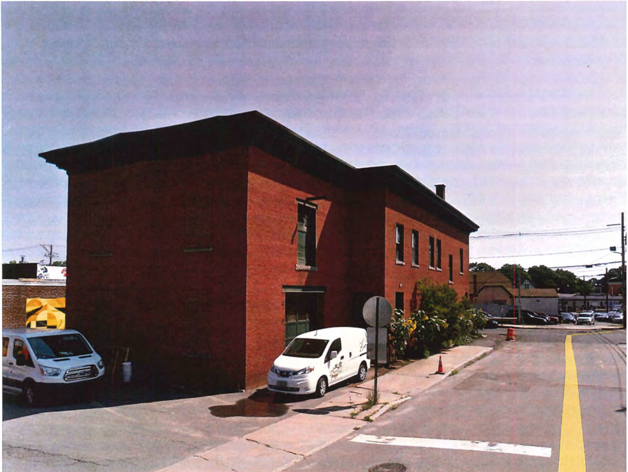
View of building from Revere Street
