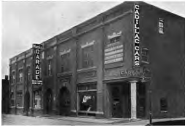
Service Station of Miles B. Mank Motor Car Co., Portland, Me.
