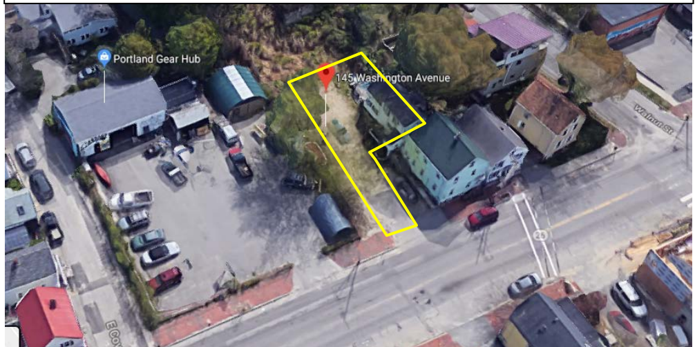
Fig. 1: Aerial View of the Subject Property (before the demo of the single-family home as the rear side)
