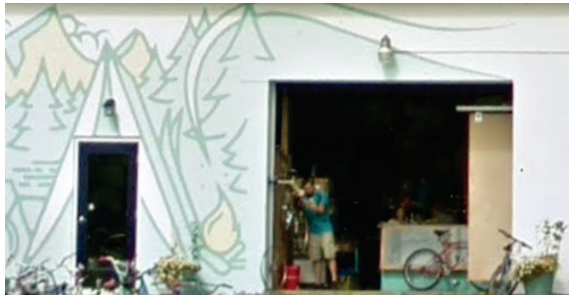
Commercial 155 Washington Ave.
