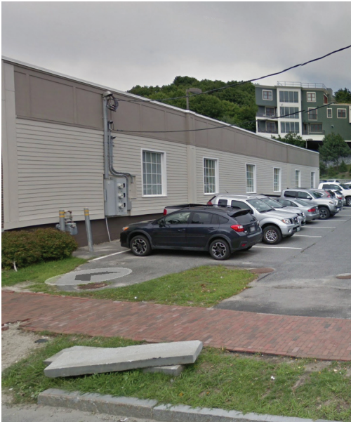
Commercial 107 Washington Ave.
