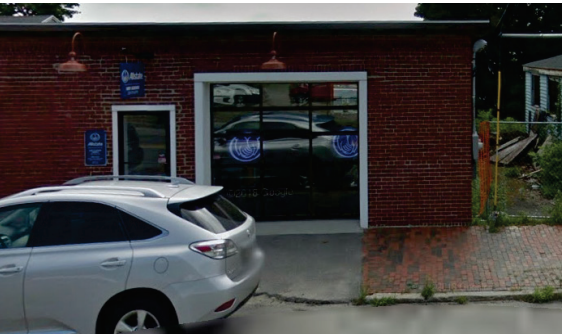
Commercial 178 Washington Ave.
