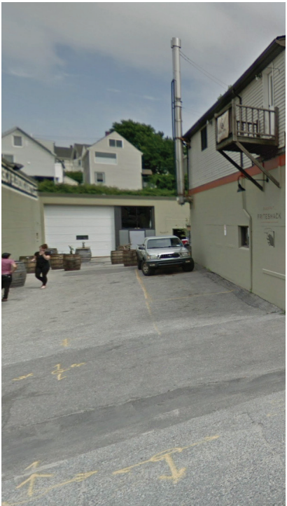
Commercial 43 Washington Ave.
