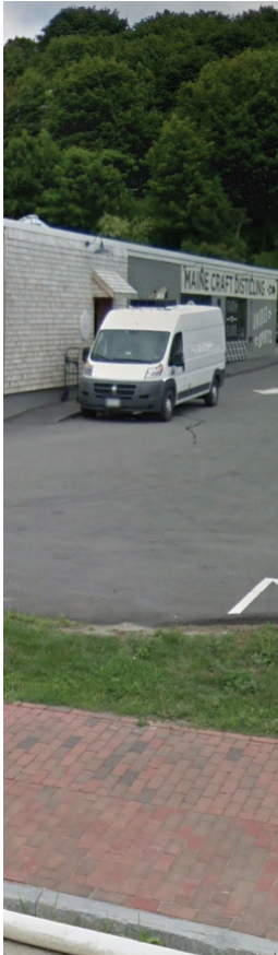
Commercial 123 Washington Ave.
