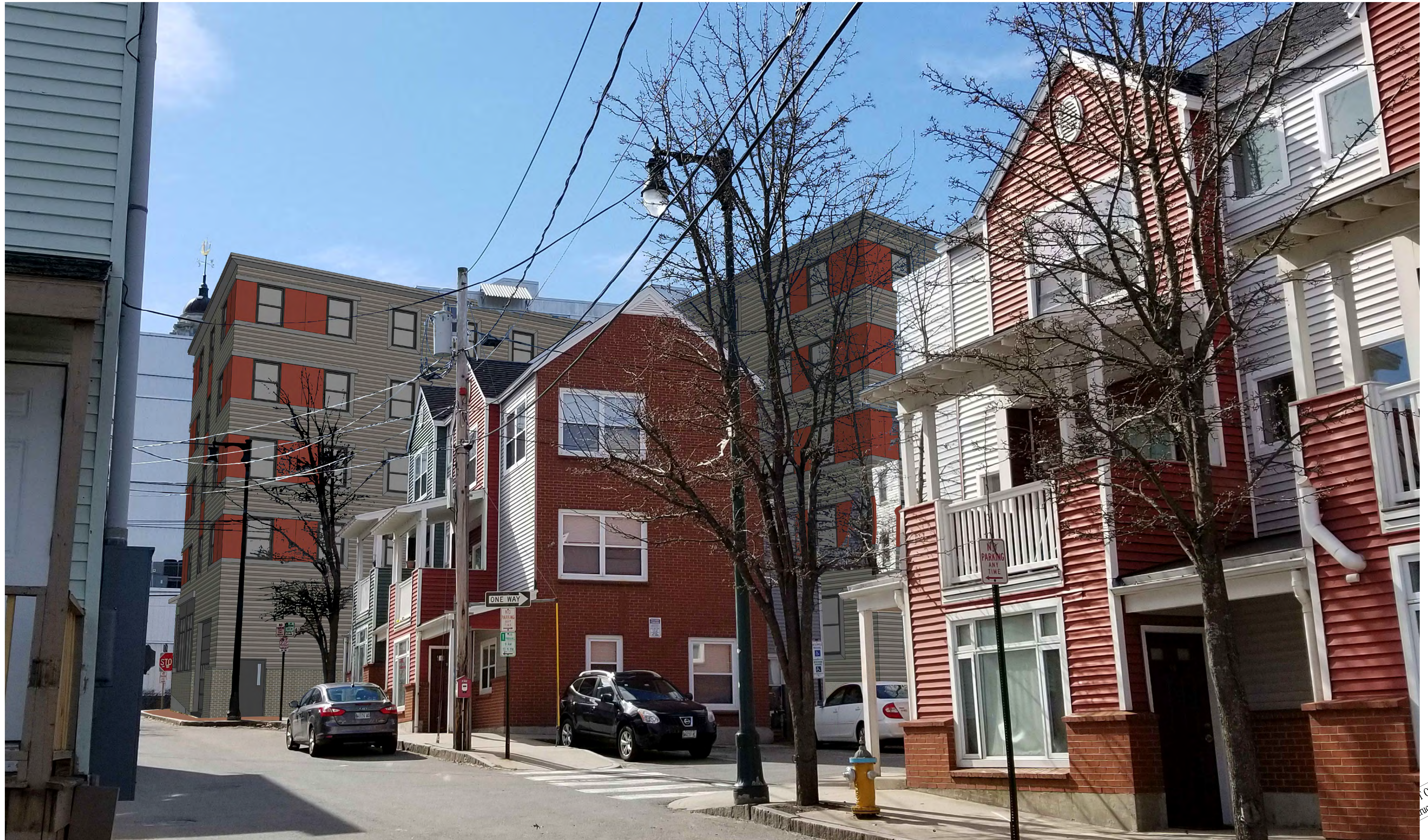
1 VIEW LOOKING SOUTH ON STONE STREET
