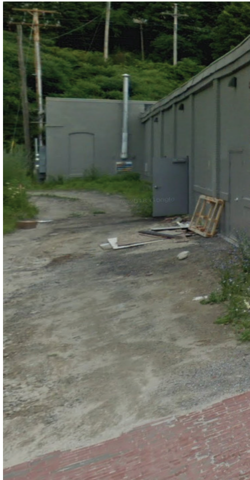
Commercial 123 Washington Ave.
