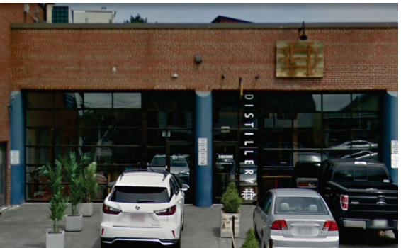
Commercial 53 Washington Ave.
