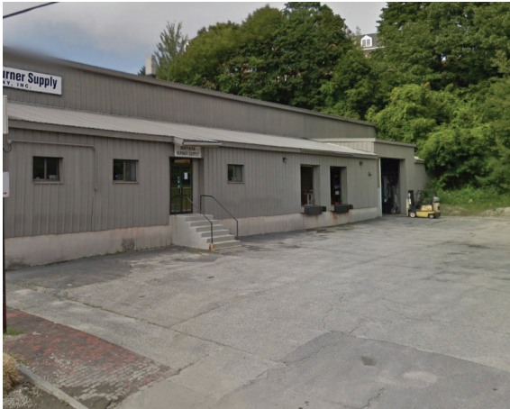
Commercial 185 Washington Ave.
