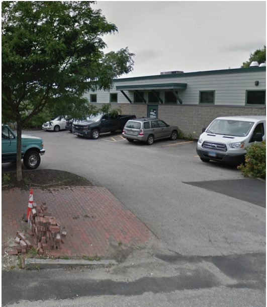
Commercial 94 Washington Ave.
