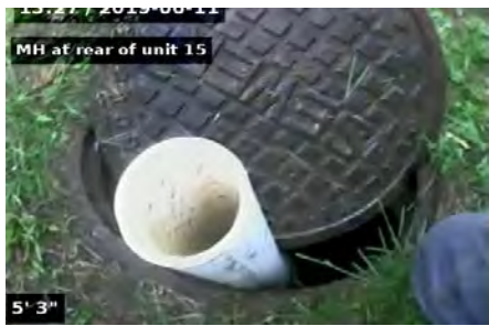
entrance to sewer mahole 1
