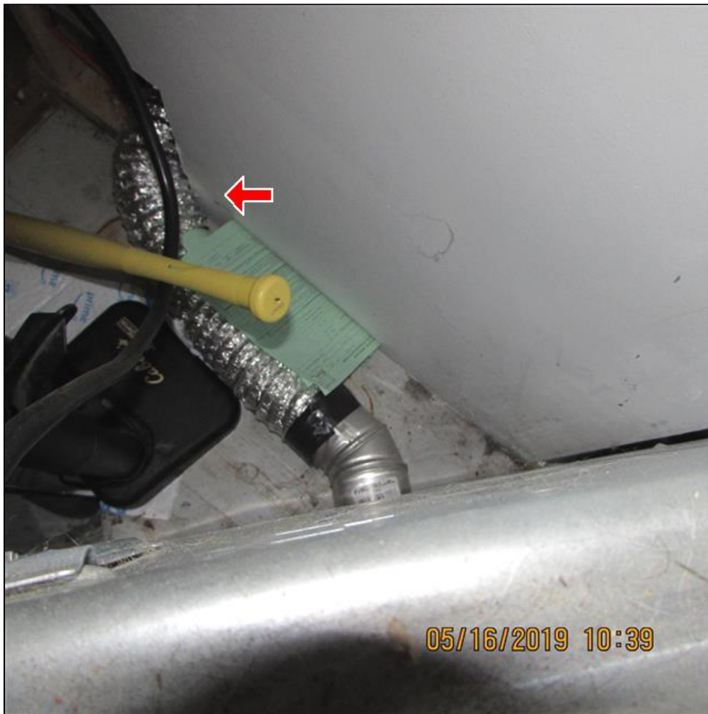
10.5 Item 1(Picture) Replace dryer duct
