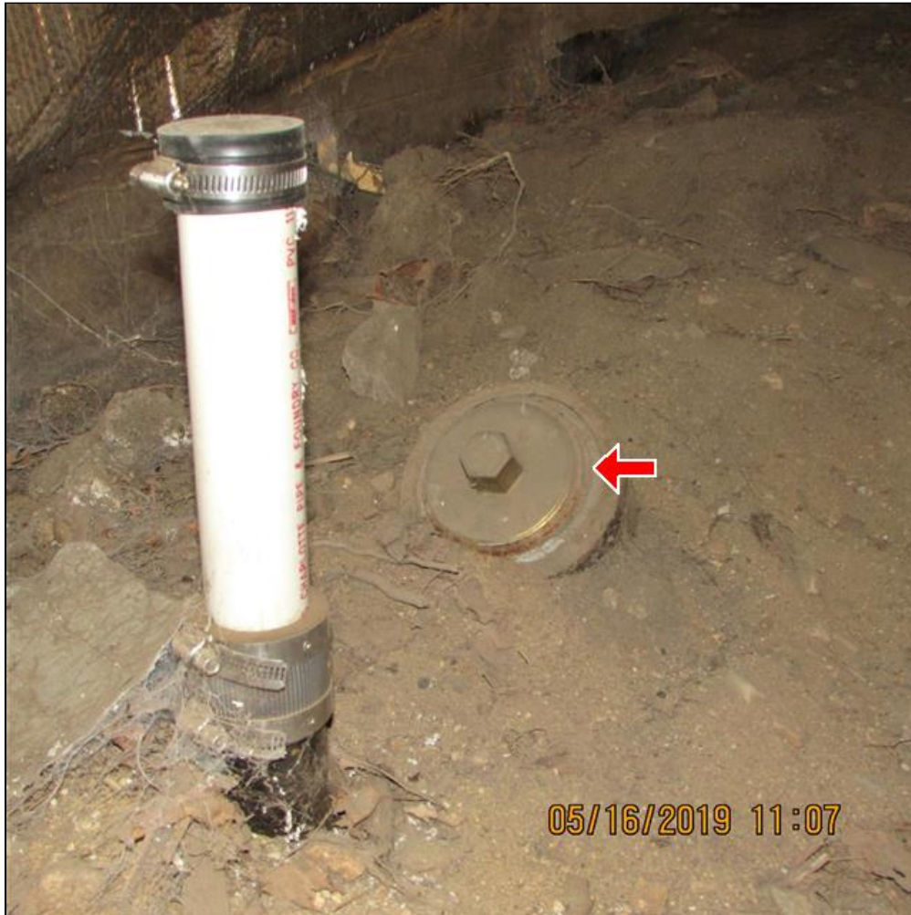
8.1 Item 1(Picture) Waste line access in crawlspace
