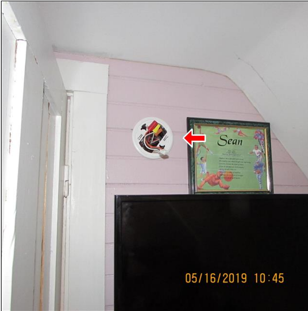
9.7 Item 2(Picture) 2nd floor missing smoke detector
