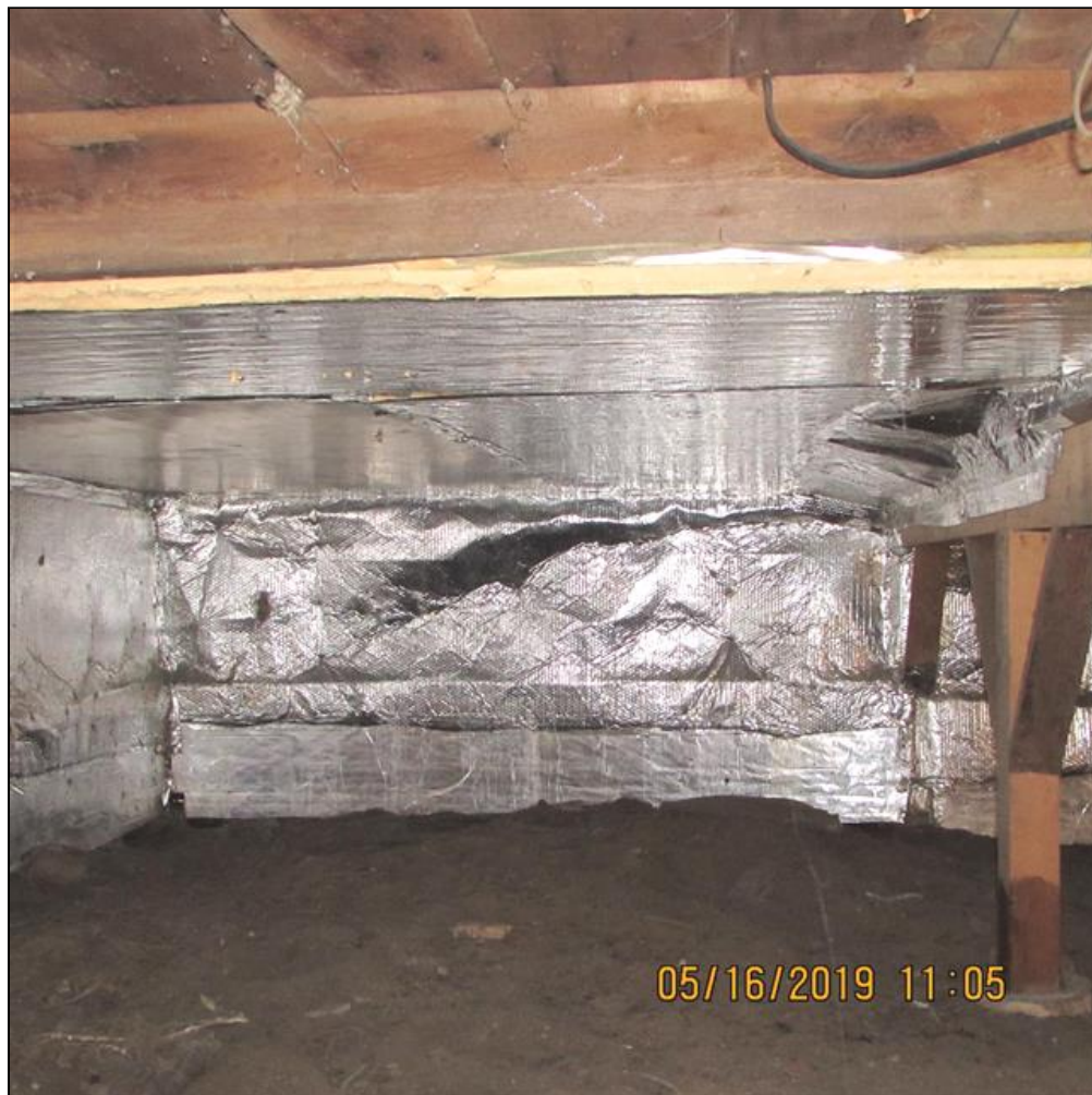
6.0 Item 12(Picture) Crawlspace
