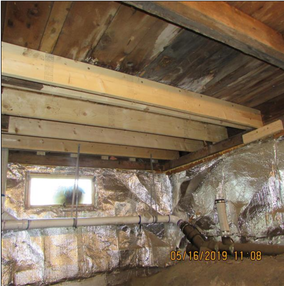
6.0 Item 14(Picture) Crawlspace
