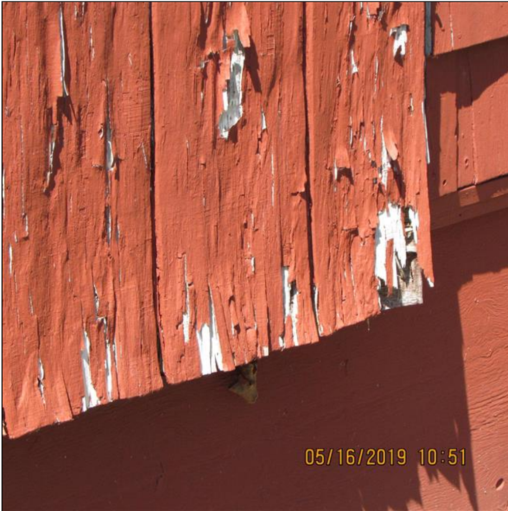
2.0 Item 3(Picture) Closer view
