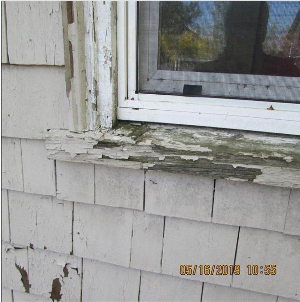
2.3 Item 4(Picture) Rear window
