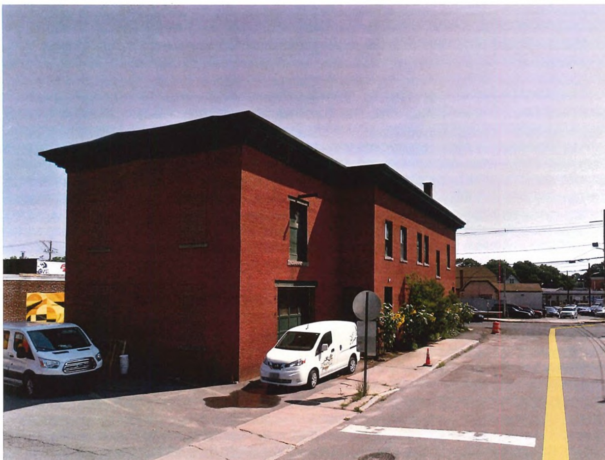
View of building from Revere Street
