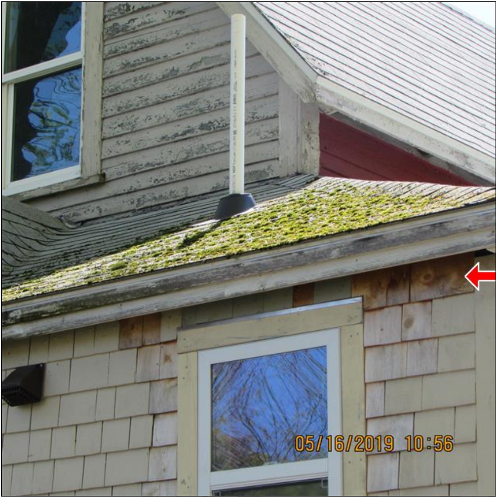
2.0 Item 6(Picture) Keep siding painted
