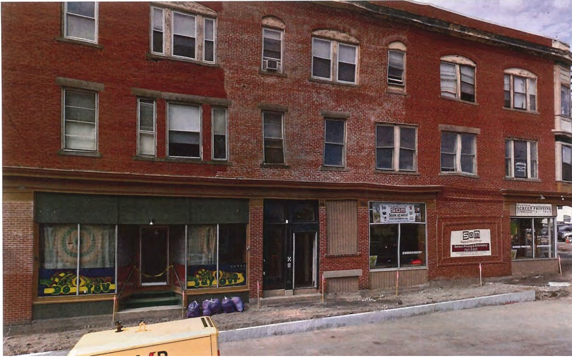
Forest Avenue elevation of Chapman Block
