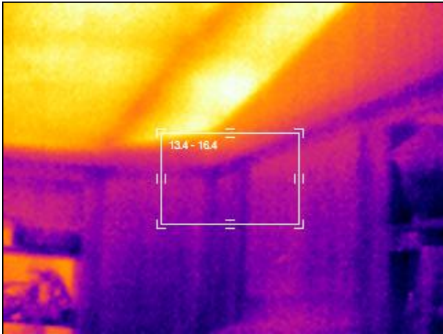
13.0 Item 16(Picture) Kitchen ceiling showing lack of insulation
