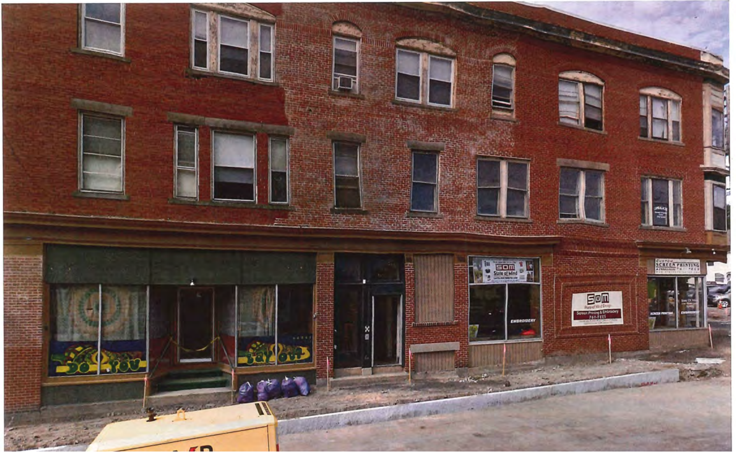
Forest Avenue elevation of Chapman Block
