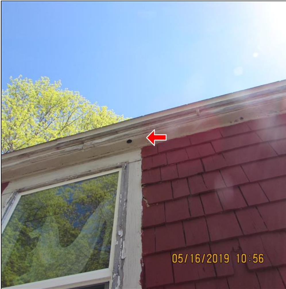
2.1 Item 3(Picture) Seal holes in soffits
