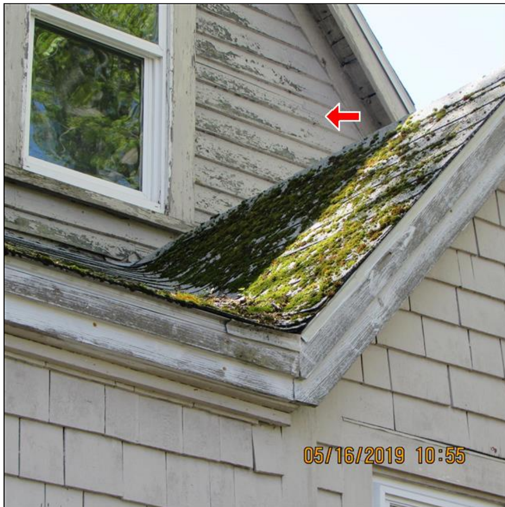
2.0 Item 4(Picture) Keep siding painted
