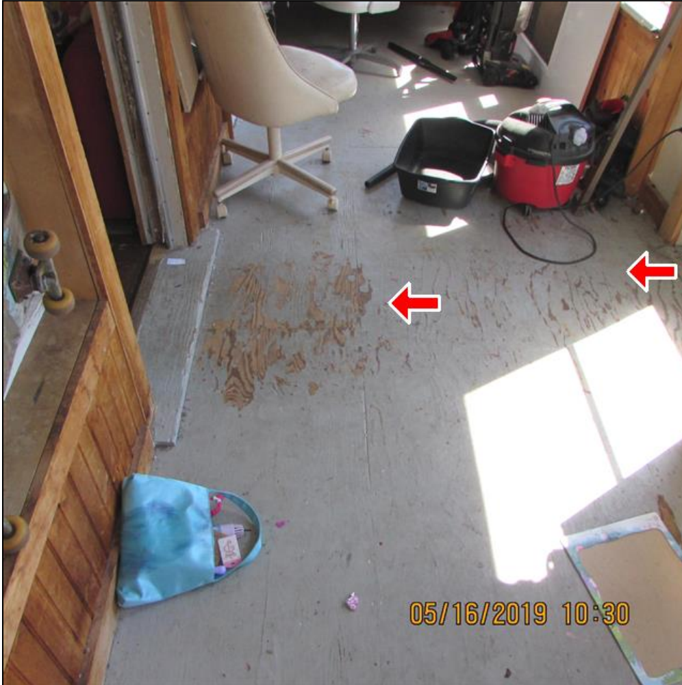
4.2 Item 1(Picture) Front porch floor
