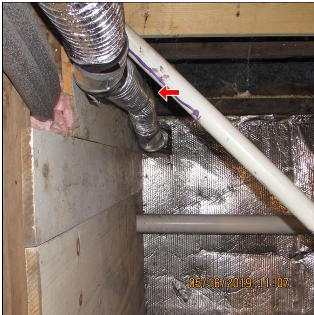
10.5 Item 3(Picture) Replace dryer duct
