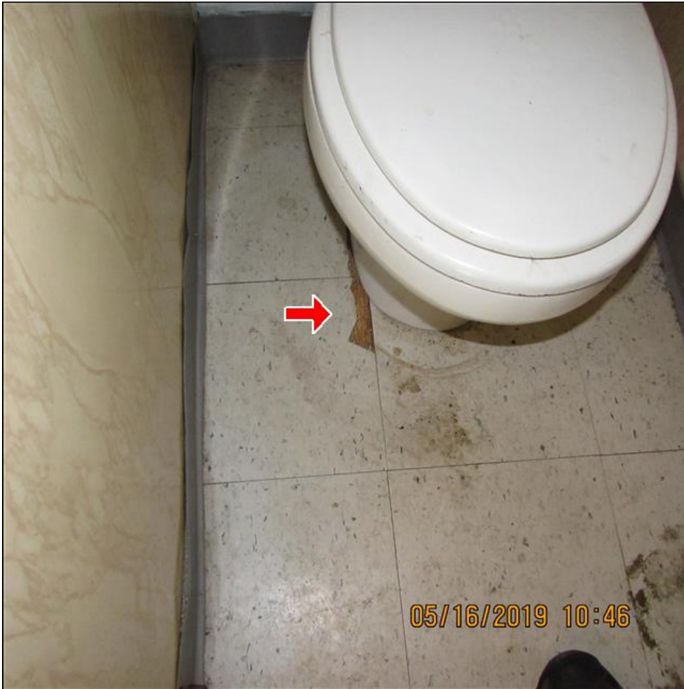
4.2 Item 3(Picture) 2nd floor bathroom
