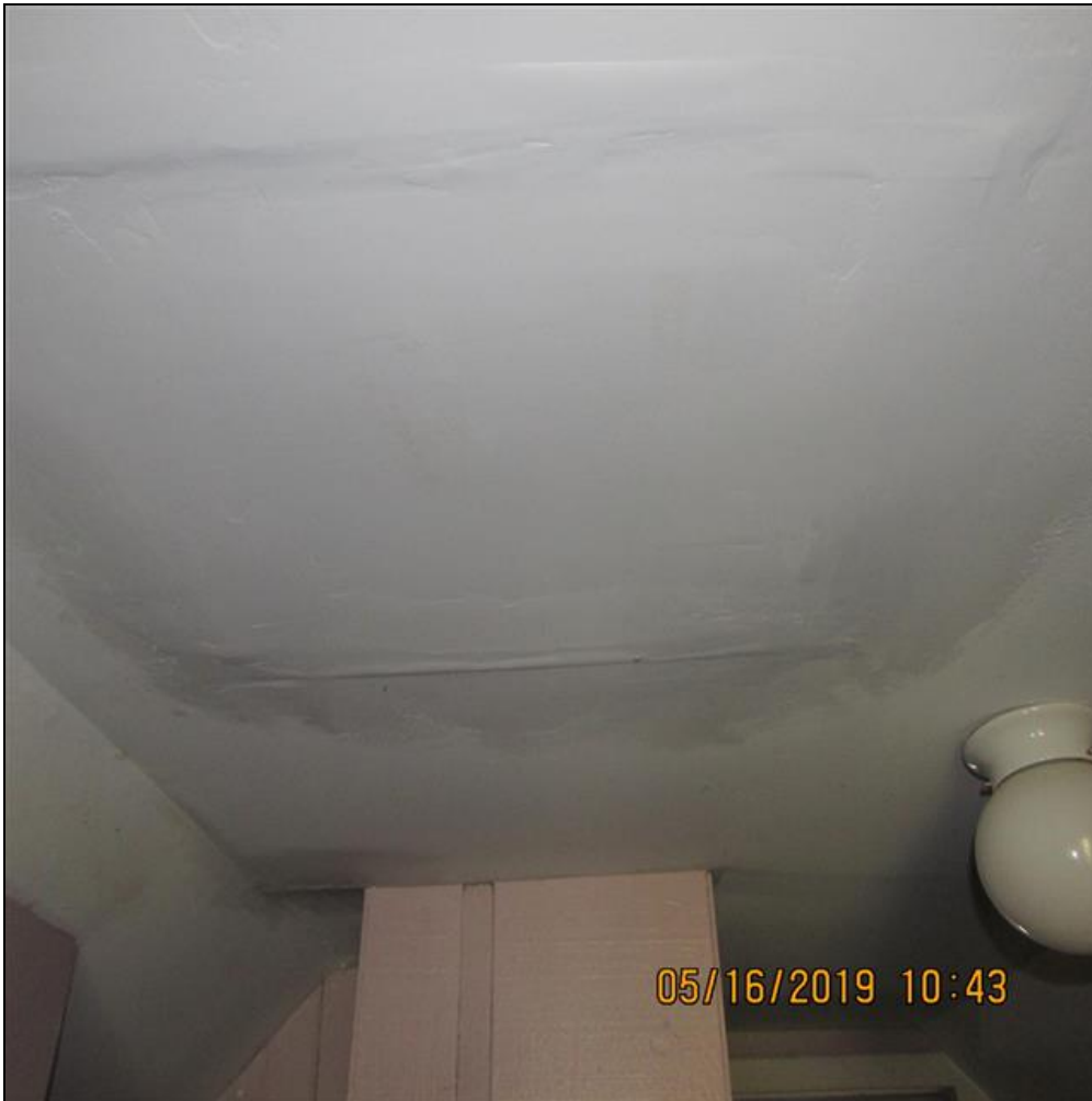
4.0 Item 1(Picture) 2nd floor ceiling repair
