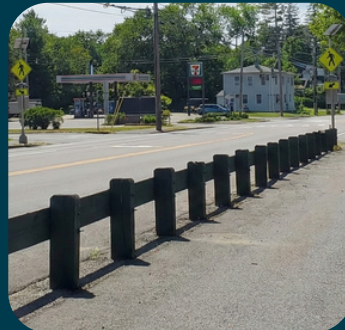
IMPROVED ACCESS TO CITY PARKS AND TRAILS ON RIVERSIDE STREET
