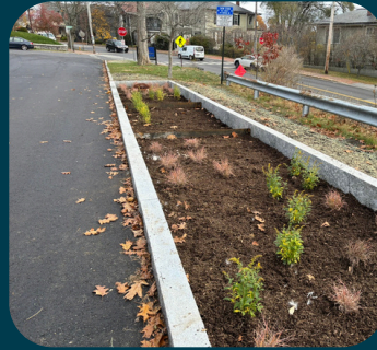
GREEN INFRASTRUCTURE INSTALLED ON THE WESTERN PROM
