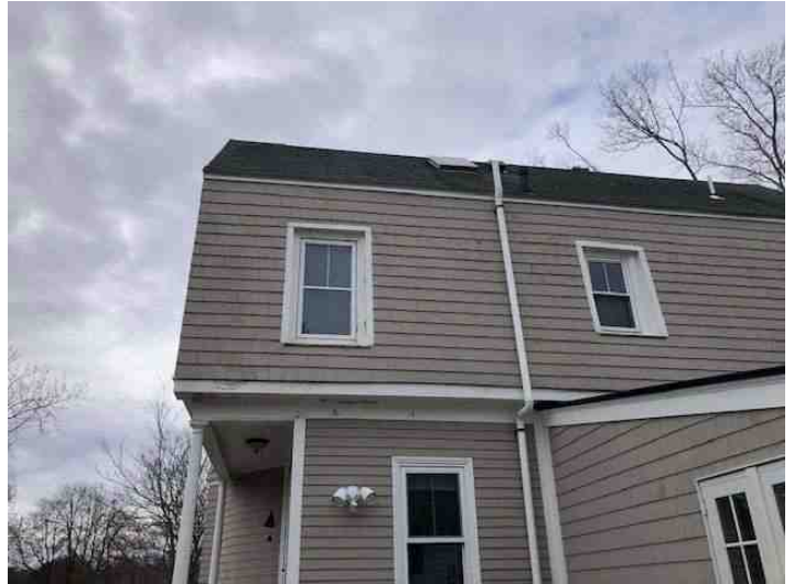
Rear - Second Floor
