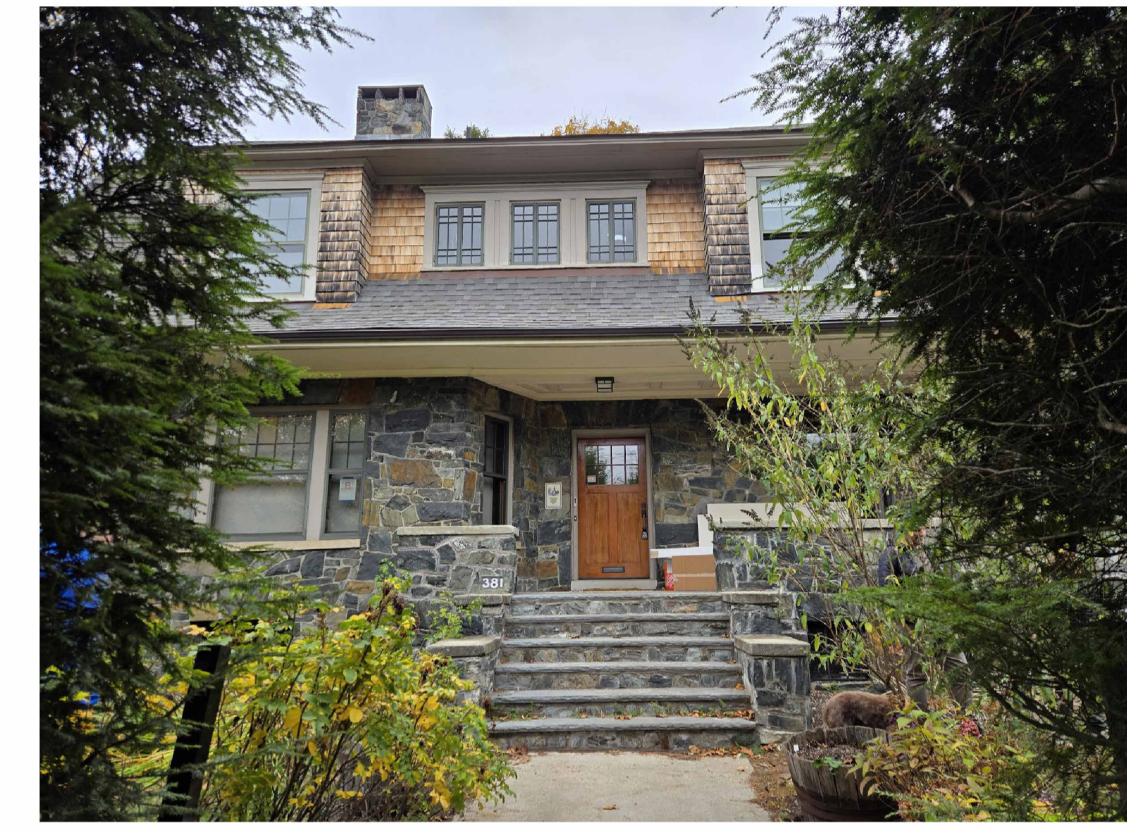
DANFORTH STREET - MAIN ENTRY WALKWAY
