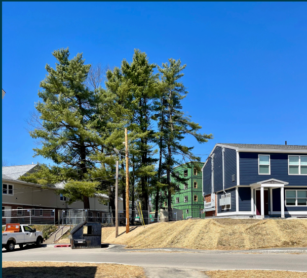
Riverton Park (approved 2023) Renovation of 21 existing townhouses and construction of a new building with 64 dwelling units.
